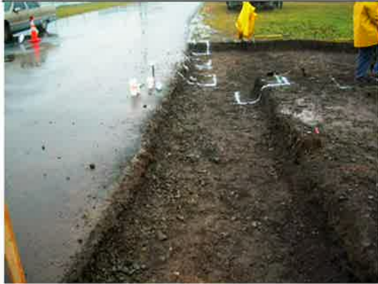
Picture 1: Sidewalk excavation and bollard layout
