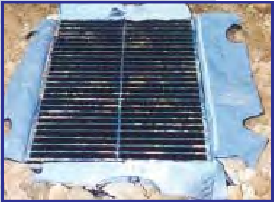
installed Siltsack held in place by grate.
