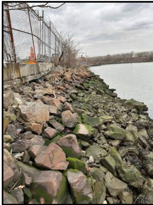
Photo 4: Stone riprap adjacent to fence/gate opening.
