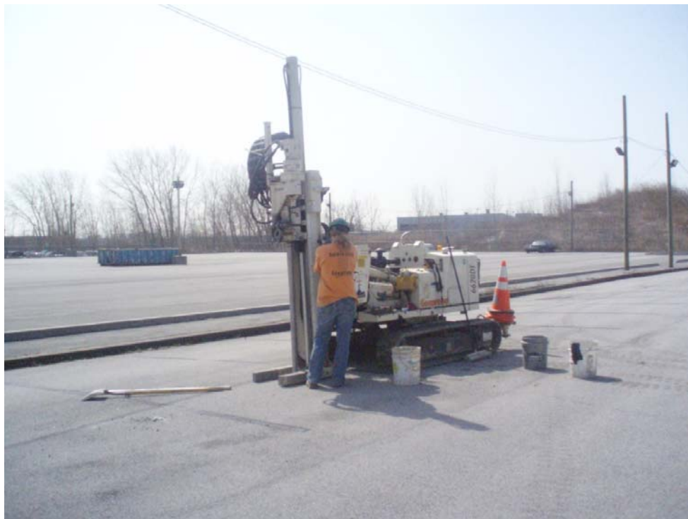
Photograph 4: Drilling Boring B18.
