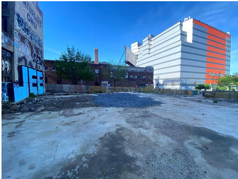
Photo 2: View of site prior to mobilization for excavation activities, facing south. Taken on 05/07/2021
