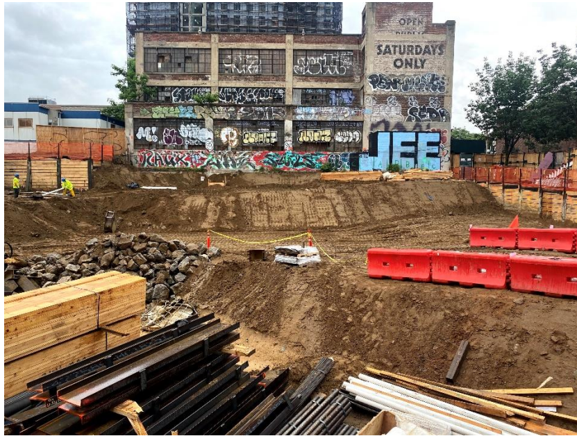
Photo 9: View of excavation progress, facing east. Taken on 06/1/2021
