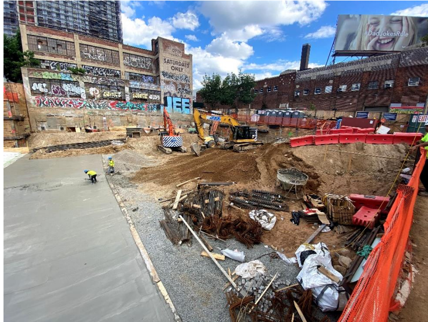
Photo 13: General view of site progress, facing southeast. Taken on 08/02/2021
