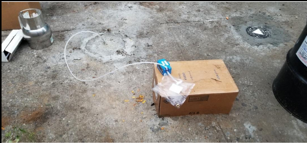
Photograph 2 - Purging vapors prior to sampling at temporary soil vapor point RI-SV-03.
