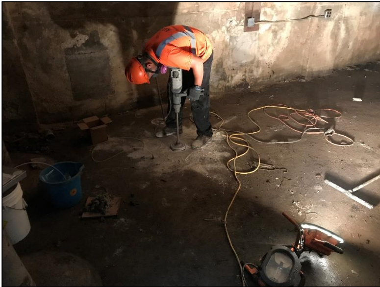
Photograph 1: Coring through the Site building concrete basement slab to facilitate installation of temporary soil vapor point RI-SV-04.
