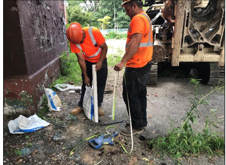
Photograph 3: Installation of groundwater monitoring well RI-MW-05.
