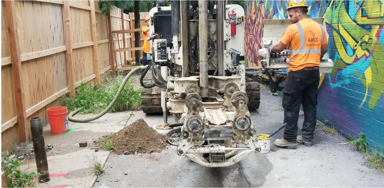
Installation of monitoring well RI-MW-03 in the Westchester Avenue sidewalk.
