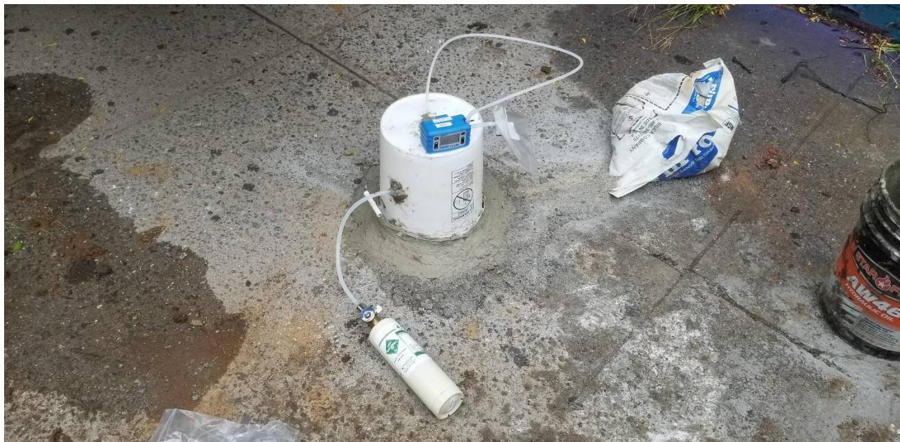
Purging vapors at temporary soil vapor point RI-SV-03.
