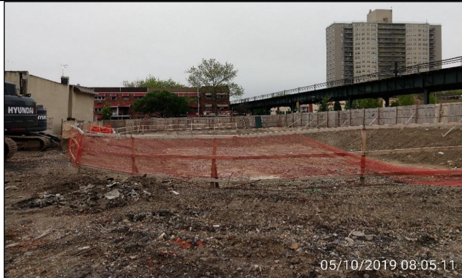
Photograph 1 - View of the southern portion of the Site, facing east.
