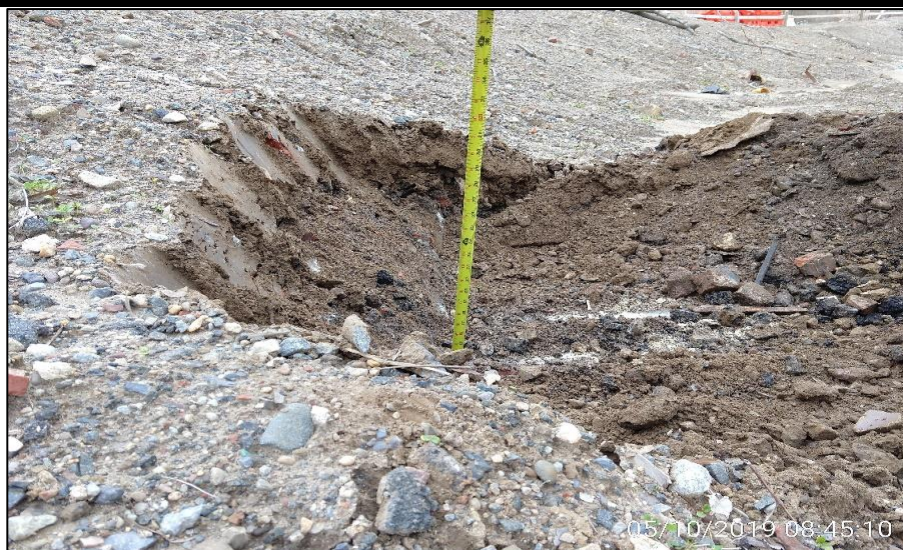
Photograph 3 - Test pit excavation in disposal grid WC-14 to facilitate waste classification sample collection.
