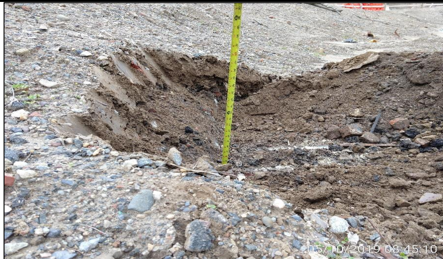
Photograph 3 - Test pit excavation in disposal grid WC-14 to facilitate waste classification sample collection.
