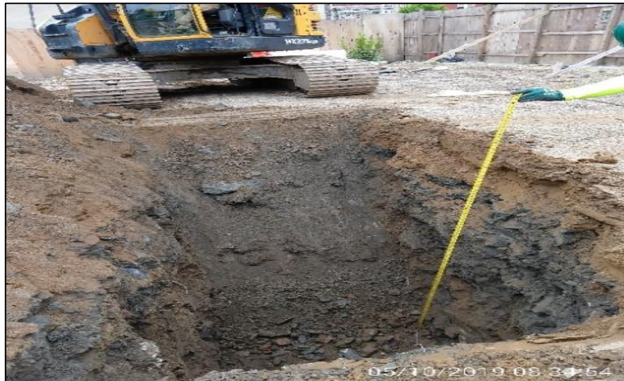
Photograph 2 - Test pit excavation in disposal grid WC-13 to facilitate waste classification sample collection.
