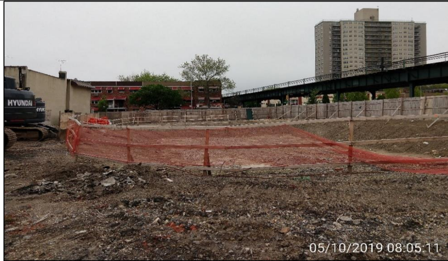
Photograph 1 - View of the southern portion of the Site, facing east.
