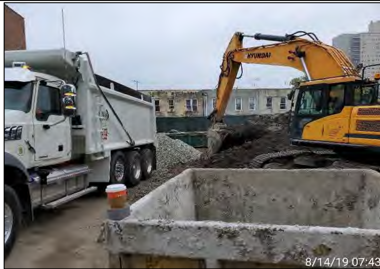
Photograph 2 - Off-site disposal of soil/fill from grid WC-07, facing east.
