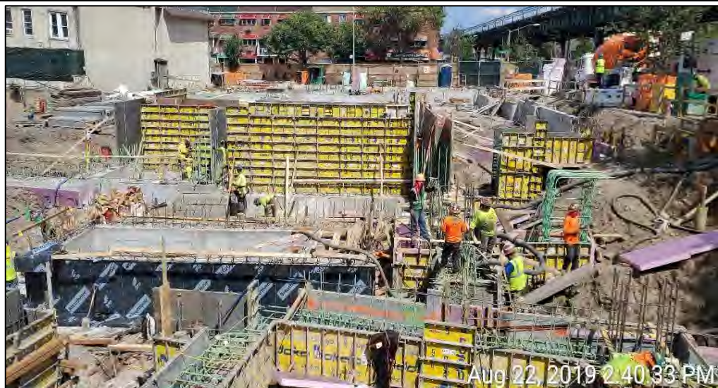
Photograph 3 - Foundation work in grid C3, facing east.
