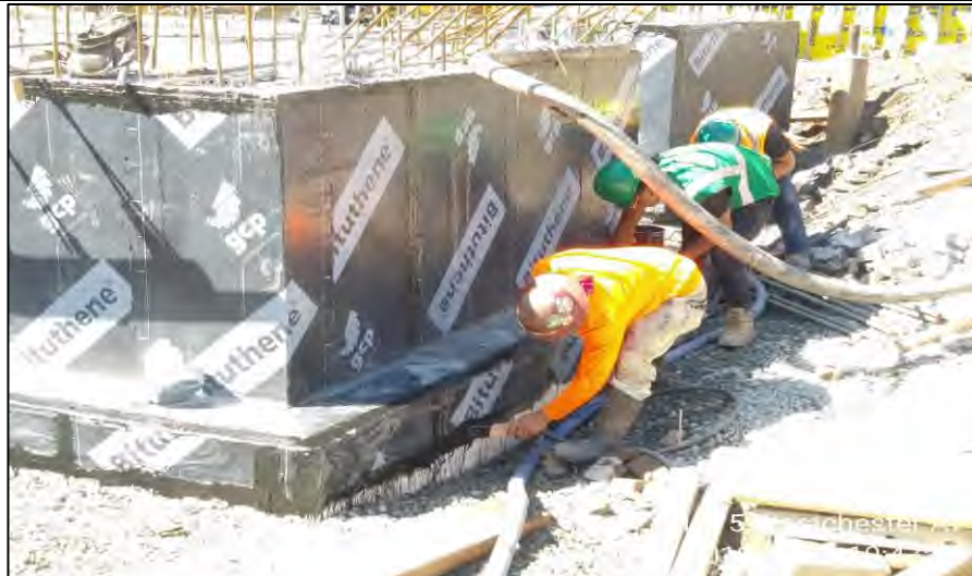
Photograph 2 - GCP Bituthene 4000 and Bituthene liquid mastic installation in grid C3.
