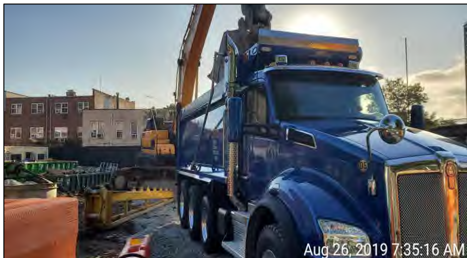
Photograph 3 - Off-site disposal of excavated soil/fill in Grid A3, facing east.
