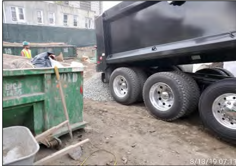
Photograph 1 - Squarried stone import in grid A2, facing southeast.
