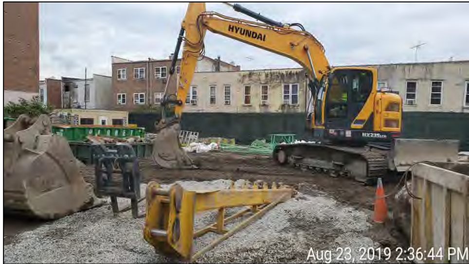
Photograph 1 - Grading soil/fill in grid A2, facing northeast.
