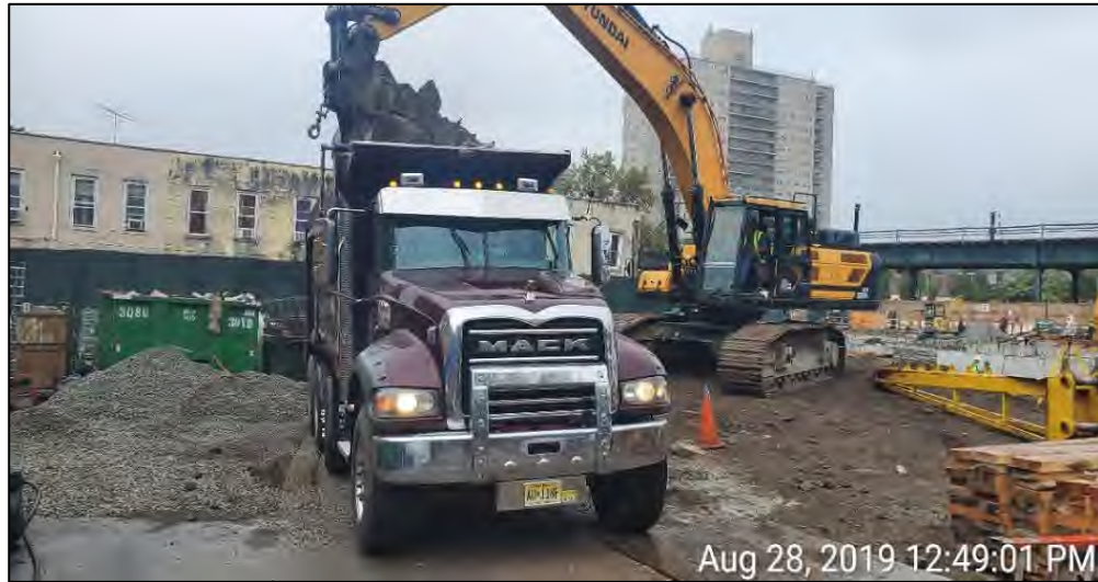
Photograph 1 - Off-site disposal of soil/fill to the SSI Metro 12 facility in Carteret, New Jersey in grid A3, facing east.
