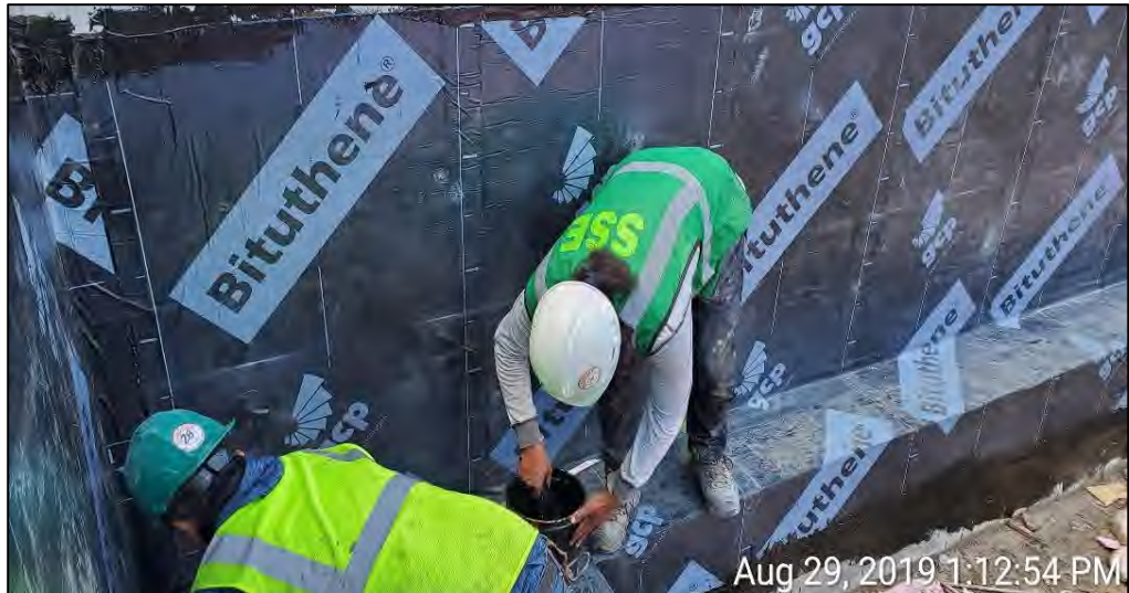
Photograph 2 - GCP Bituthene 4000 waterproofing membrane installation in grids B2 and C2.
