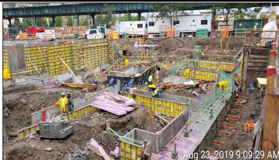
Photograph 3 - Foundation work in grid C3, facing south.
