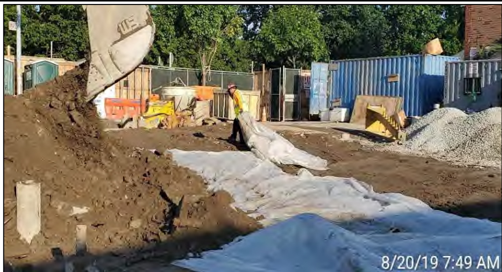
Photograph 3 - Staging excavated soil/fill on polyethylene sheeting in grid A3, facing northwest.
