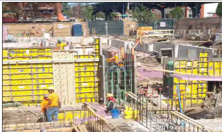
Photograph 3 - Rebar and concrete form installation in grid C3, facing east.
