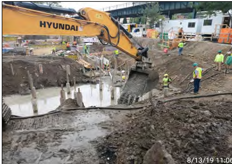
Photograph 2 - Quarried stone installation at sump pit in grids B3 and C3, facing southeast.
