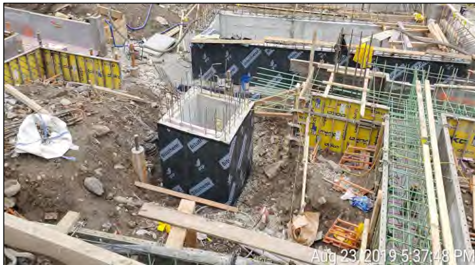
Photograph 2 - GCP Bituthene 4000 and liquid mastic installed in grid C3, facing east.
