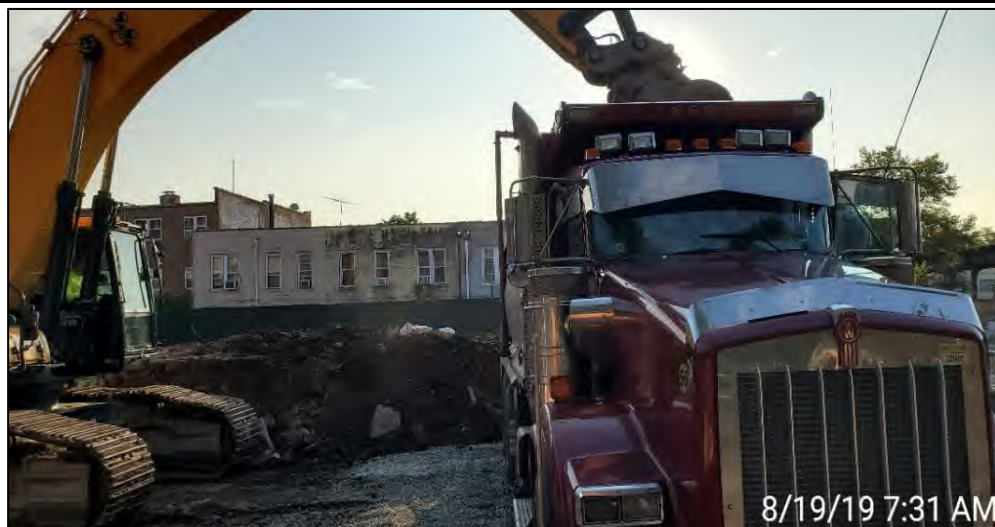
Photograph 3 - Loading trucks for off-site disposal of soil/fill to SSI Metro 12 in Carteret, New Jersey.
