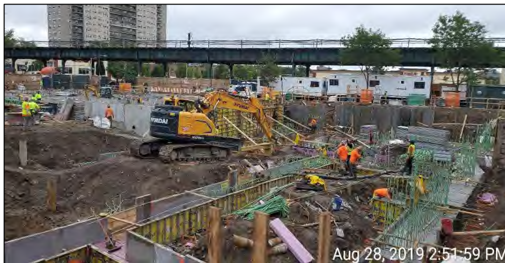
Photograph 3 - Foundation work in grids B3, C3, C2, facing south.
