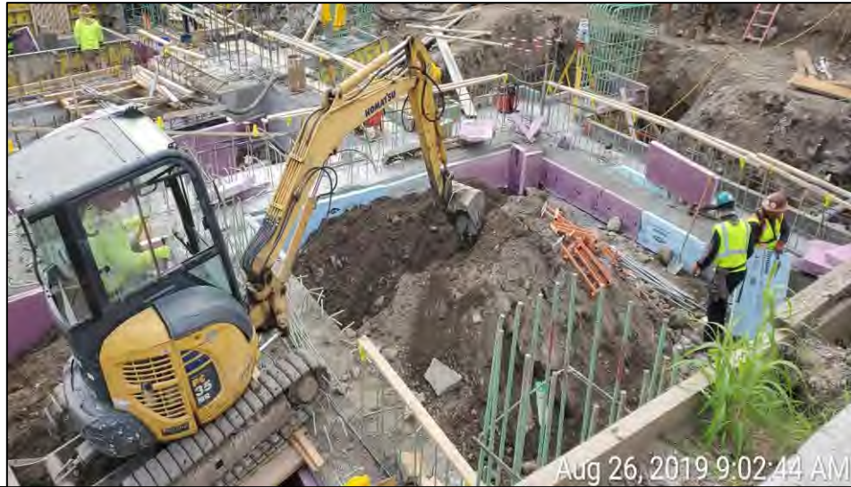
Photograph 1 - Grading soil/fill in grid C3.
