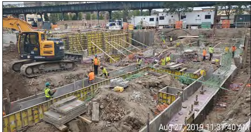
Photograph 2 - Foundation work in grids B3, C3, C2, facing south.
