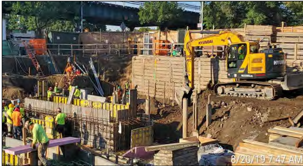
Photograph 1 - Excavation in grid C3, facing southwest.
