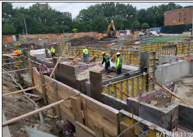
Photograph 3 - Rebar and form work in grid C2, facing northwest.
