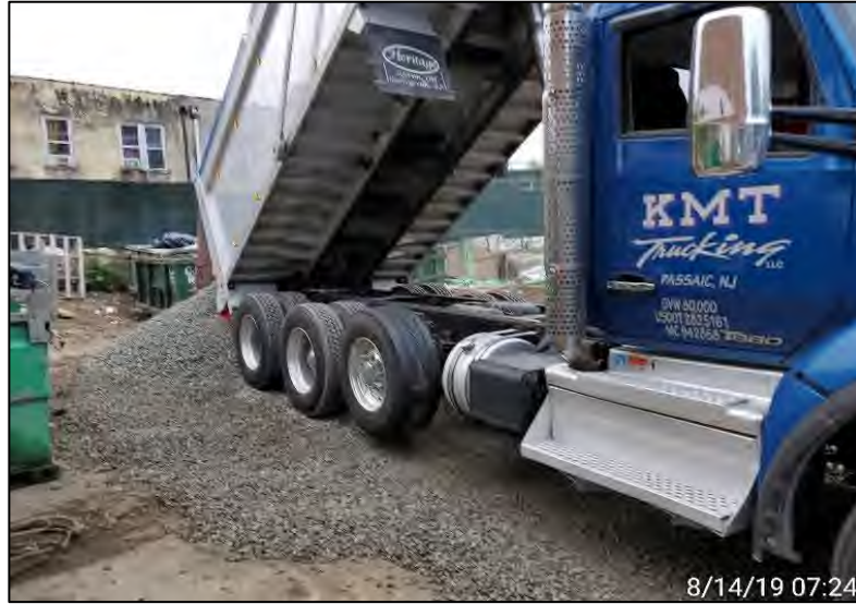
Photograph 1 - Quarried stone import in grid A2, facing east.
