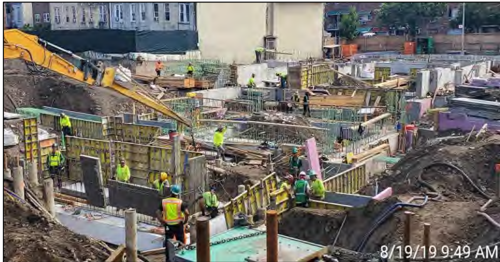
Photograph 1 - Foundation element installation in grid C3 facing northeast.
