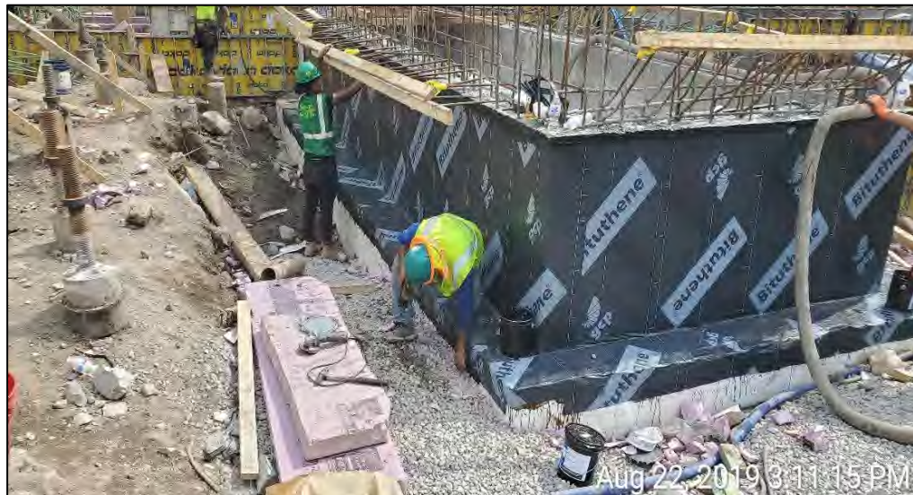
Photograph 2 - GCP Bituthene 4000 and Bituthene liquid mastic installation on the exterior elevator pit wall in grid C3.
