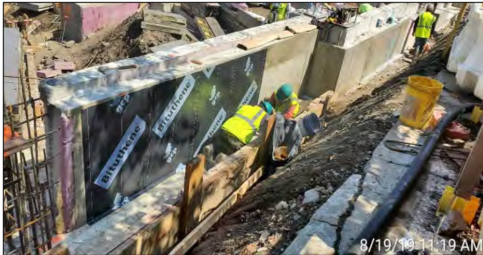
Photograph 2 - GCP Bituthene 4000 installation in grid C2, facing.
