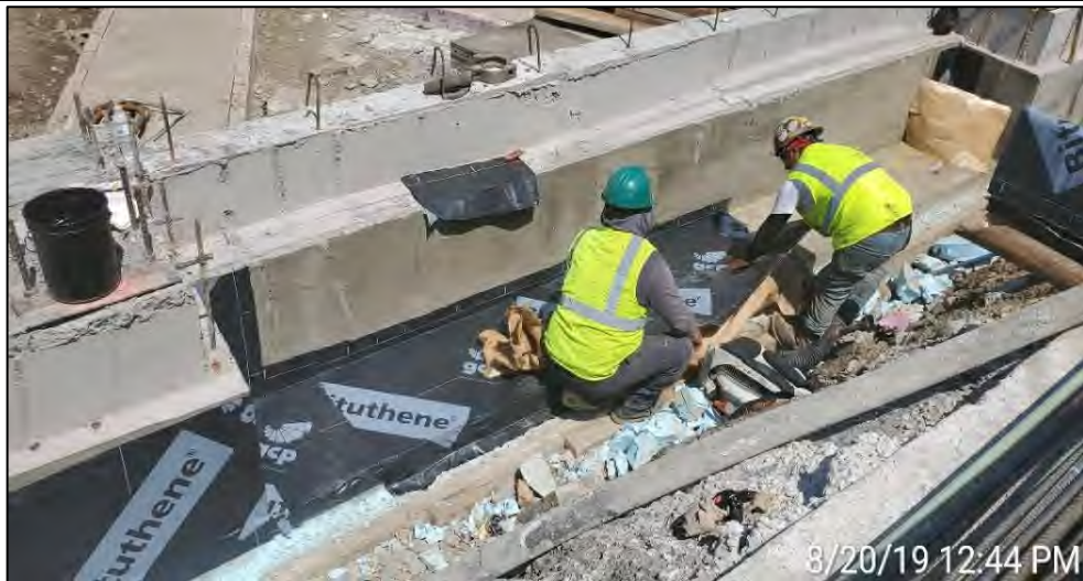
Photograph 2 - GCP GCP Bituthene 4000 waterproofing membrane installation in grid C2.
