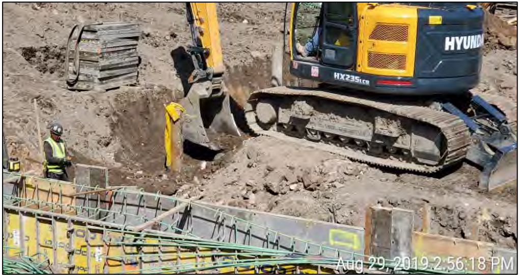
Photograph 1 - Minor excavation of soil/fill in grids A3 and A2, facing north.
