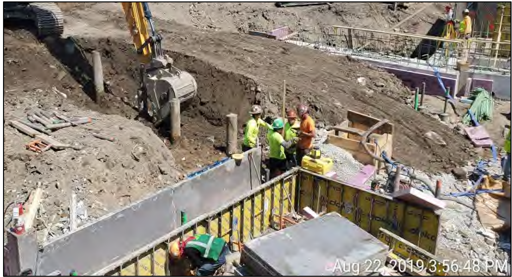
Photograph 1 - Soil/fill excavation in grid B3, facing northeast.
