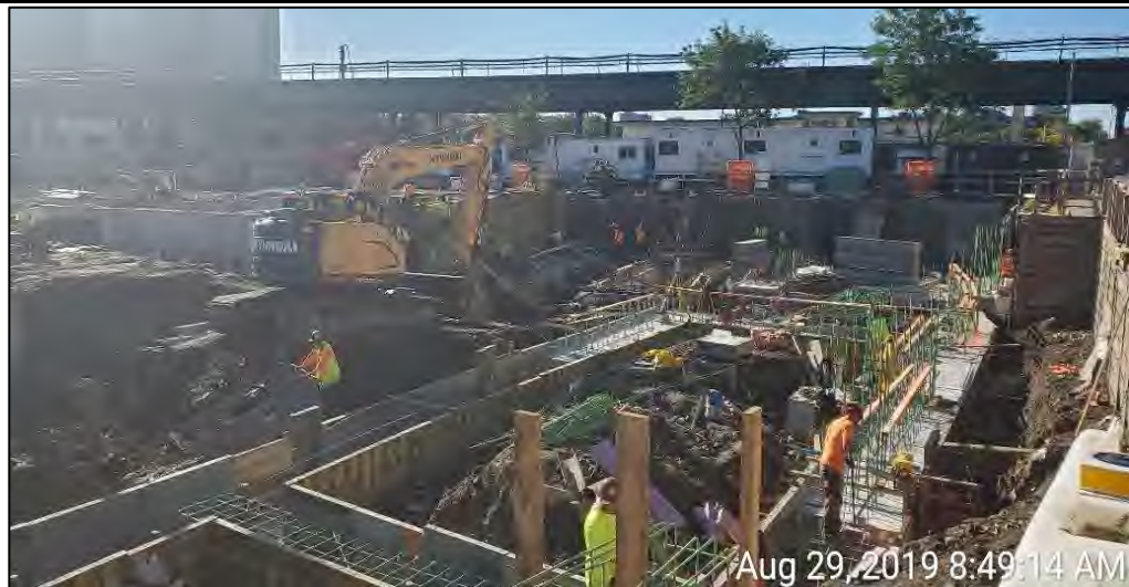
Photograph 3 - Foundation work in grids B3, C3, B2, C2, facing south.
