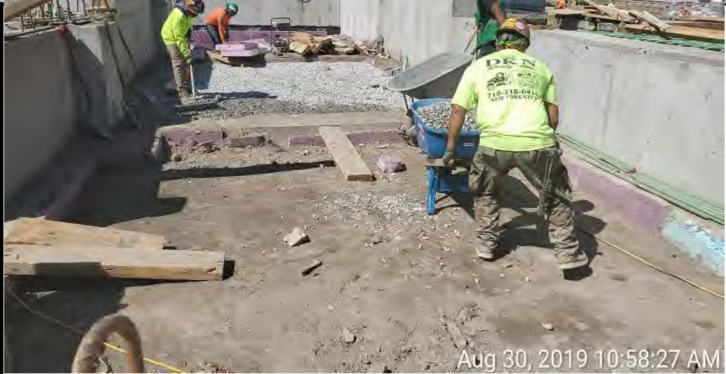
Photograph 1 - Placing imported stones on soil/fill in grid B2, facing west.
