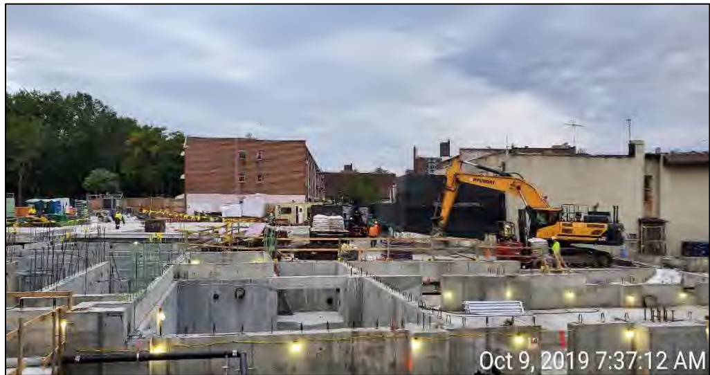
Photograph 1 - View of the site facing north.
