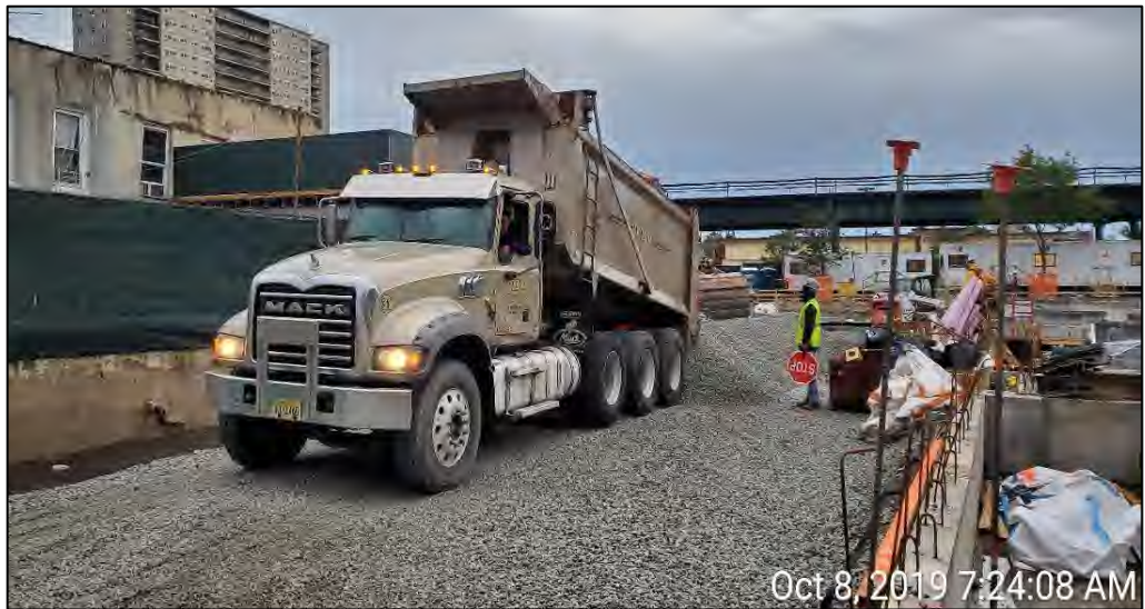
Photograph 1 - Importing quarried stone from Hamburg Quarry in Hamburg, New Jersey at grid A2, facing south.
