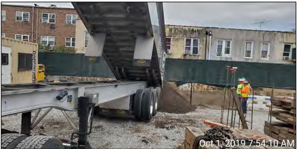
Photograph 3 - Delivering in grid A2, view facing east.
