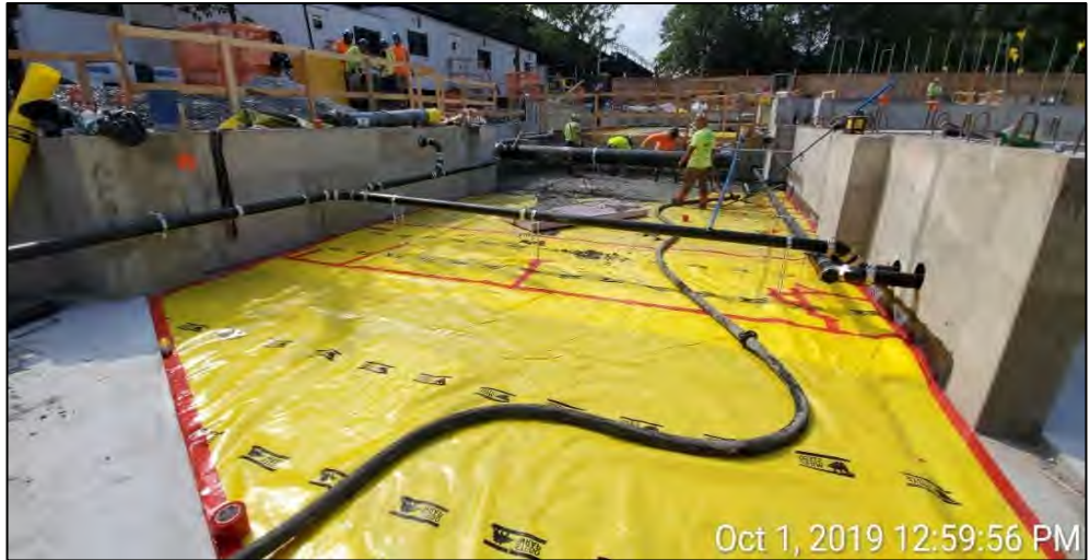
Photograph 1 - Vapor barrier installation in Grid C2, view facing west.
