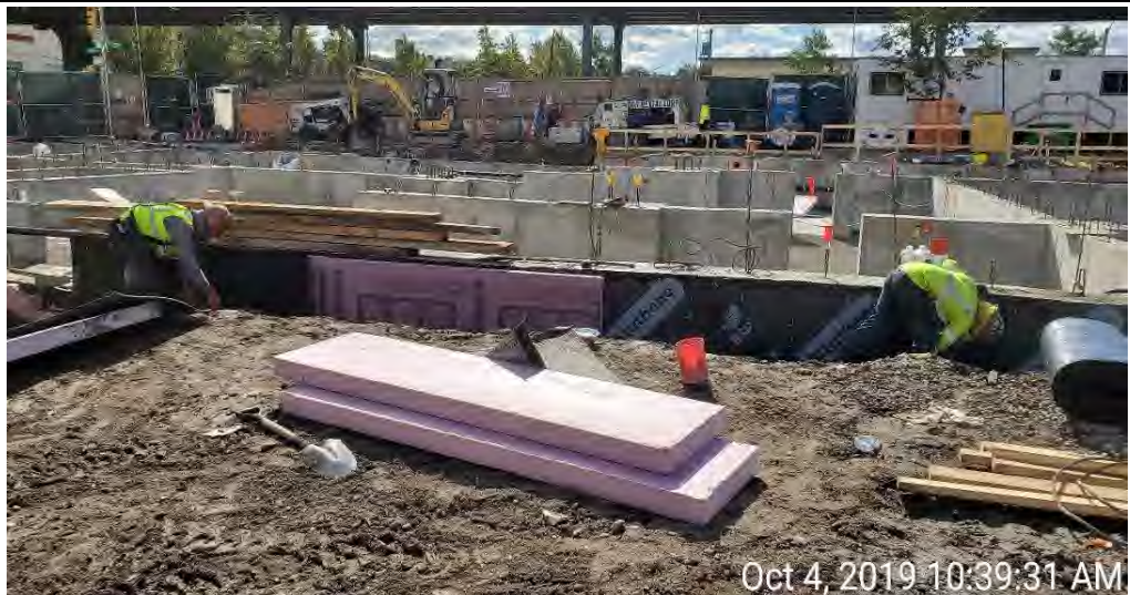
Photograph 2 - Waterproofing in grid B2, facing south.
