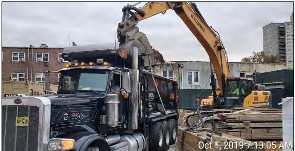
Photograph 2 - Loading trucks for off-site disposal of soil/fill from grid WC-09 (Grid A2), view facing east.
