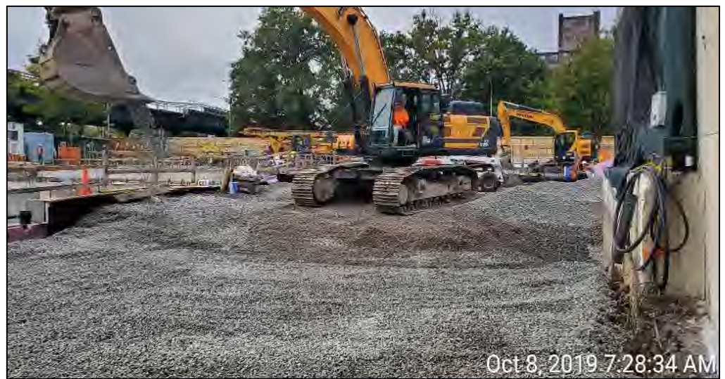
Photograph 3 - Imported quarried stone from Hamburg Quarry in Hamburg, New Jersey placed on grid B2, facing southwest.
