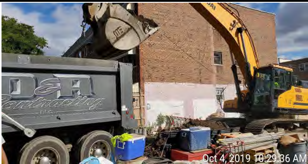
Photograph 3 - Soil/fill trucking in grid A3, facing north.
