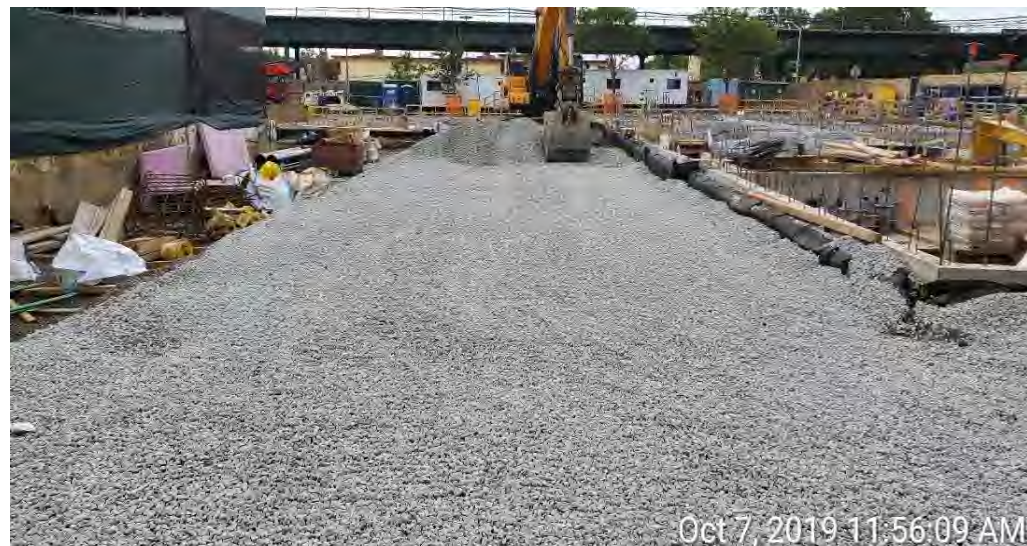
Photograph 2 - Imported quarried stone from Hamburg Quarry in Hamburg, New Jersey placed on grid A2, facing south.
