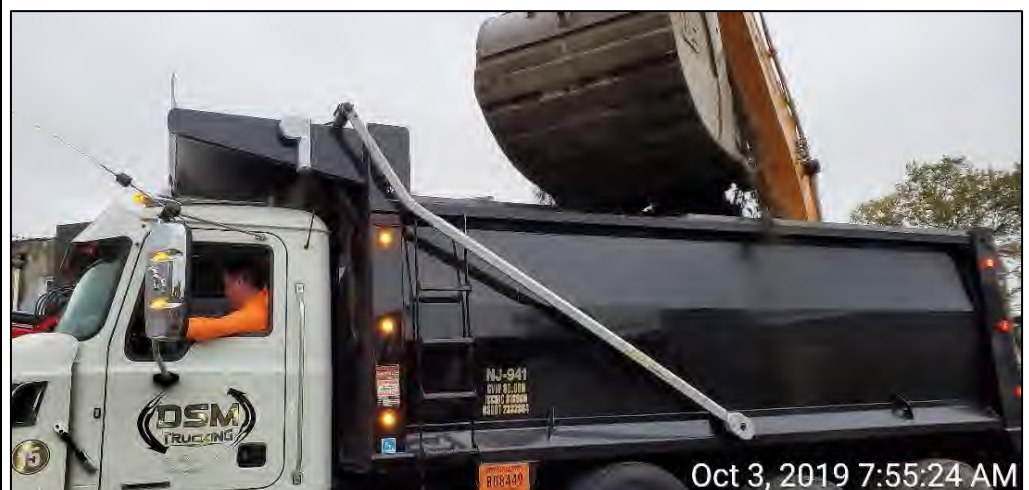
Photograph 3 - Soil/fill trucking in grid A2, facing east.
