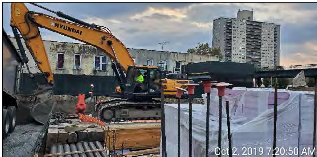
Photograph 2 - Stone delivery in grid WC-09 (Grid A2), view facing east.
