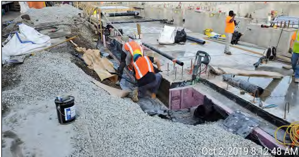
Photograph 1 - Waterproofing installation in grid C2, facing west.
