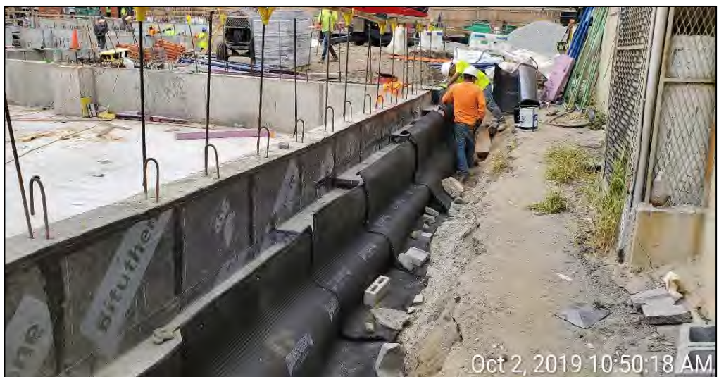
Photograph 3 - Waterproofing installation in grid B1, facing north.
