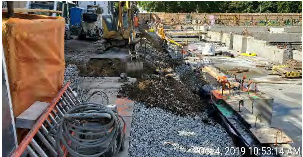
Photograph 1 - Trenching for piping outside the site perimeter in grid C3, facing west.
