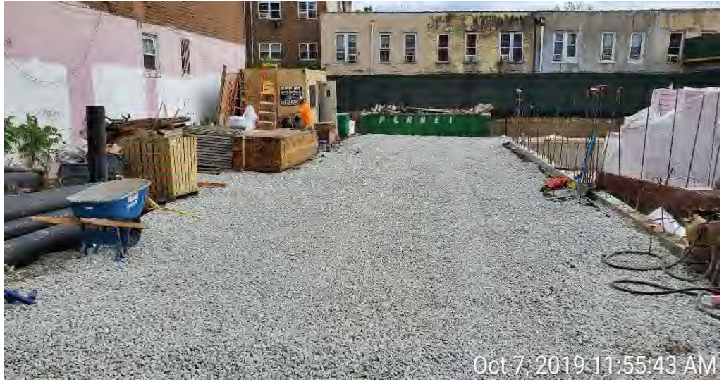
Photograph 1 - Imported quarried stone from Hamburg Quarry in Hamburg, New Jersey placed on grids A3 and A2, facing east.
