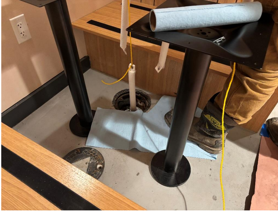
Photo 1: ORC sock deployment in RMW14
