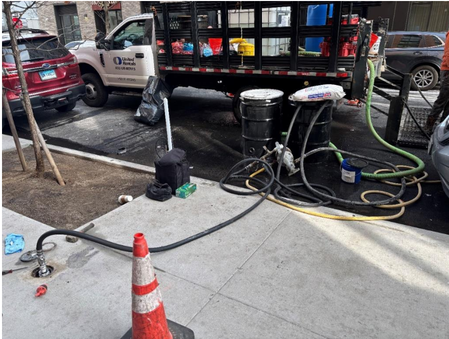
Photo 1: View of Coastal injecting PetroFix into off-site monitoring well OMW-02.
