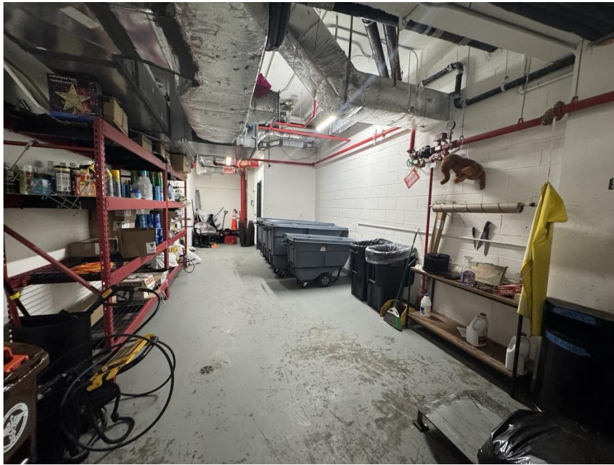
Photo 7: General view of surface cover in the building cellar
