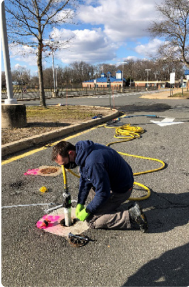
Figure 6 - Client performing a well flush.
