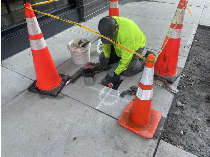
Photo 1: AARCO installing a flush-mounted road box and concrete pad at OMW-01.
