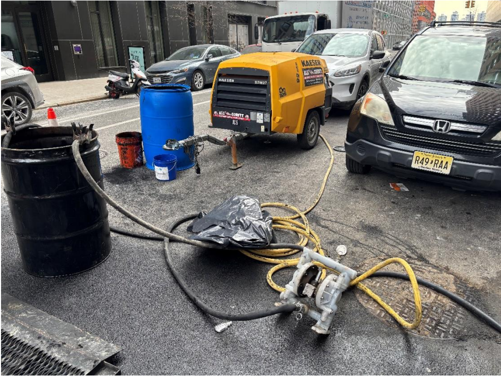
Photo 2: Injection system set up prior for injections in OMW-02
