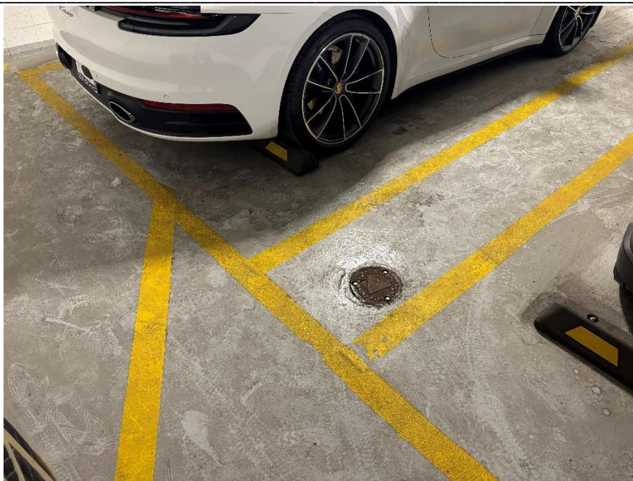
Photo 9: View of post-remediation groundwater monitoring well RMW03
