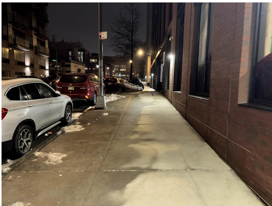
Photo 2: View of the sidewalk along the western part of the site.
