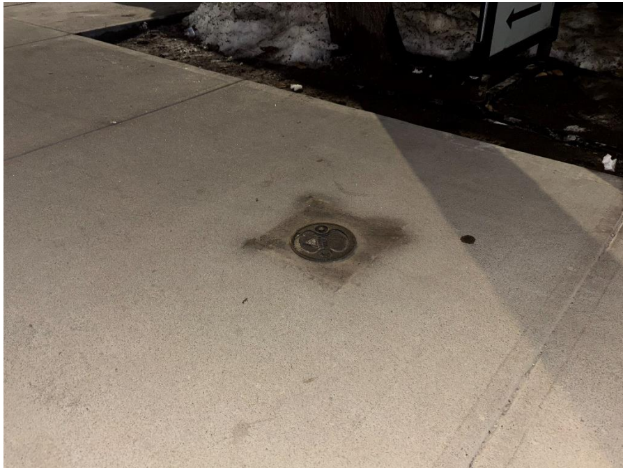
Photo 8: View of off-site groundwater monitoring well OMW-01
