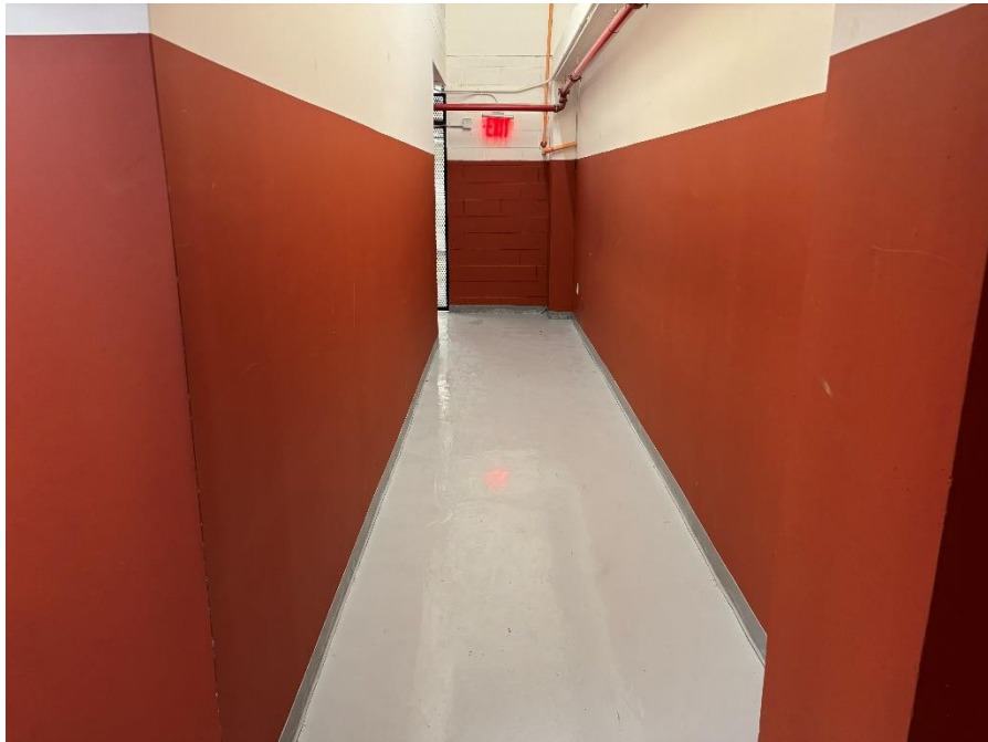
Photo 6: General view of surface cover in the building cellar
