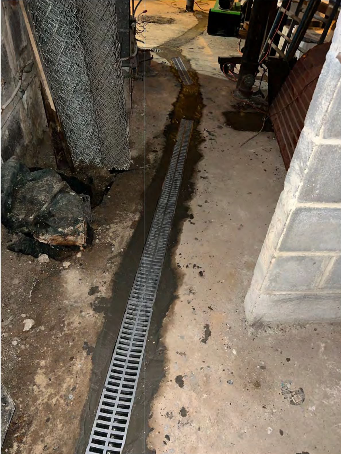
Newly installed drains following installation
