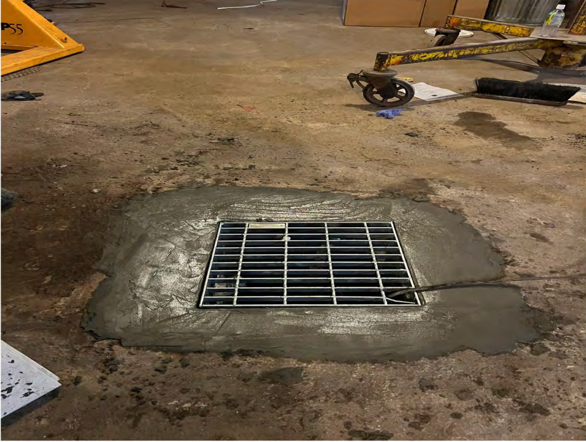
Newly installed catch basin following installation
