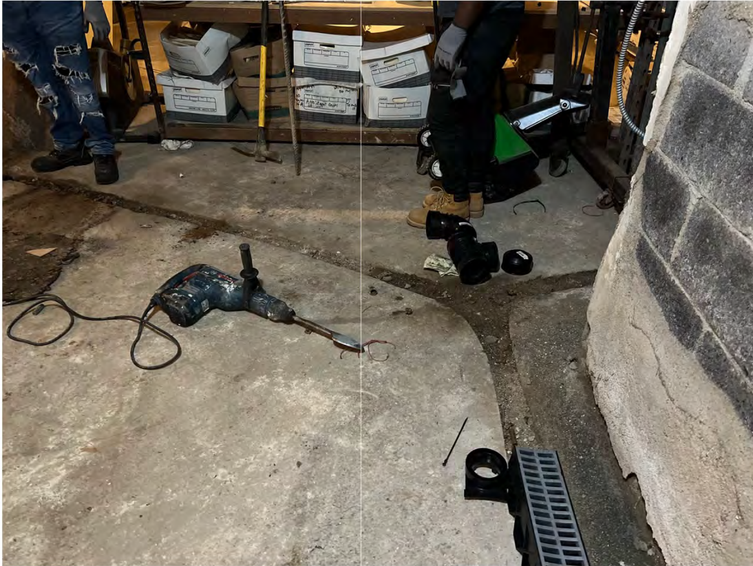
Existing exposed trenches to be sealed during IRM
