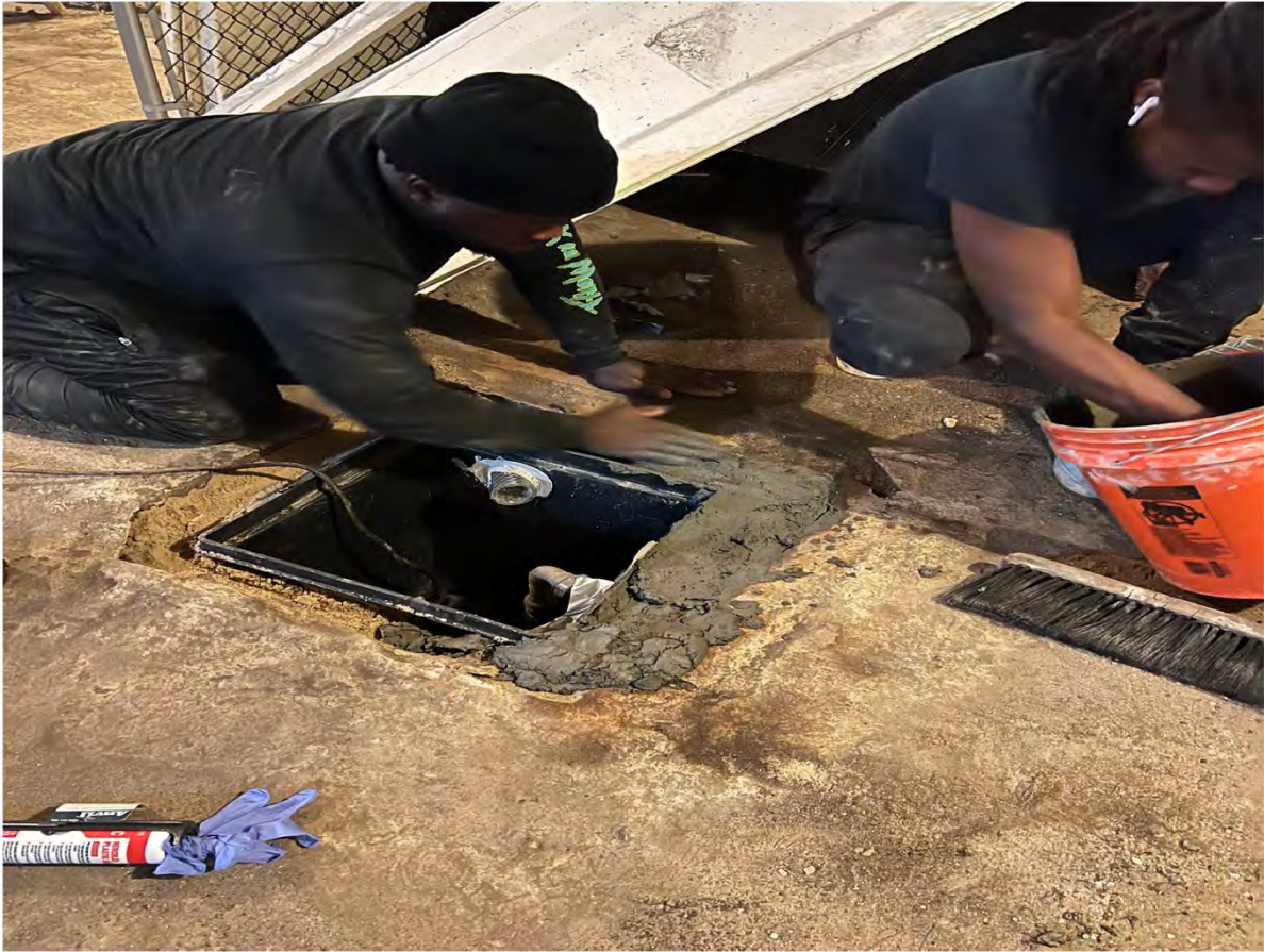
Installed Catch basins to replaced brick exposed sumps
