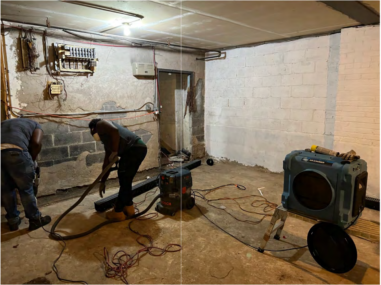
Bosch HEPA Dust Collector to collect dust during concrete trench work
