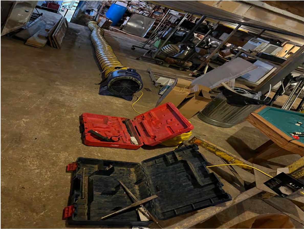
Ventilation Fan during ground intrusive work
