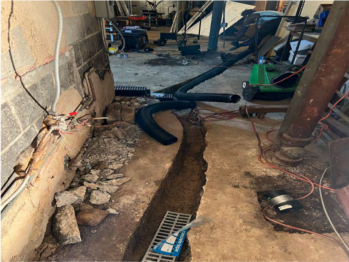
Expanded Trenches with Sealed drains and subsurface piping to be installed
