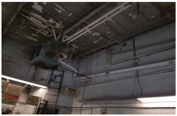
View of electric/natural gas-fired space heater within Karz Auto Collision, which is typical of other Site buildings, and potential ACBM-containing pipe insulation.
