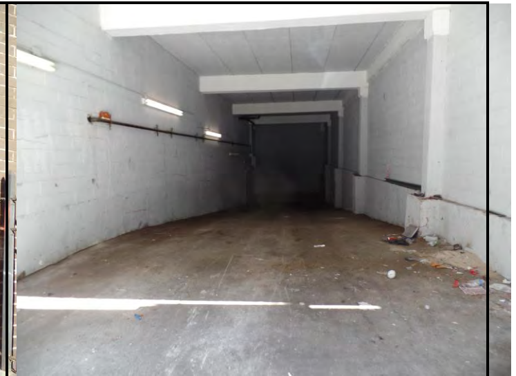
Eastern Portion of Garage
