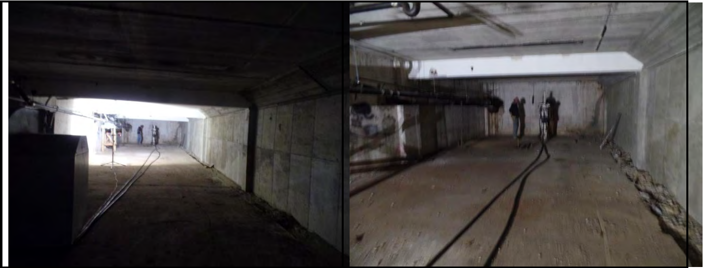
Installation of SB-1 / MW-1
