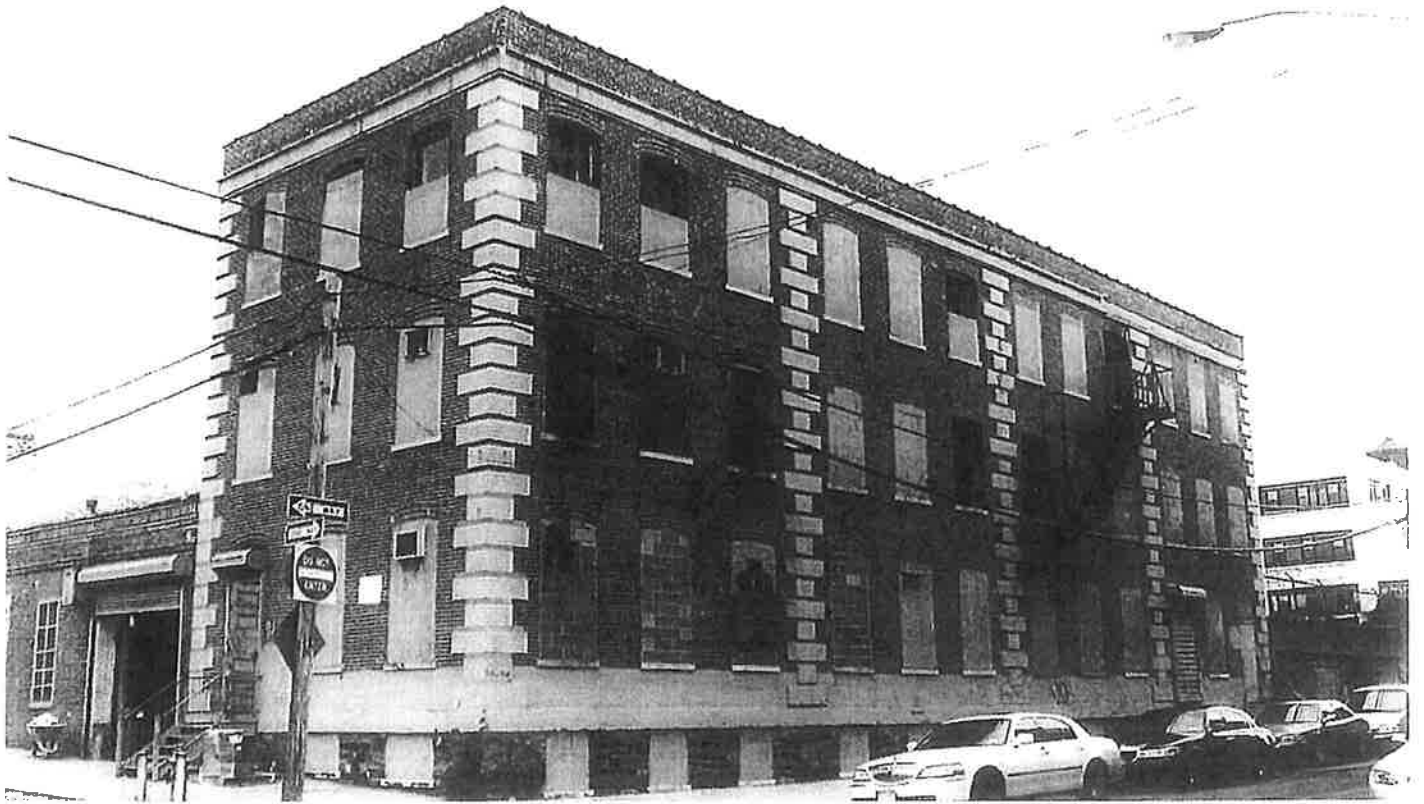
SE corner of property; view facing NW
