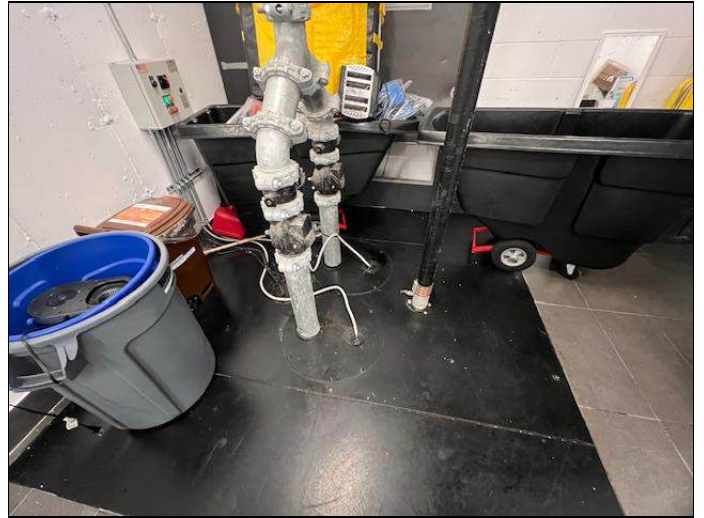
8. Sump Pump in Basement
