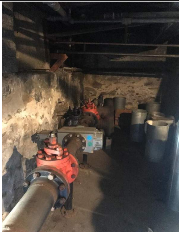
Photo 18: Incoming natural gas connections in the crawl space.
