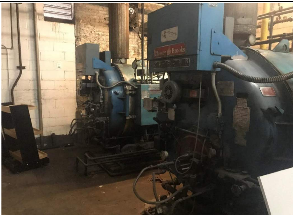
Photo 12: Two natural gas fired boilers located on the ground level.
