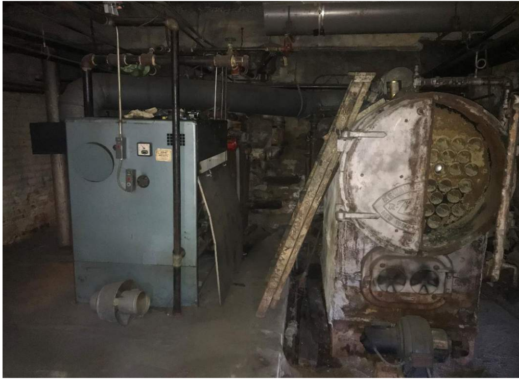
Photo 19: One natural gas fired boiler and one decommissioned boiler in the crawl space.
