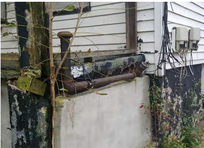
Vent & fill at 720 East 216th Street – rear building
