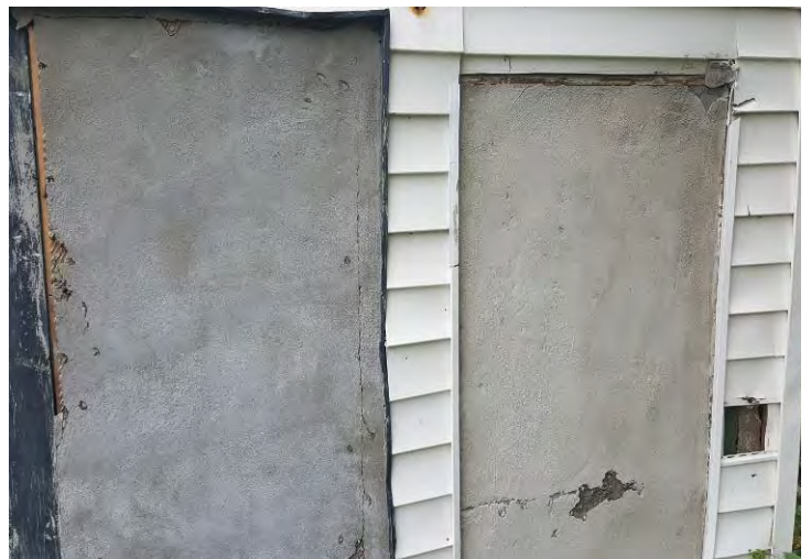
Sealed first floor door
