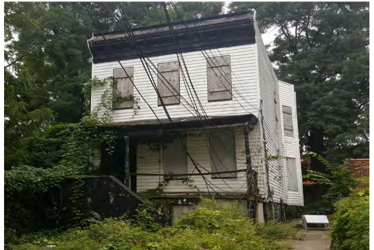
720 East 216th Street – rear building
