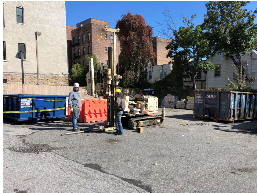
Installing Soil Probe
