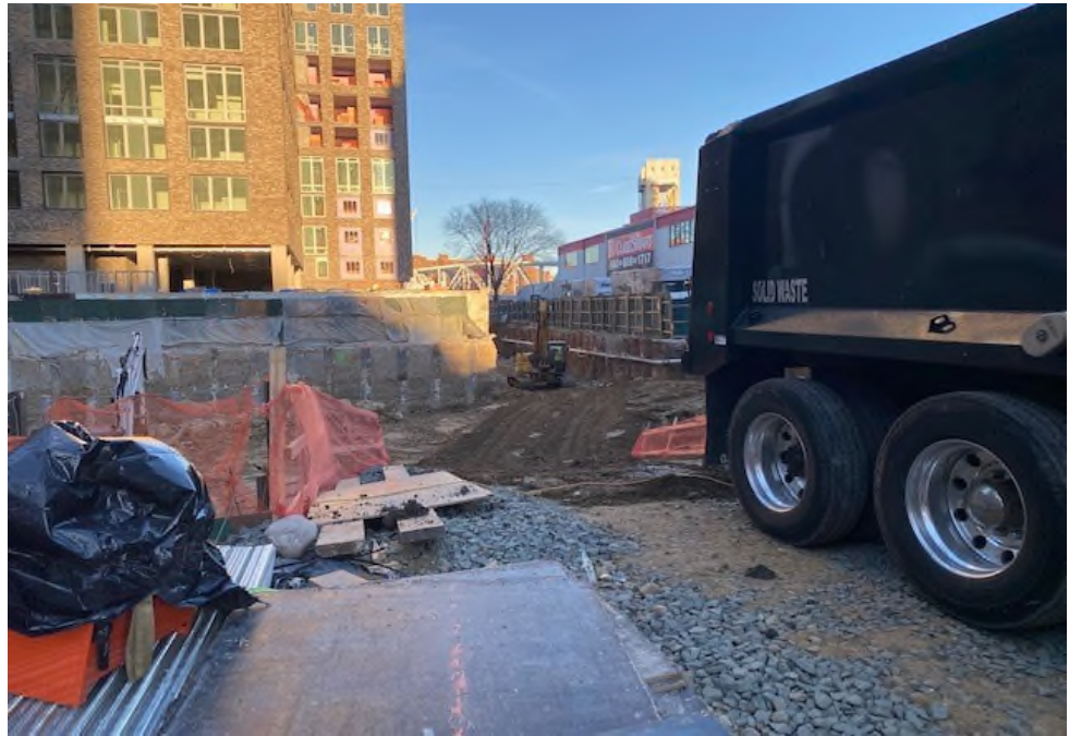
Photograph 1 - Loading out truck for soil export, view facing north
