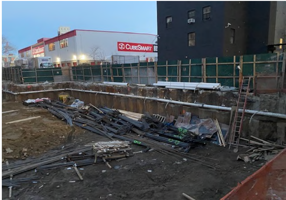
Photograph 1 - Staged rebar in Grid A3, view facing north
