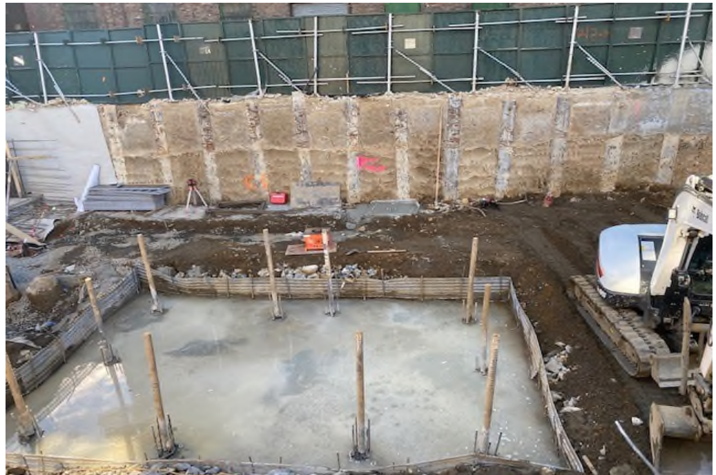
Photograph 2 - Installed waterproofing (background) and pile cap work (foreground), view facing west.
