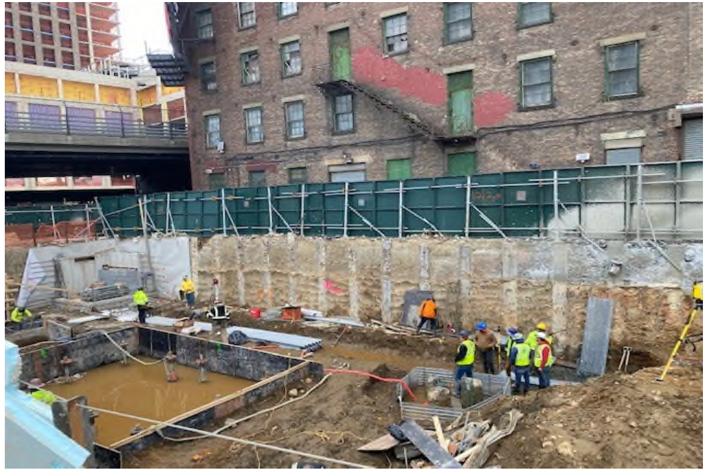
Photograph 1 - Installing waterproofing (background) and pile cap work (foreground), view facing southwest
