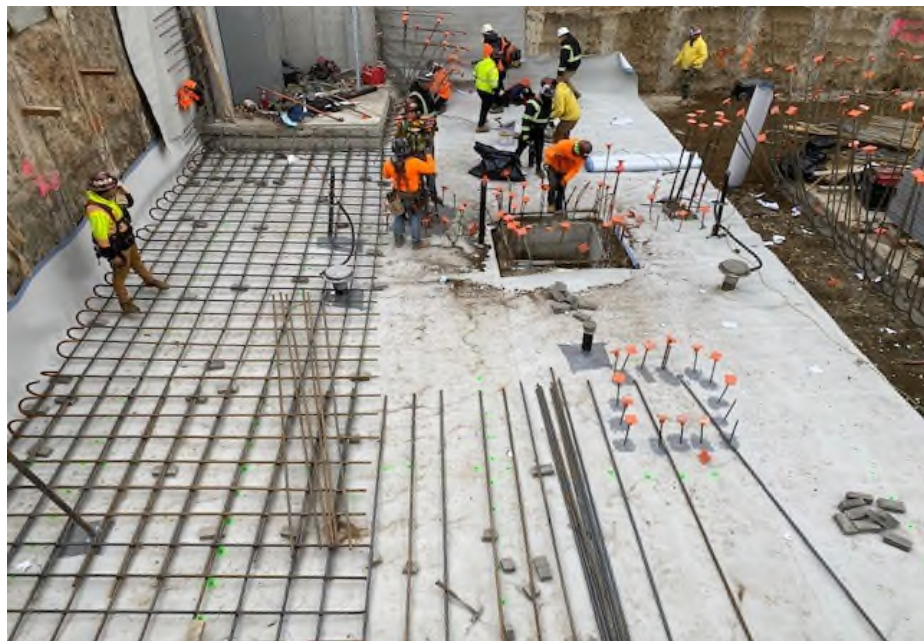
Photograph 2 - Installing waterproofing/vapor barrier membrane in Grid B4, view facing west.
