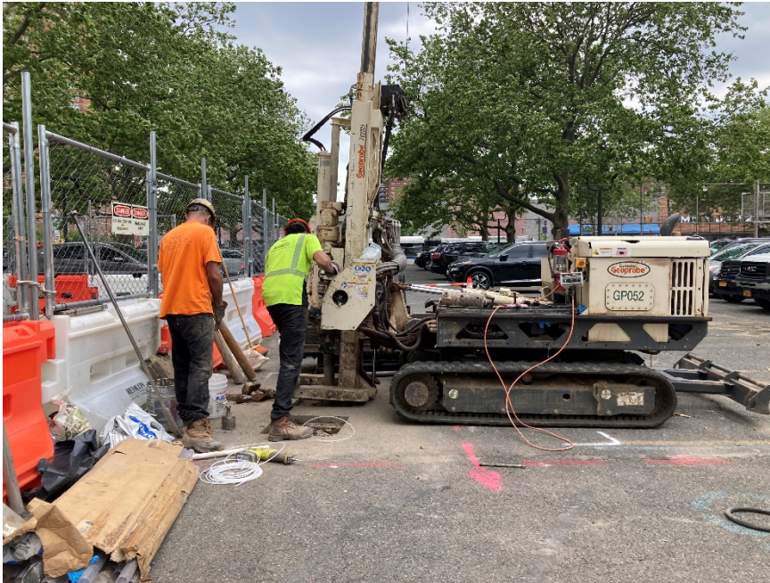
Photo 3: Looking west, view of AARCO drilling RXSB-2/MW-2/SV-2 using hand tools and vacuum/air-knife.
