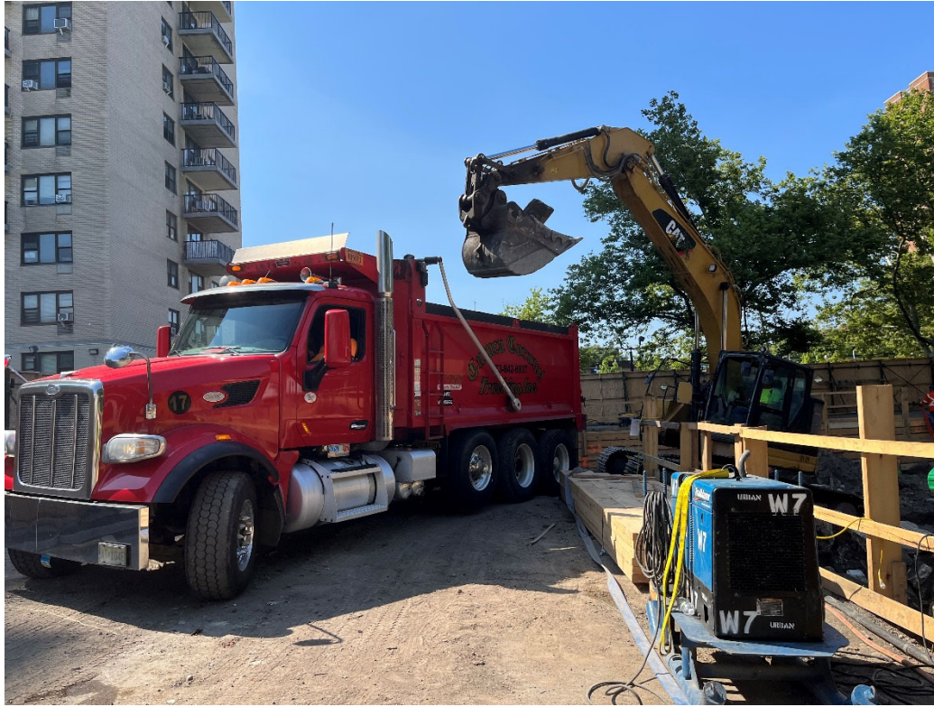
Photo 1: Looking south, Urban loads Cuenca Coronel truck #17 with rock for offsite disposal.
