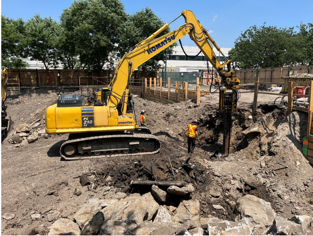
Photo 1: Looking north, Urban drives I-beam along eastern edge of excavation.
