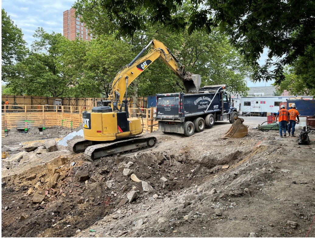
Photo 1: Looking southwest, Cuenca Munoz truck #14 is loaded with non-hazardous soil.
