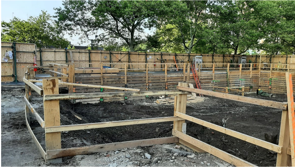
Photo 2: View facing SSW, conditions of the Site late morning.
