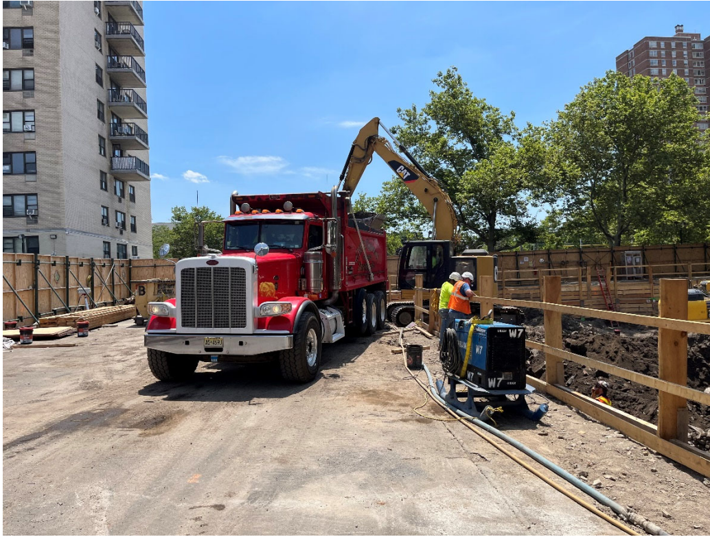
Photo 1: Looking south, Cuenca Coronel truck #65 is loaded with non-hazardous soil.
