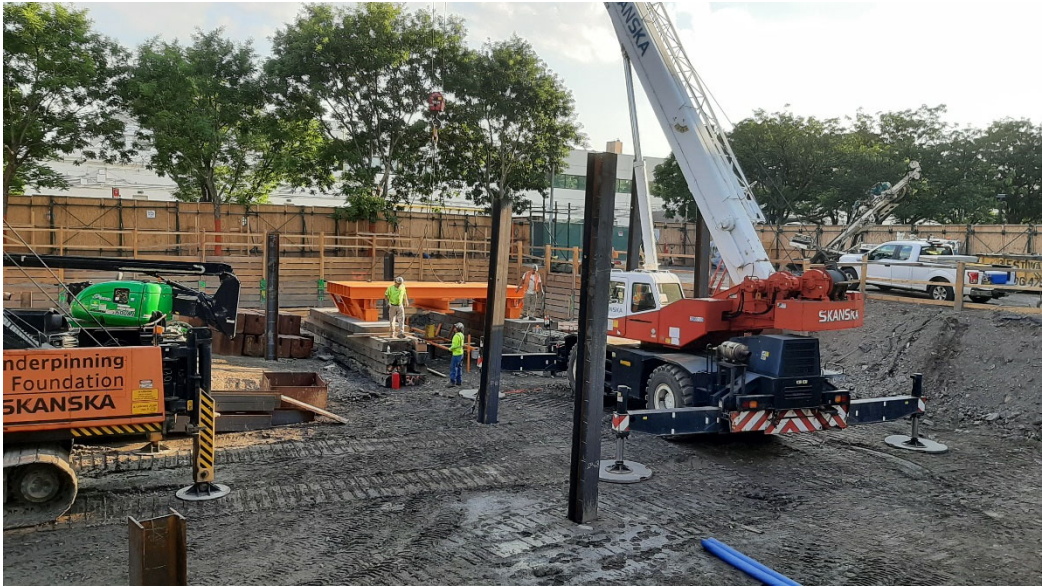
Photo 1: View facing northeast, pile load testing in progress.
