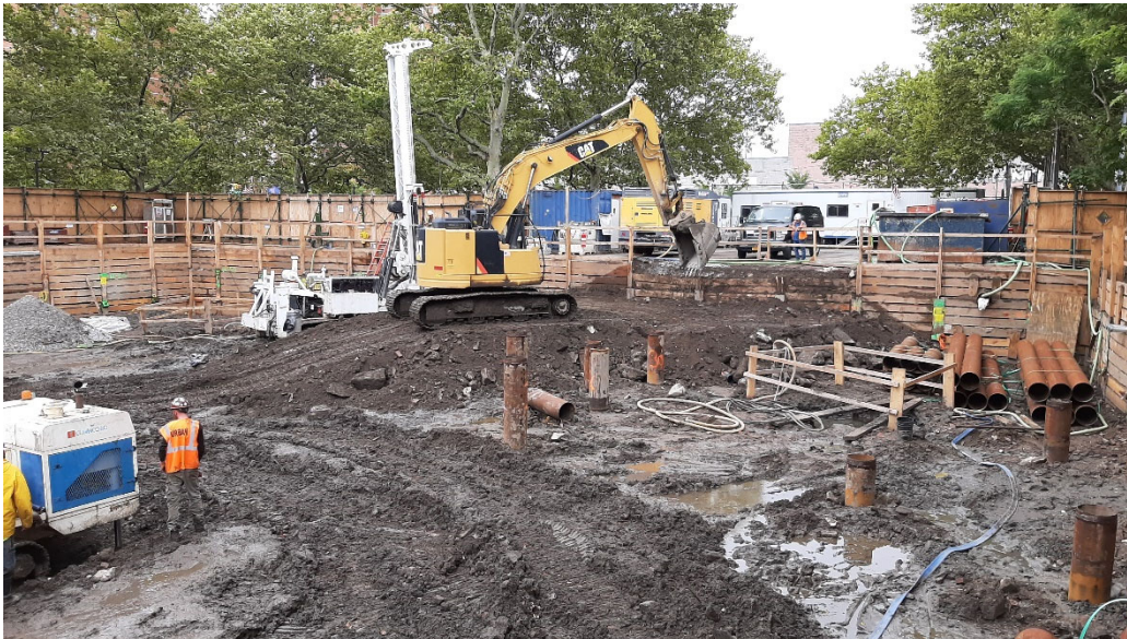
Photo 2: Looking southwest, view of excavator lowering the soil ramp along the west perimeter of the excavation.
