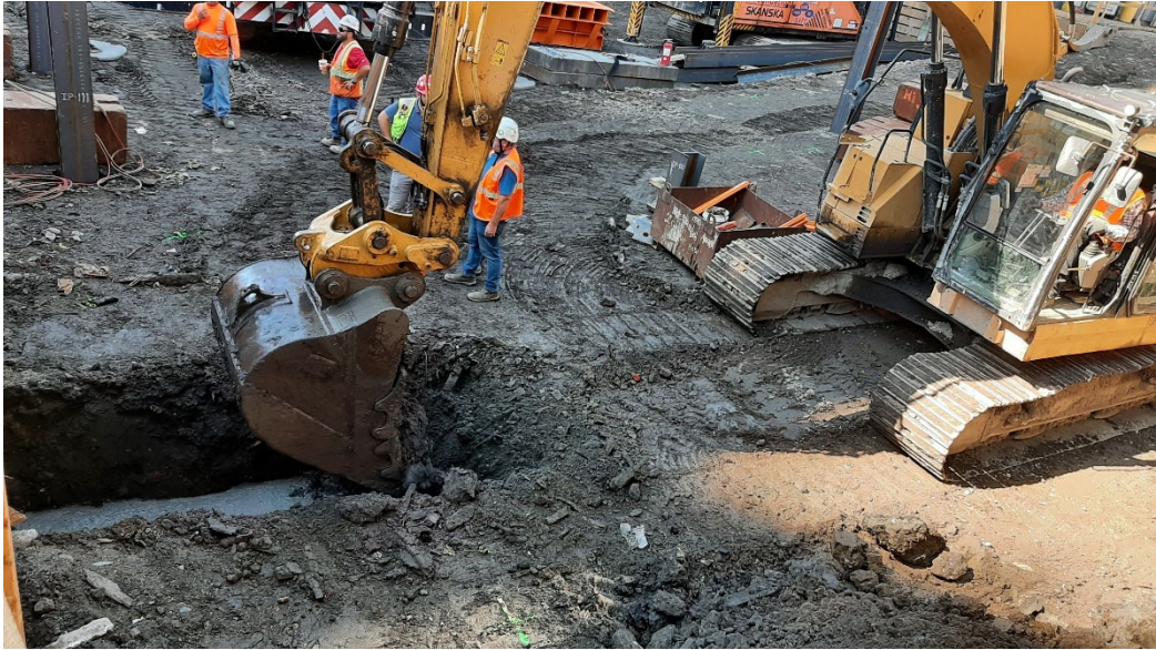
Photo 2: View looking southwest, excavation of test pit to identify cause of refusal.
