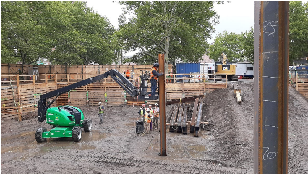
Photo 3: View looking west, GTR removing the attached PDA monitoring equipment from pile.
