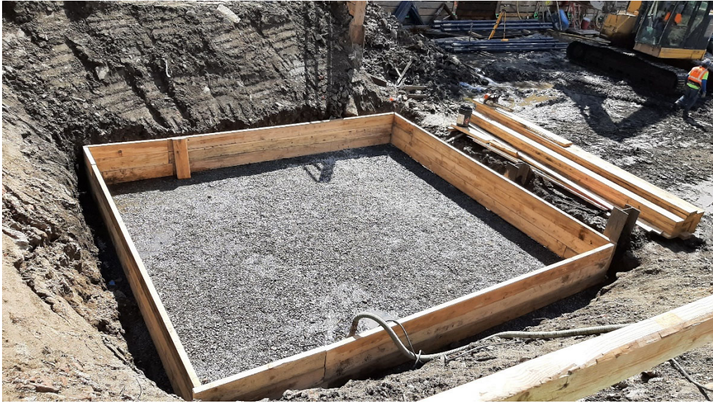
Photo 3: Looking southwest, view of the progress of the detention tank construction, which includes formwork laid on top of the gravel sub-base.
