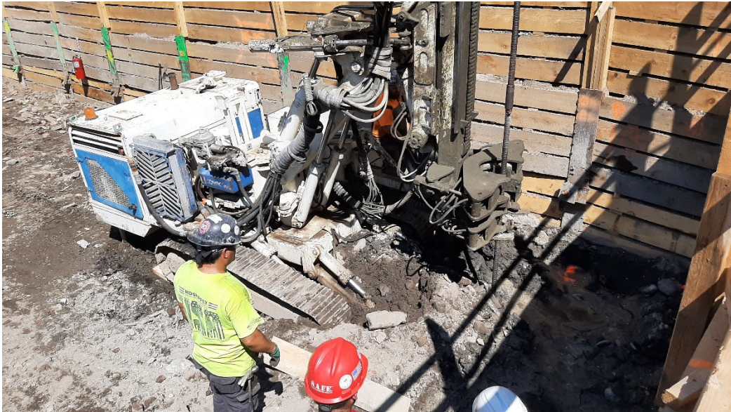
Photo 2: View facing northeast corner, drill rig utilized to test depth to sub-surface refusal point.
