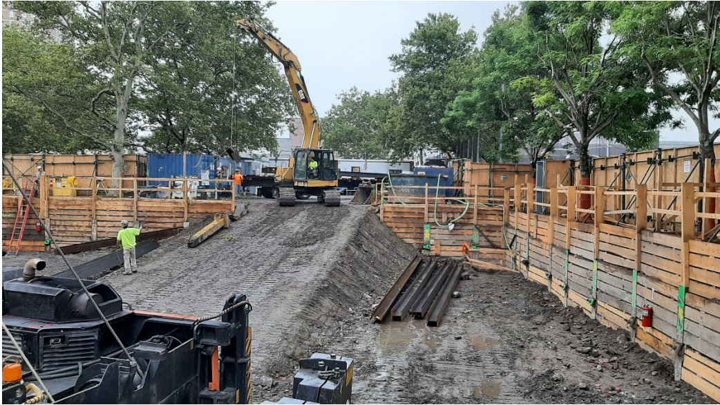
Photo 2: View facing northeast, excavator assisting the unloading of piles for pile driving use into footprint area.
