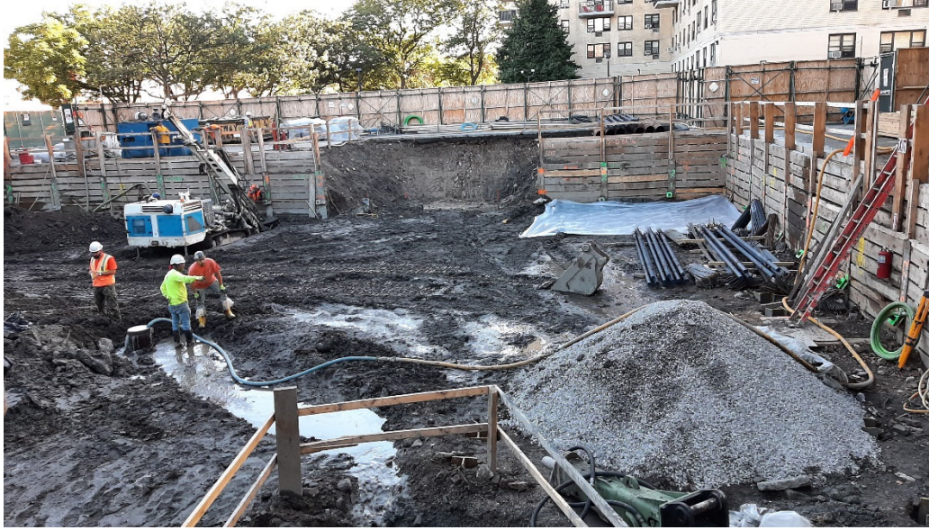
Photo 1: Looking east, view of tiebacks being drilled along the eastern shoring and staging of construction materials for installation of detention tank.
