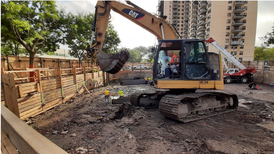
Photo 1: View facing northeast, excavator clearing space for pile driving in northwest area of the building footprint.
