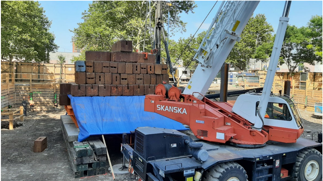
Photo 2: View facing southwest, second test load structure is complete.
