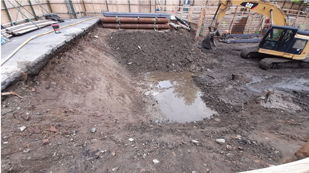
Photo 3: Looking south, view of excavation for detention tank.
