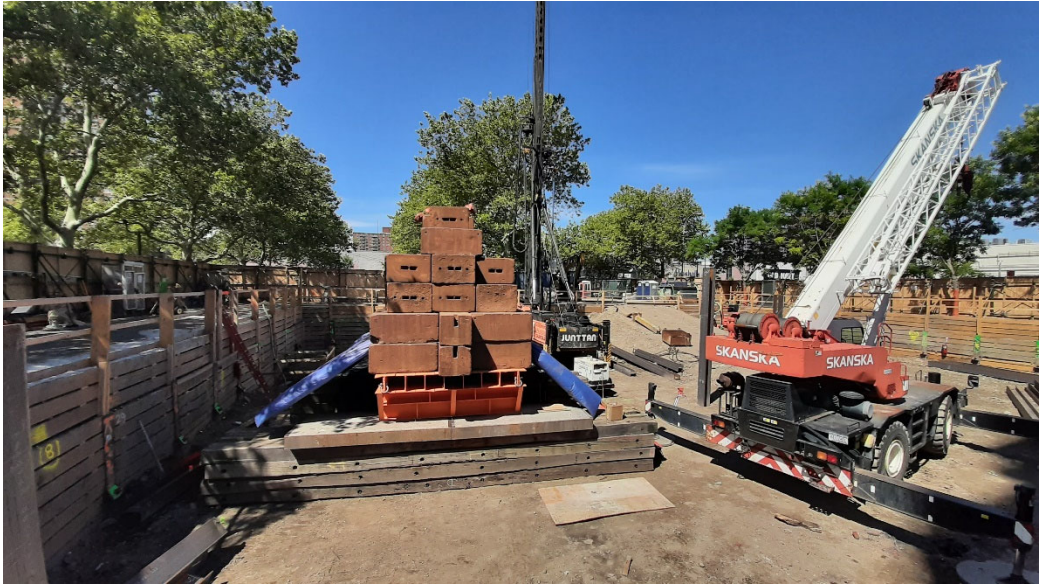
Photo 3: View of the Site facing southwest, conditions of the Site upon pile test load structure completion.
