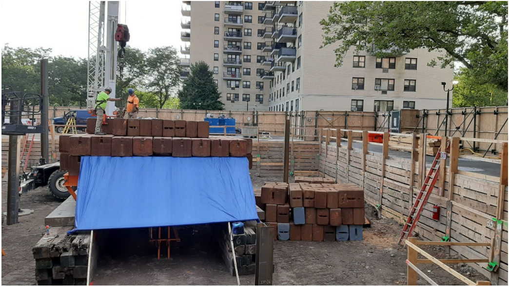
Photo 1: View of southeast area of building footprint, progress of pile load test structure.
