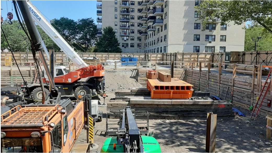
Photo 3: Southeast view of the Site, progress of test load deconstruction by end of day.
