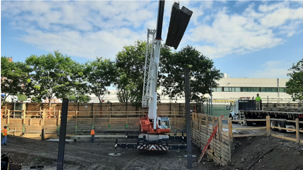
Photo 2: View facing north, crane transporting materials for pile load testing into excavation.
