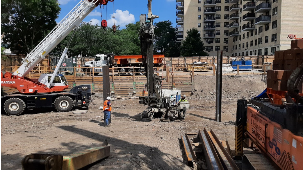
Photo 3: View of the Site facing east, test drilling for refusal depth measurements.
