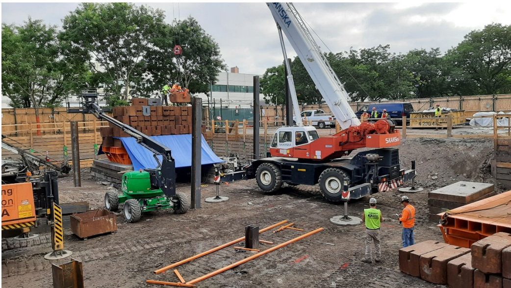
Photo 2: View facing northeast, deloading of the first pile load test structure and setup of the second.
