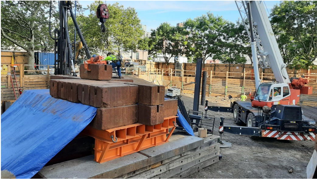
Photo 1: View facing northwest, assembly of pile test load structure in progress.
