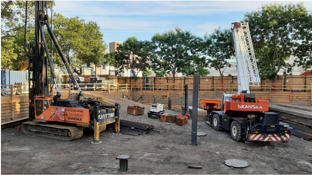
Photo 1: View facing northwest, site conditions at the start of day. Pictured front center, second load test pile.
