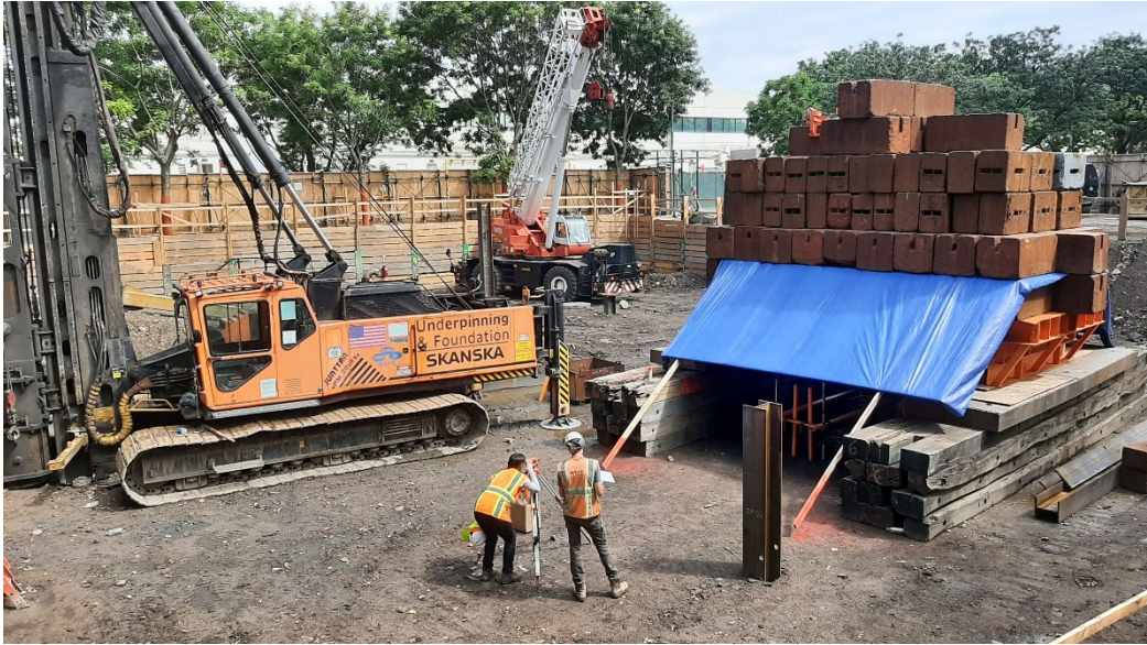
Photo 3: View of the Site facing northeast, MRCE performing pile load testing analysis.
