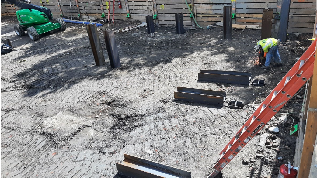
Photo 3: Progress of pile driving work done within the south-southwest area of the building footprint.
