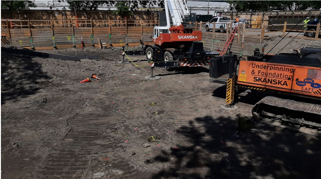
Photo 3: Progress of pile driving work done within the south-central portion area of the building footprint. Also pictured, pile markers applied for upcoming work.
