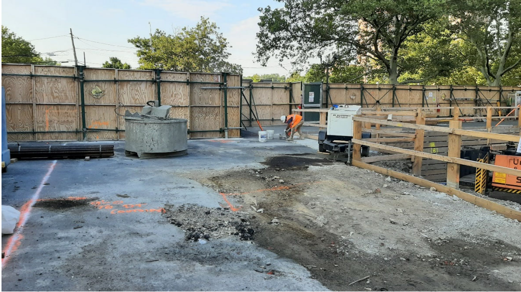
Photo 1: View facing southeast of Track 4 zone, Urban cutting asphalt for detention tank area.
