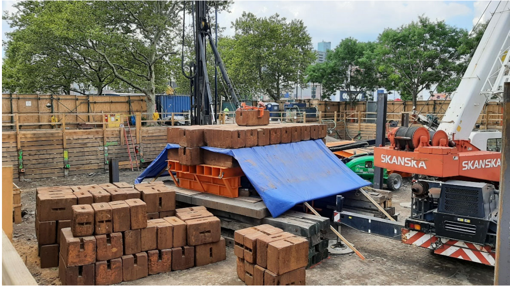
Photo 3: View of the Site facing west-southwest, progress of second pile load test structure by the end of day.
