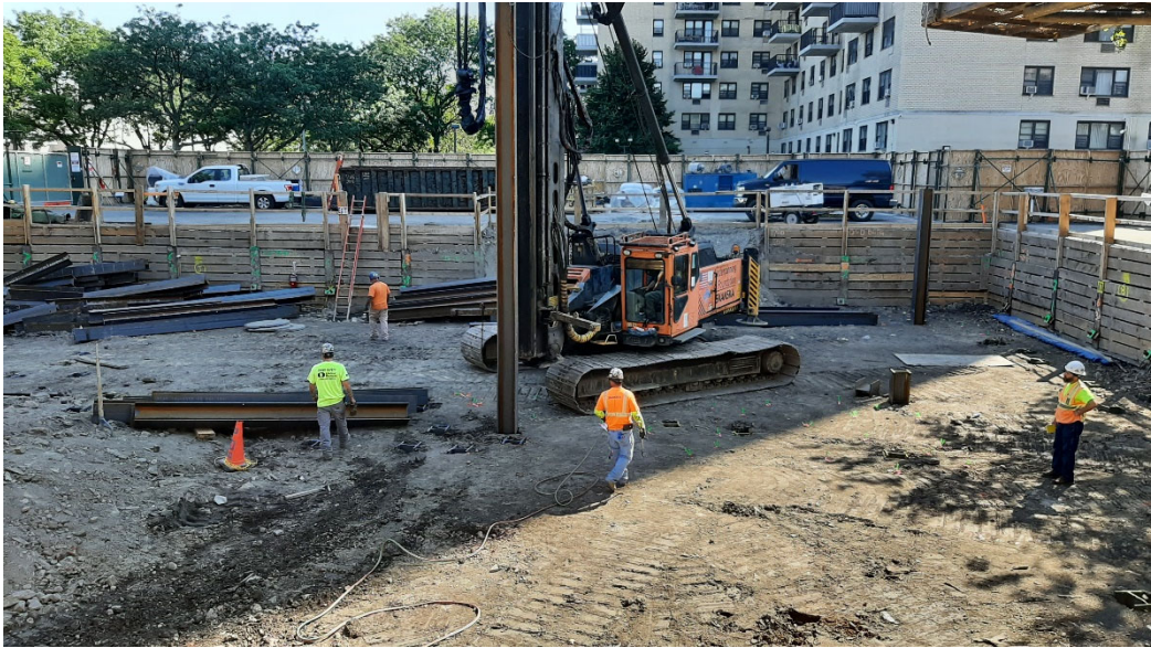
Photo 1: View facing east, pile driving work in progress within the building footprint .
