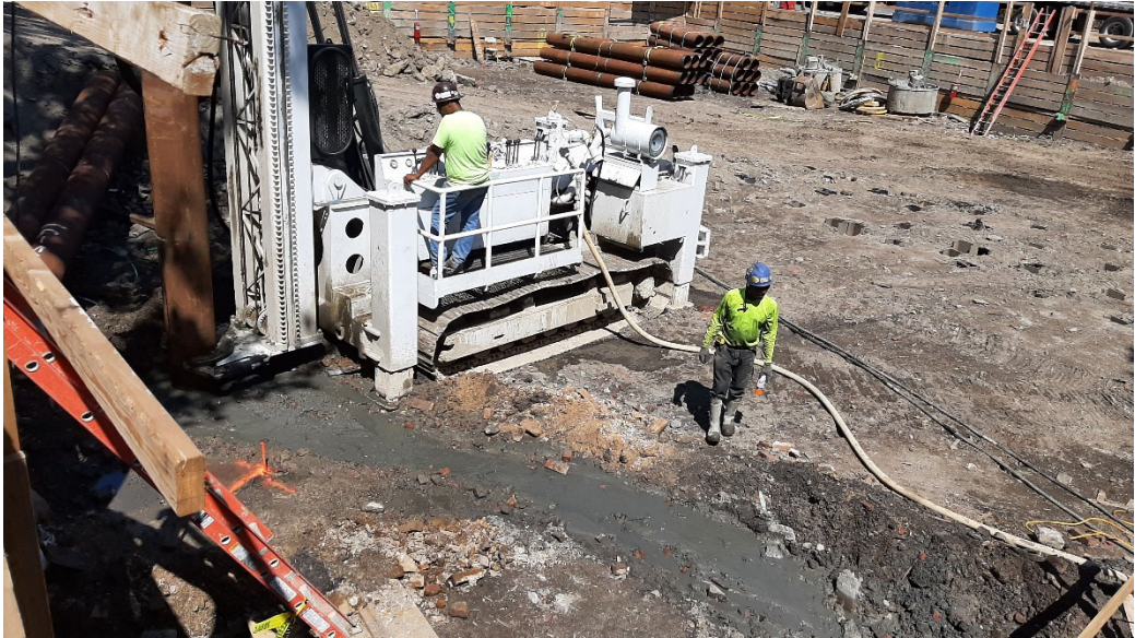
Photo 3: Looking east, drill rig advancing grout casings within building footprint.
