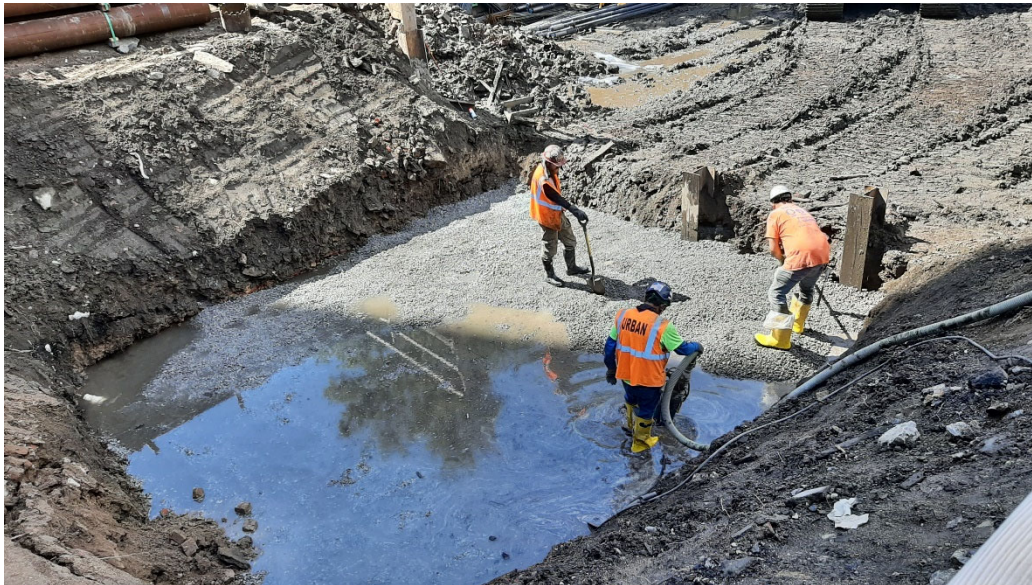
Photo 2: Looking southwest, view of Urban dewatering the excavation for the detention tank and adding the gravel sub-base.
