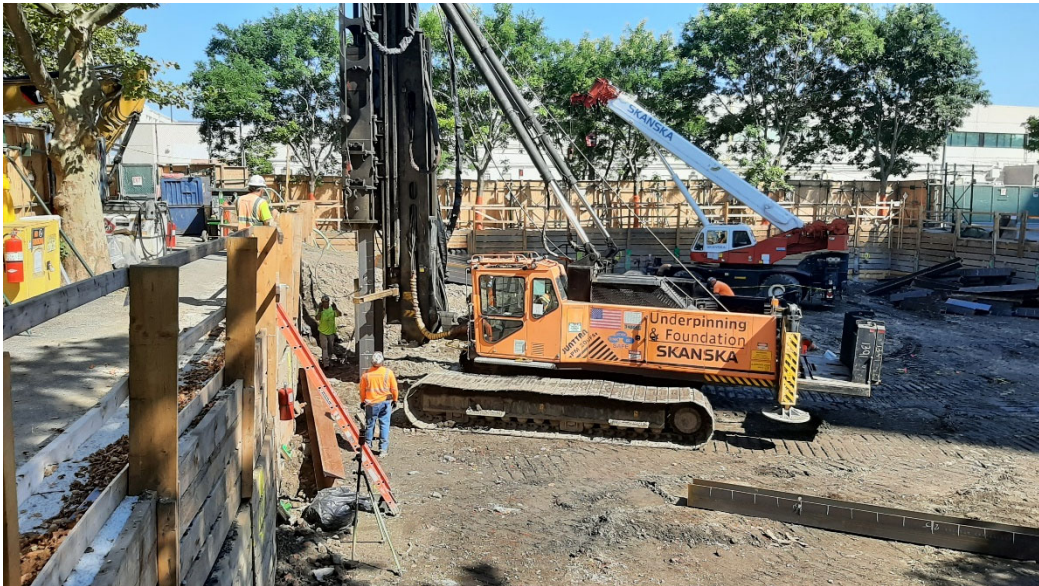
Photo 2: View facing north, progress of pile driving work along western perimeter of building footprint.
