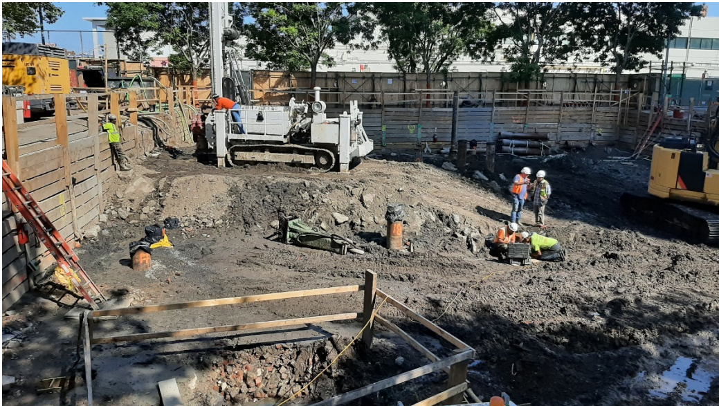
Photo 2: Looking north, view of MRCE analyzing sub-surface conditions and Urban drilling pile casings within the building footprint.
