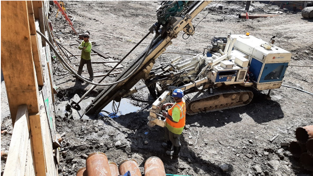
Photo 2: View of secondary tieback work along east-northeast shoring, .
