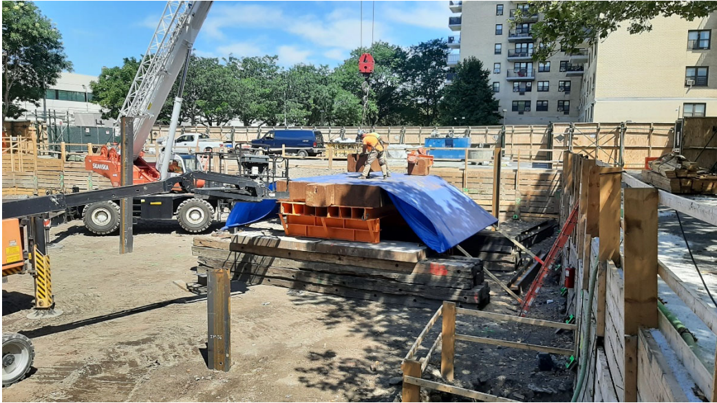
Photo 3: View of the Site facing southeast, assembly of third load test structure.
