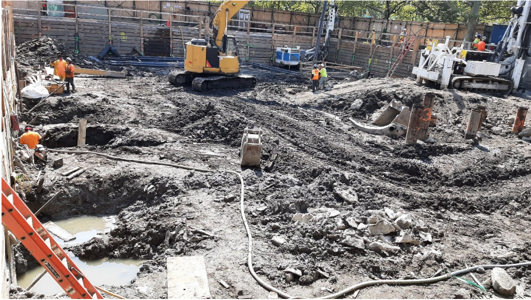
Photo 3: Looking southwest, view of Urban reinforcing tiebacks and dropping rebar into pile casing within the building footprint.
