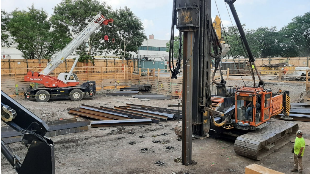
Photo 3: Progress of pile driving work done within the south-central portion area of the building footprint.
