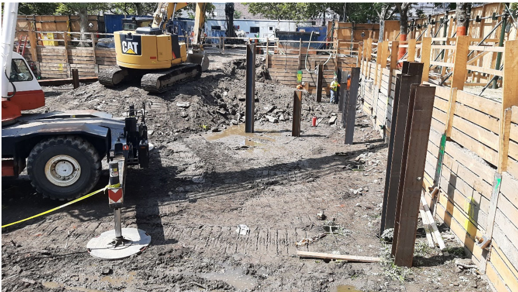
Photo 2: View facing west, progress of pile driving work along northern perimeter.
