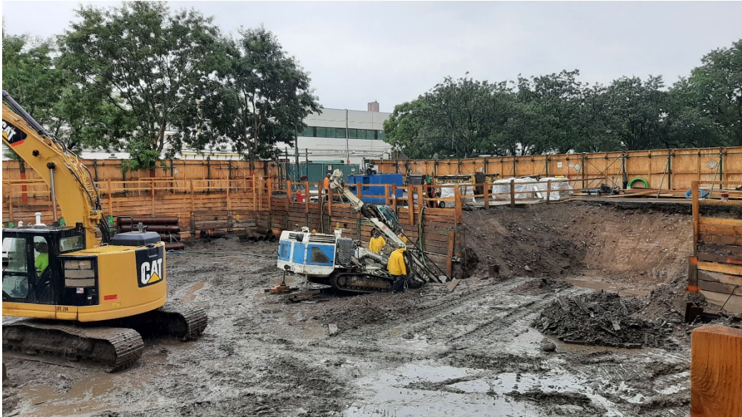
Photo 2: View of tie-back drilling along the eastern shoring.
