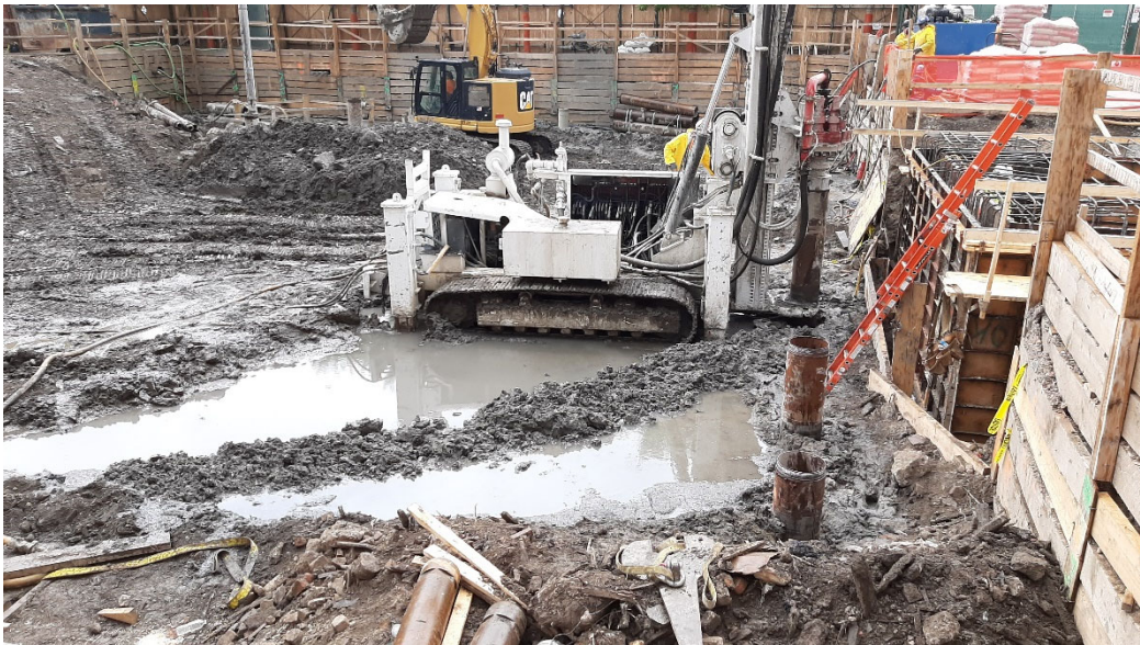
Photo 2: Looking north, drilling of pile casing along the central eastern shoring of the building footprint.
