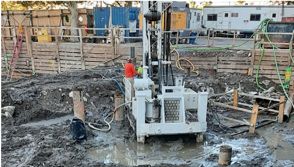
Photo 2: Looking west, drilling of pile casing within the building footprint.
