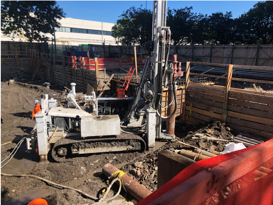
Photo 2: Looking northeast, drilling of pile casing in the southeast corner of the building footprint.
