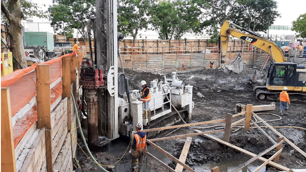
Photo 1: Facing north, view of well drilling in the southwest corner of the building footprint.
