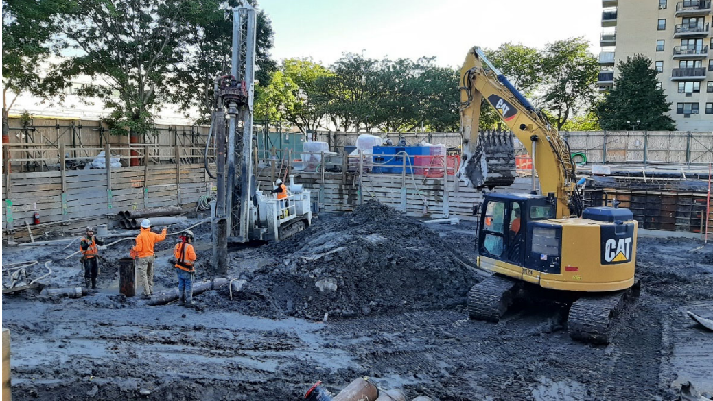
Photo 1: Looking northeast, drilling of pile casing and modification of digout for grout mixing.
