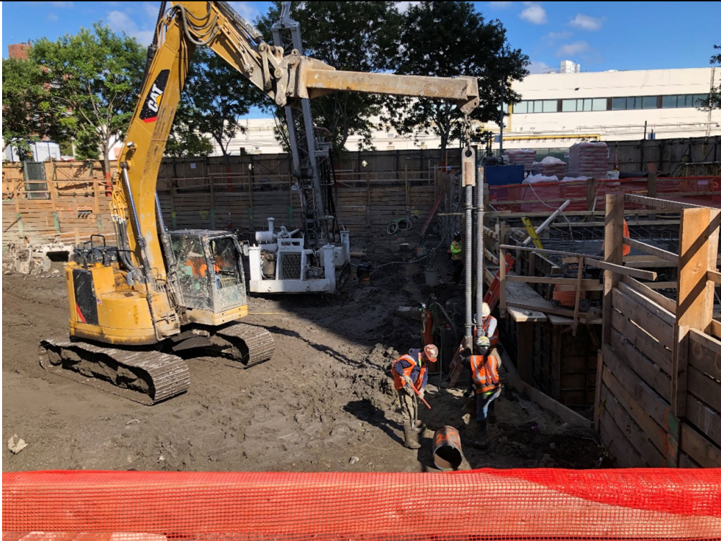
Photo 1: Facing north, steel rods being installed into pile casing along the east shoring.
