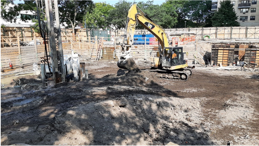
Photo 3: View facing east, Urban excavates digout for grout mixture to be injected into pile casing.
