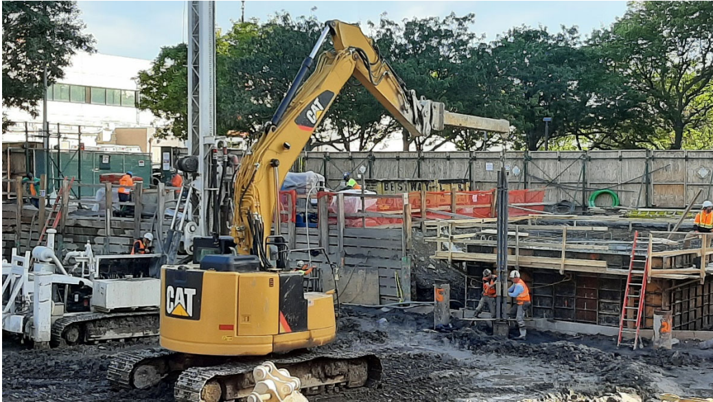
Photo 3: Looking northeast, progress of pile casing work along the east shoring of the building footprint.
