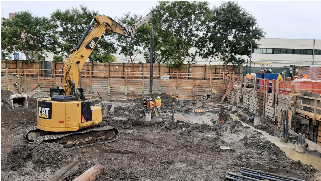
Photo 2: Facing north, steel rods being inserted in to casing in the central east region of the building footprint.
