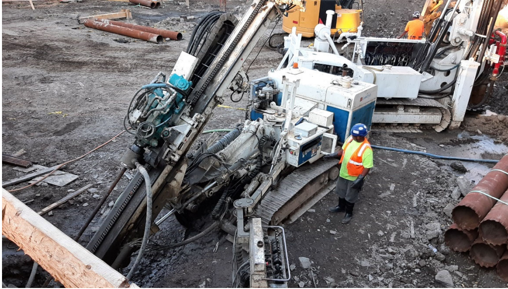
Photo 1: View of tieback drilling into east-northeast shoring.
