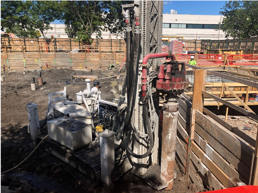
Photo 2: Facing north, view of case drilling in the southeast corner of the building footprint.
