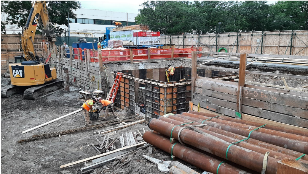
Photo 1: Looking northeast, progress of formwork assembly in the detention tank area.
