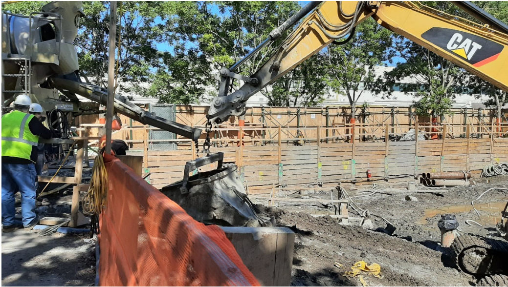
Photo 2: Looking northwest, Urban receiving delivery of cement for detention tank structure.
