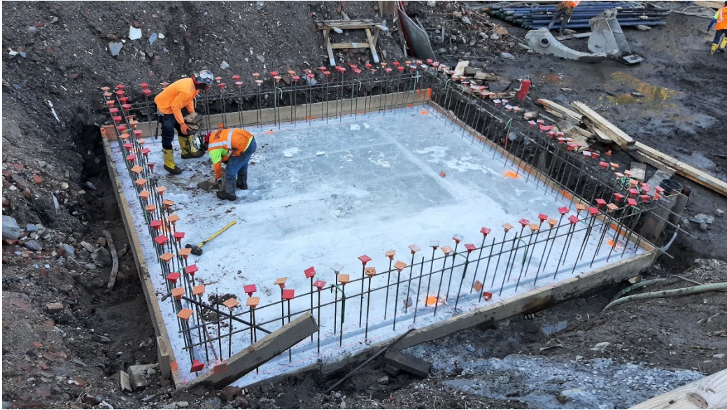
Photo 3: View of concrete pad for detention tank.
