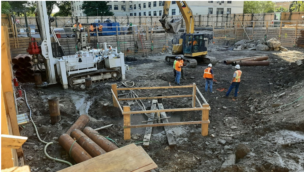
Photo 2: Looking east, view of surveyors plotting markers for pipe casing drill work within the building footprint.
