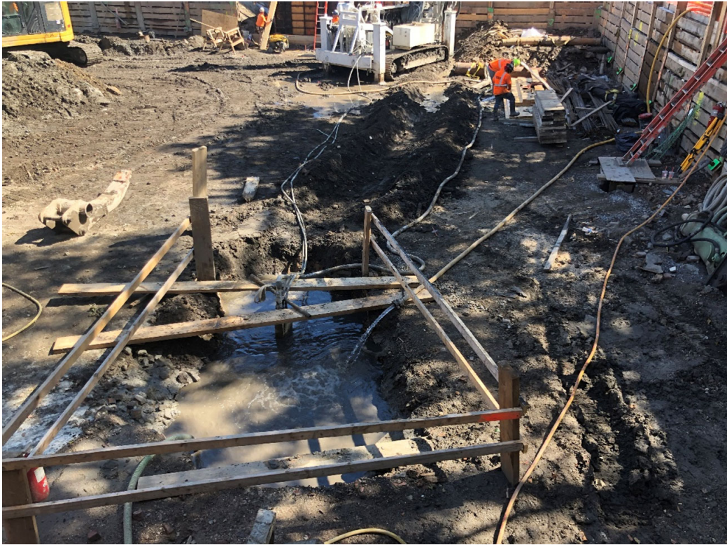
Photo 3: Looking east, digout made in southwestern corner of Site for drilling the pile casing.
