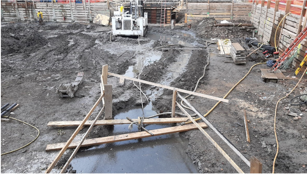
Photo 3: Looking east, digout made in southwestern corner of Site for drilling of the pile casing.
