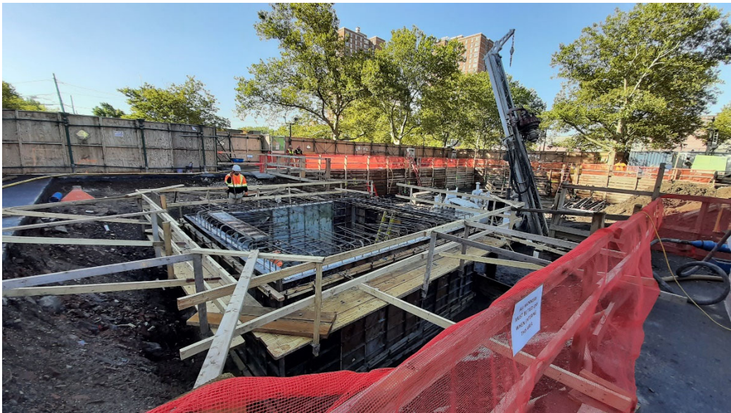
Photo 2: Looking southwest, progress of formwork assembly in the detention tank area.
