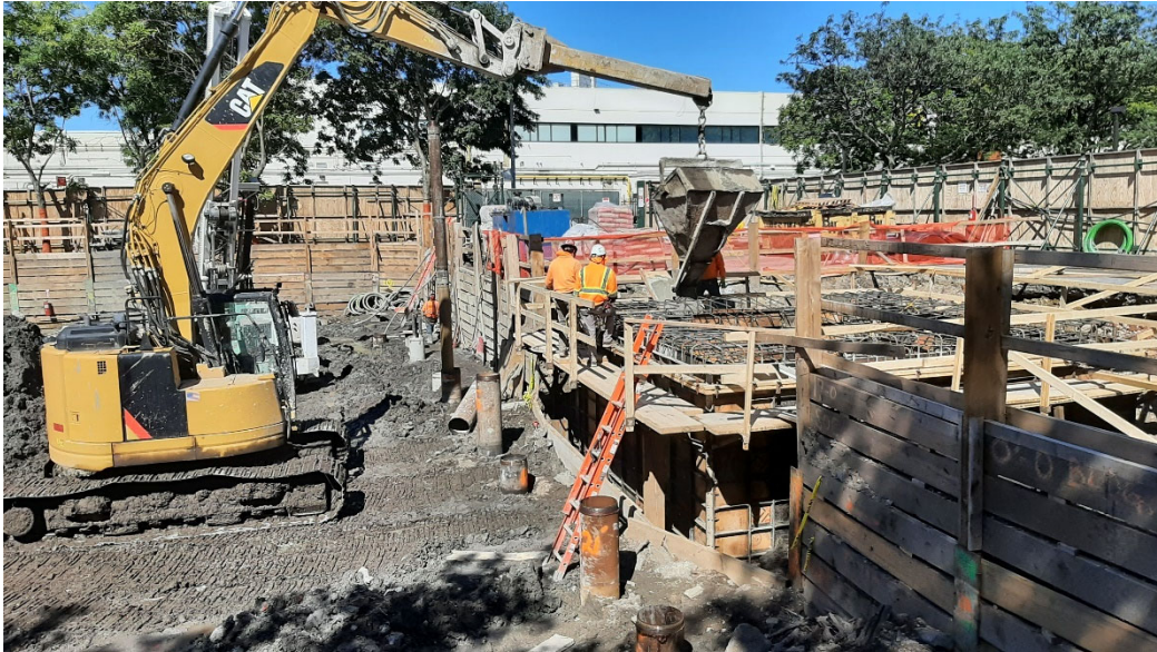
Photo 3: Looking northeast, pouring of concrete for the walls of the detention tank structure.
