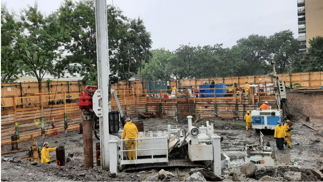
Photo 1: Looking northeast, view of drilling pile casings within the building footprint.
