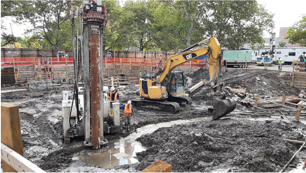
Photo 3: Drilling of pile casing and modification of terrain for grout mixing path in the northeast area of the Site.
