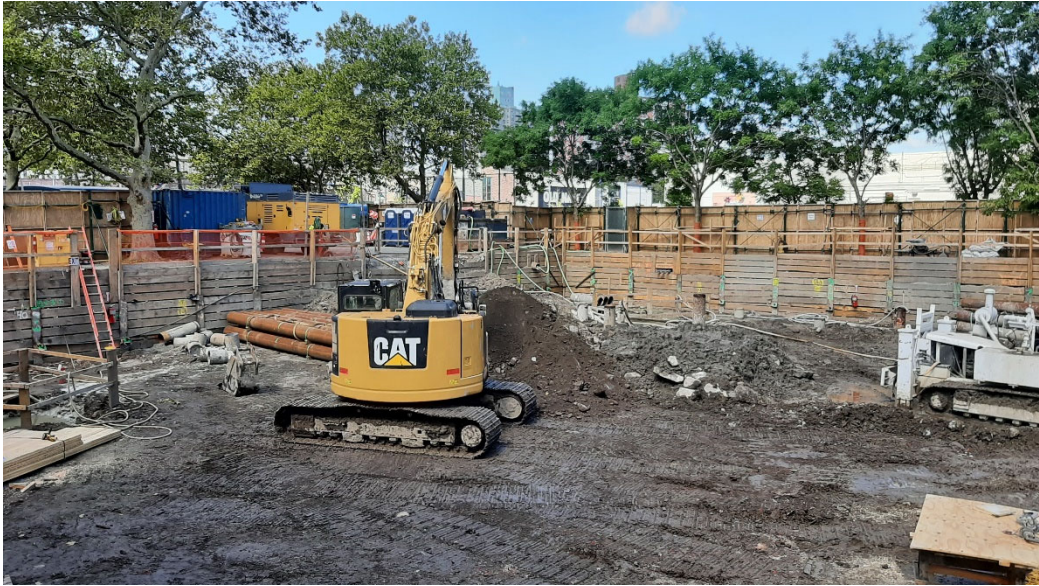
Photo 3: Looking northwest, excavator removes soil from ramp.
