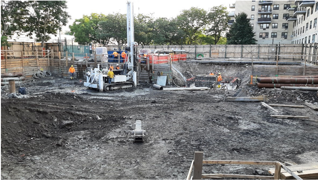
Photo 1: Looking east, drilling of pile casings along the eastern shoring and assembly of formwork in the detention tank area.
