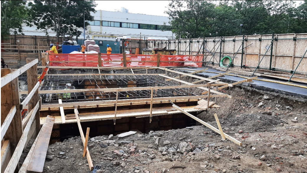
Photo 1: Looking north, progress of formwork assembly in the detention tank area.
