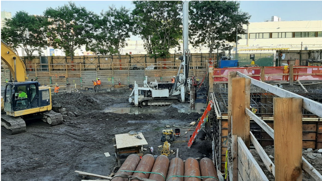
Photo 2: Looking north, drilling of pile casing in the northern half of the building footprint.
