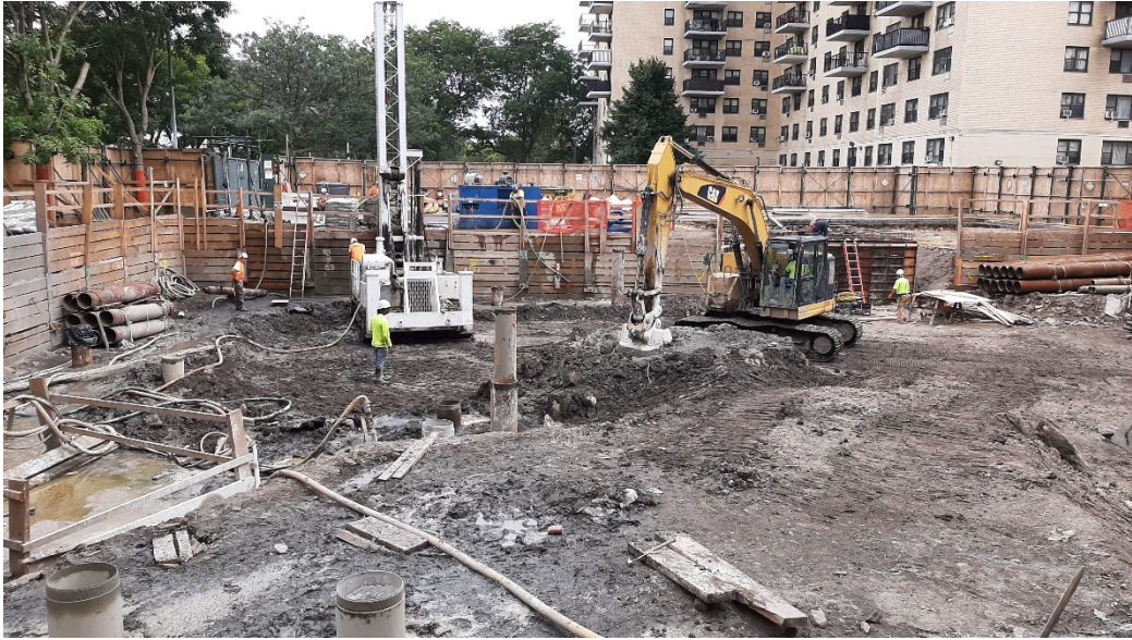
Photo 3: Looking east, drilling of pile casing and excavation of digout for grout mixture along east shoring.
