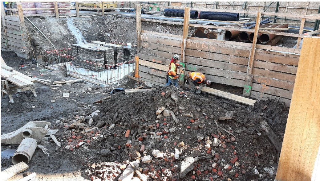
Photo 2: Looking east, Urban repairs shoring that was damaged from inclement weather.
