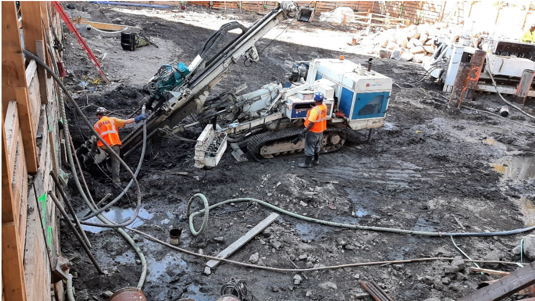
Photo 2: View of tie-back drilling and dewatering along east-northeast shoring.
