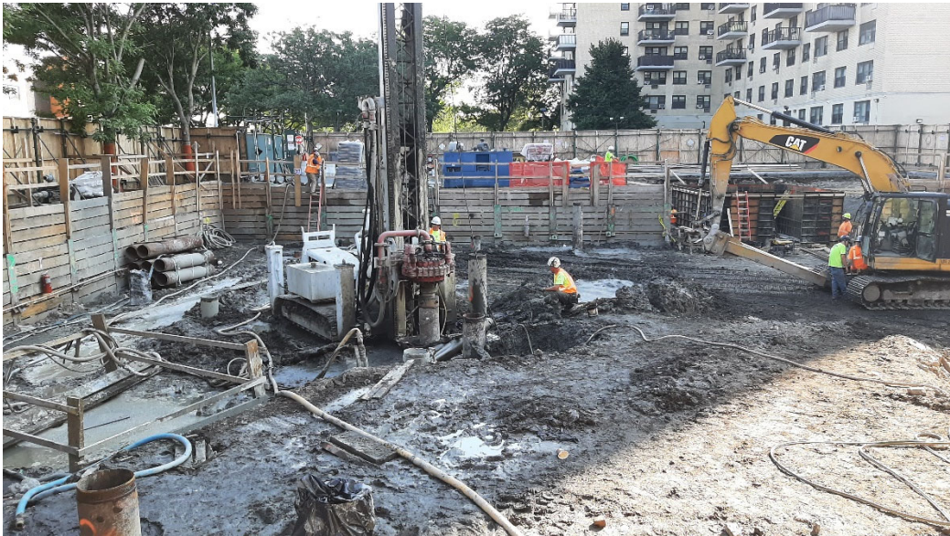
Photo 2: Looking east, drilling of pile casings in the northern half of the building footprint.
