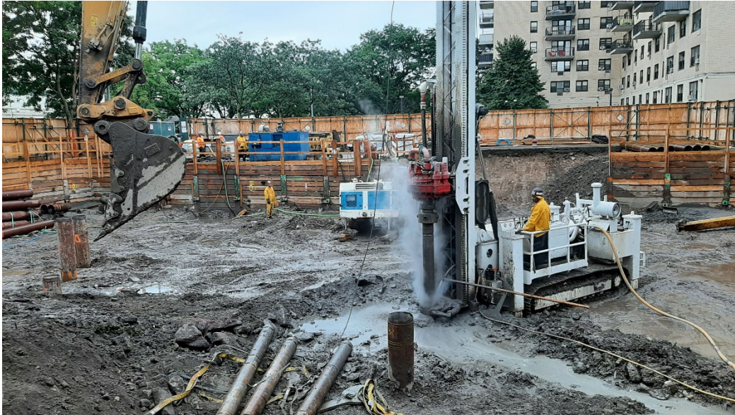
Photo 3: Looking east, view of pile casing drilling work in the center of building footprint.
