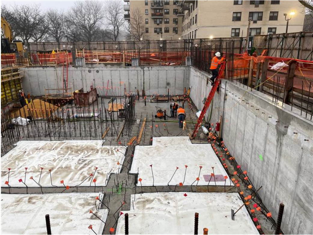
Photo 2: View facing east, foundation waterproofing in southern portion of the building footprint.
