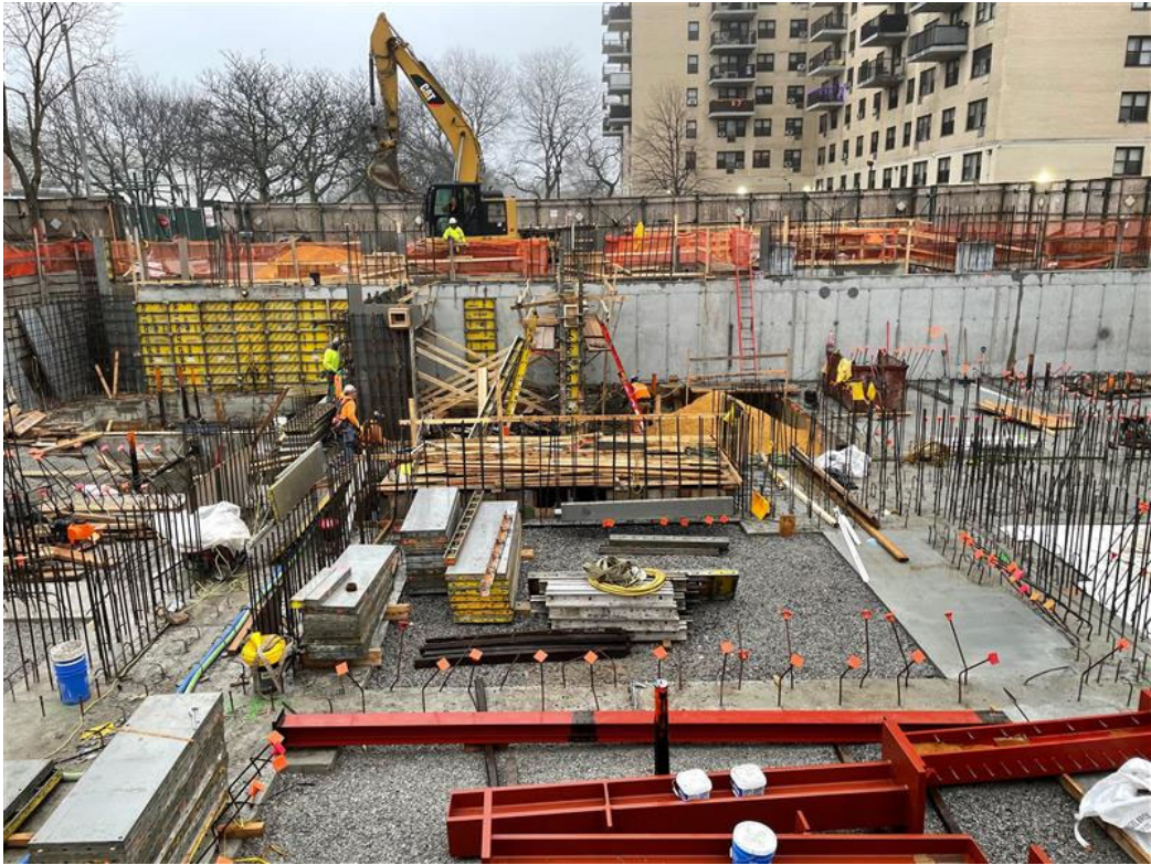
Photo 1: View facing east, concrete form work and rebar installation in grid BDS-4. Import of NYSDEC-approved backfill in grid BDS-6.
