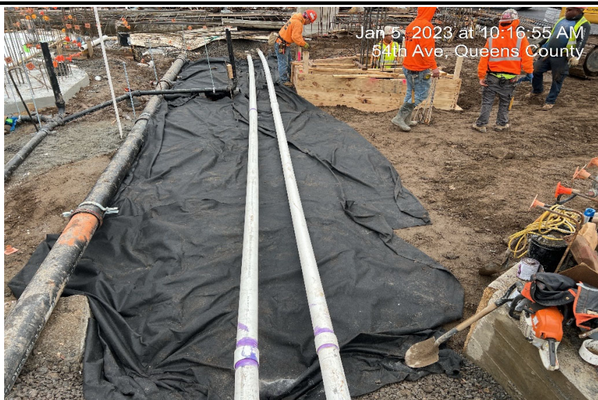
Photograph 2 - CCJV completes installation of SSDS system in WC-11, view facing east.
