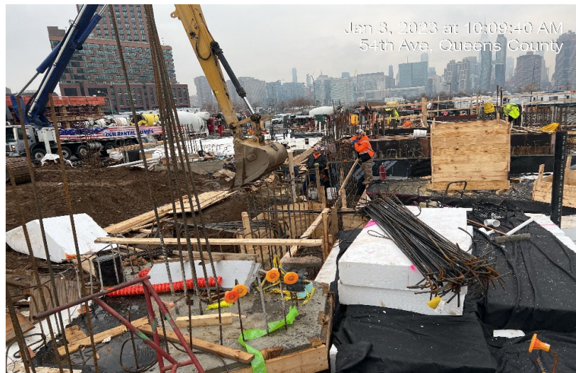
Photograph 1 - Civetta backfills material around pile caps in WC-11, view facing west.
