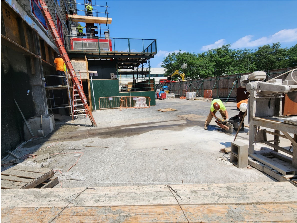
Photo 2: Facing northeast, URBAN cutting through the asphalt cap for Siamese standpipe trench.
