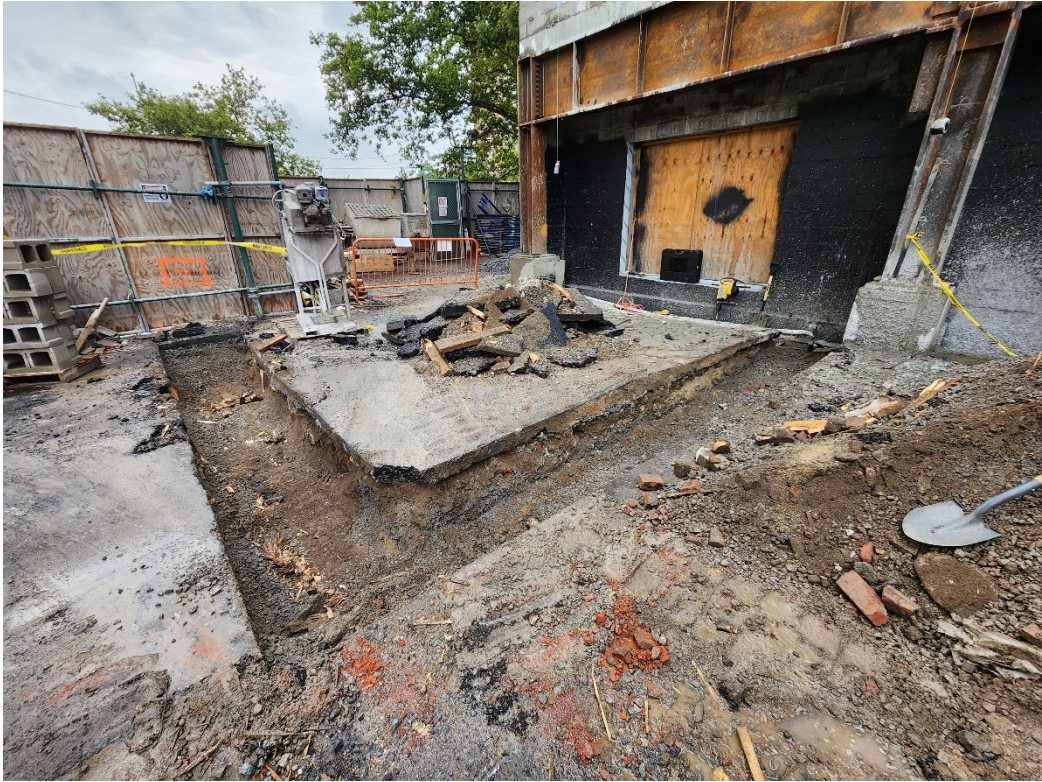
Photo 2: Facing south, general view of Siamese standpipe trench after the excavation was completed.
