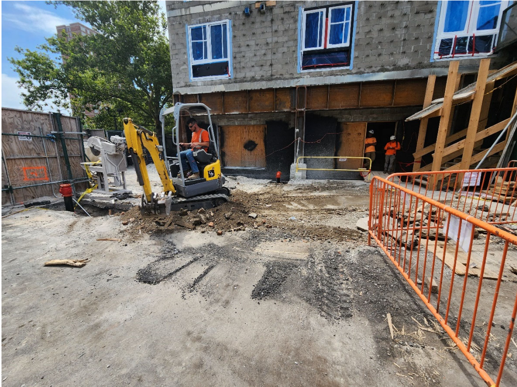
Photo 2: Facing southwest, URBAN backfilling the trench with DEC- approved backfill.
