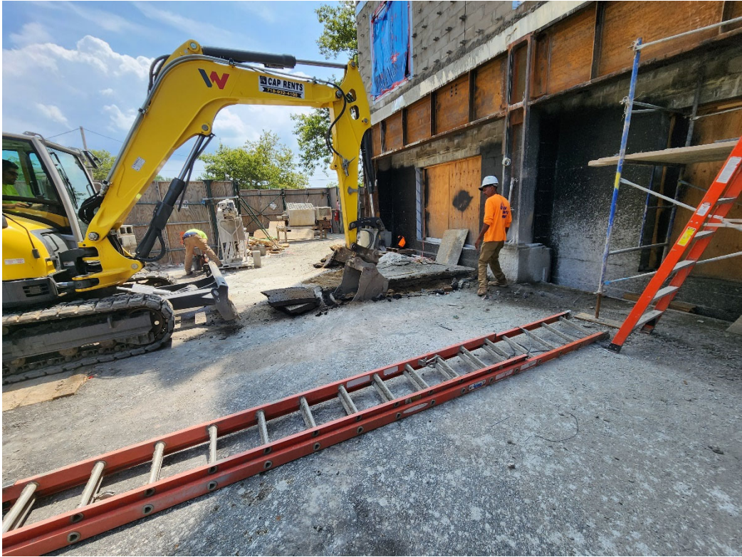
Photo 3: Facing south, URBAN removing the cut asphalt for the trench.
