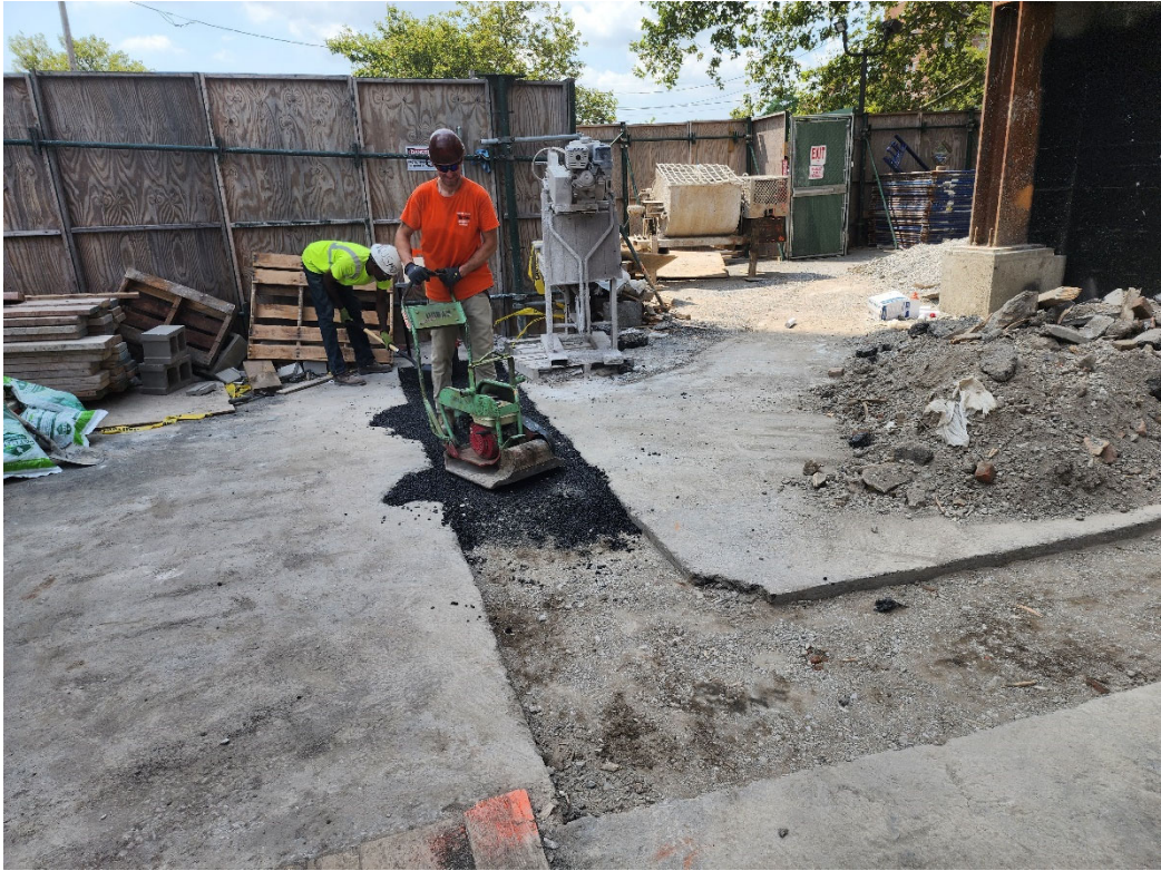
Photo 2: Facing southwest, URBAN compacting and leveling the asphalt.
