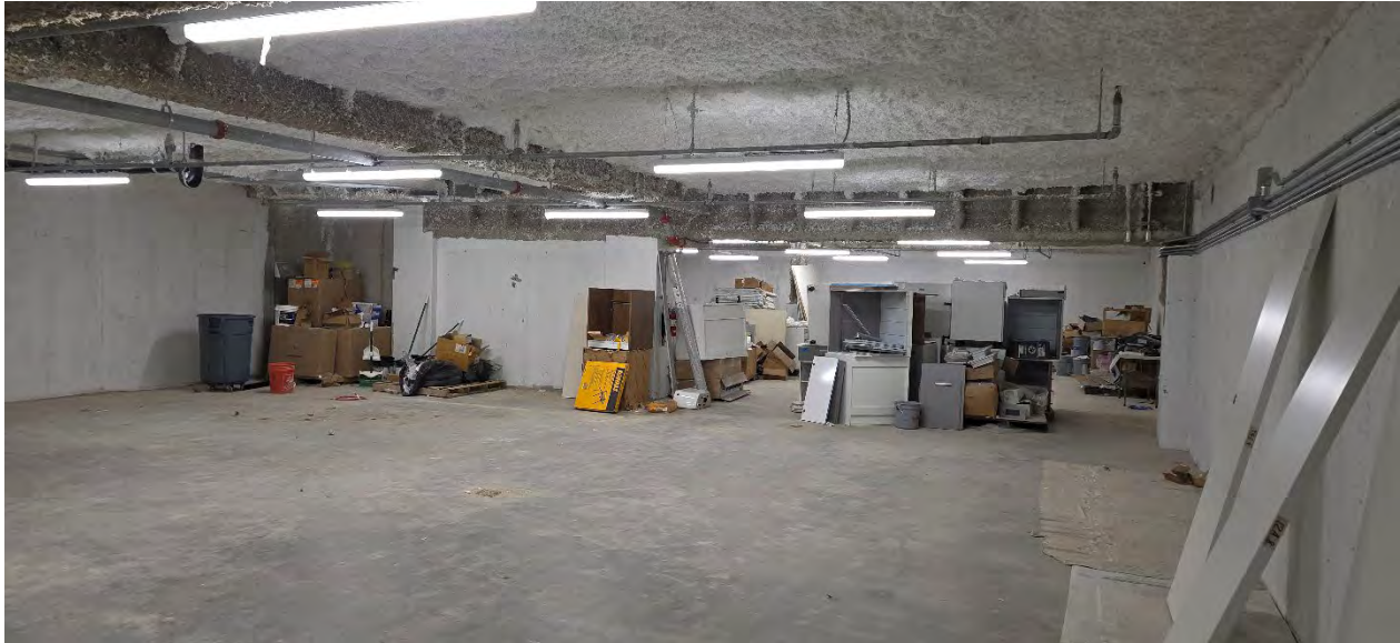
Photograph 5: Photo inside 1940 Turnbull Ave building basement within the northwest corner of the building facing south (Track 2).
