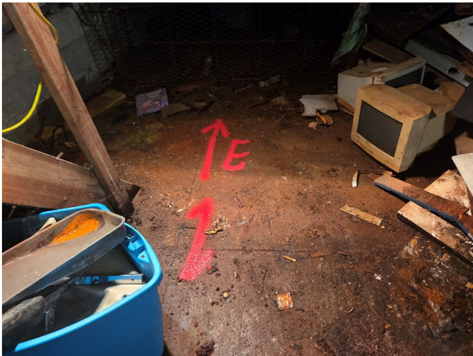
Photos 8 & 9 – Views of the basement below the barber shop. The accessible areas within the basement were investigated for subsurface findings and one electrical line was detected.
