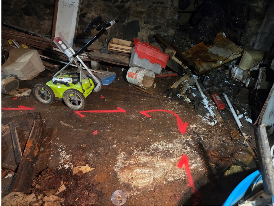
Photos 8 & 9 – Additional views of the basement below the barber shop. The detected electrical line and cleared boring location were marked here.
