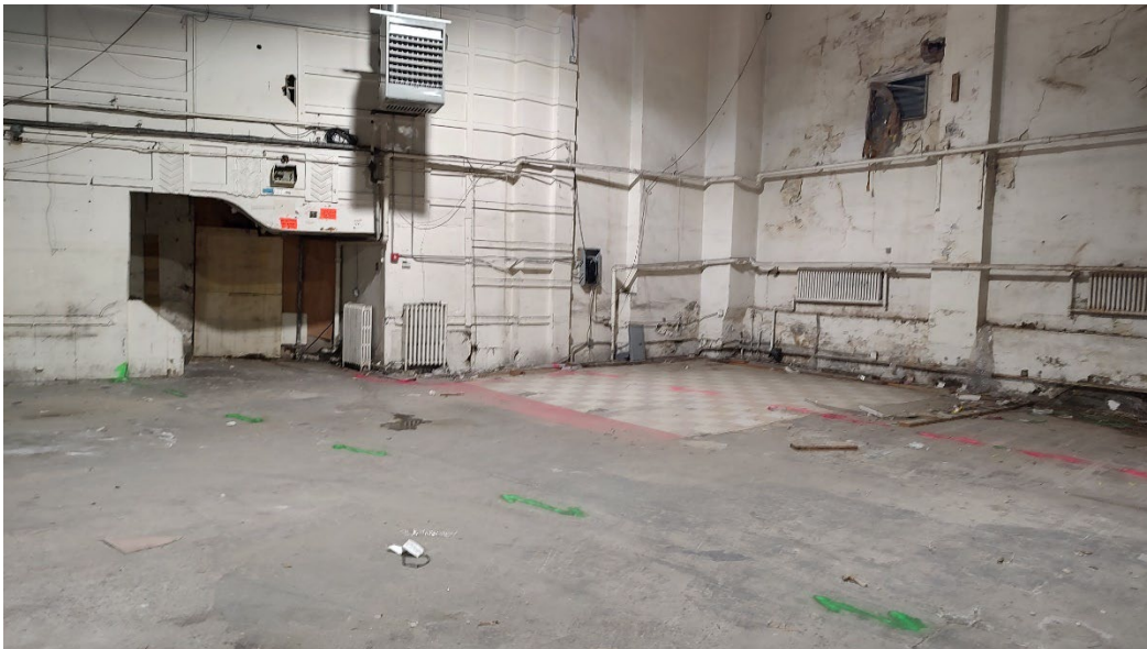
Photos 1 & 2 – Views of the north end of the former kitchen warehouse at the location of the roof drain (marked in green) and the unknown line (marked in pink). The unknown line may have been related to the former hot water based heating system.
