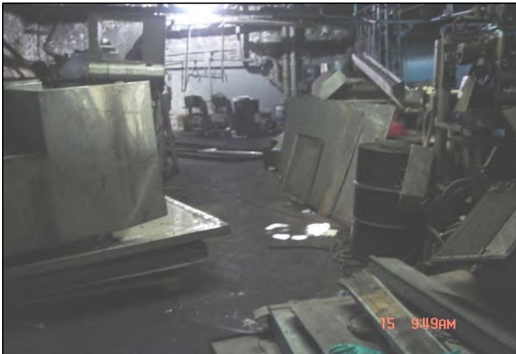
Photograph 15: 1560 Boone basement storage area.
