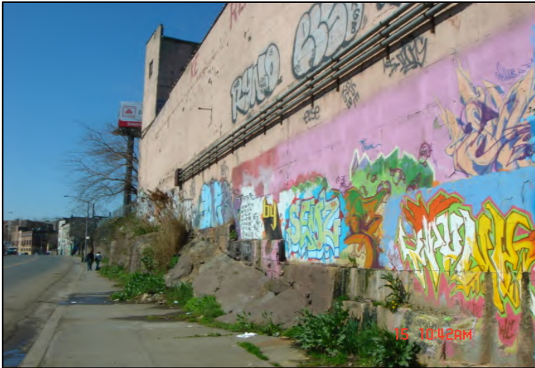
Photograph 5: 1560 Boone along West Farms Road facing SW; observe the exposed bedrock .
