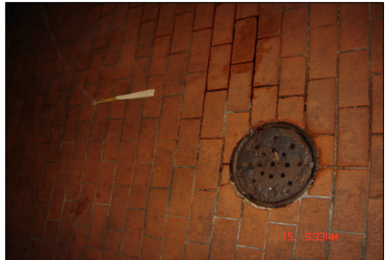
Photograph 8: Floor drains observed throughout.
