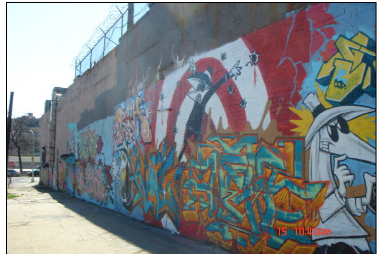
Photograph 4: 1560 Boone along E 173 rd St, facing SE
