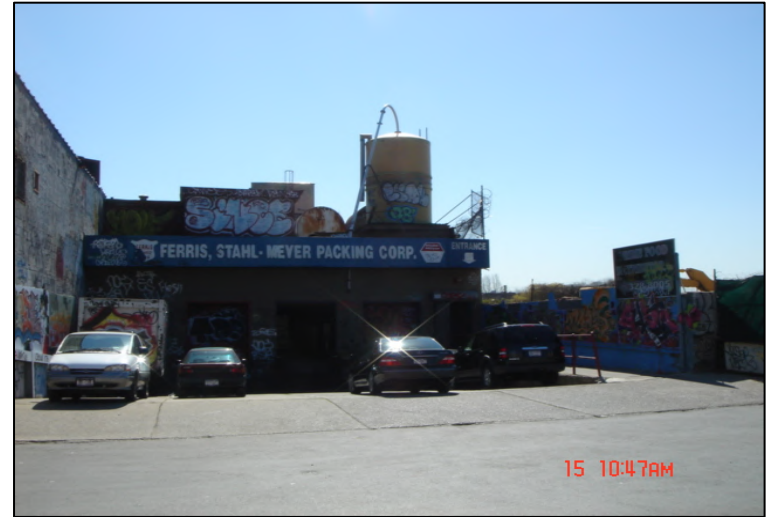
Photograph 2: 1560 Boone; Royal Foods loading dock, observe old chilling tanks on the roof.
