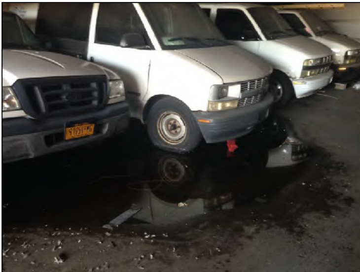
Photograph 15. A puddle on the southern side of the building, apparently due to a roof leak.
