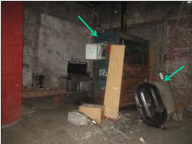
Photograph 11. A hydraulic lift and an approximately 275-gallon aboveground storage tank (AST) in the northeastern corner of the Compass 4 Site building.
