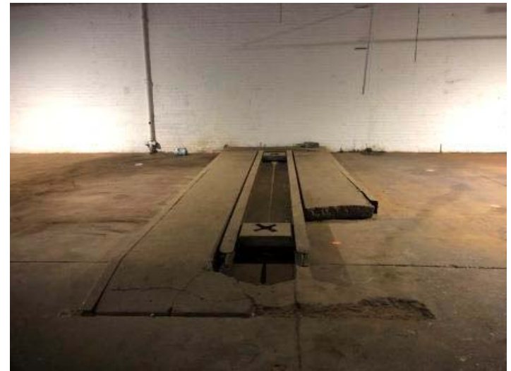
4. Truck lifts located along north wall of building.
