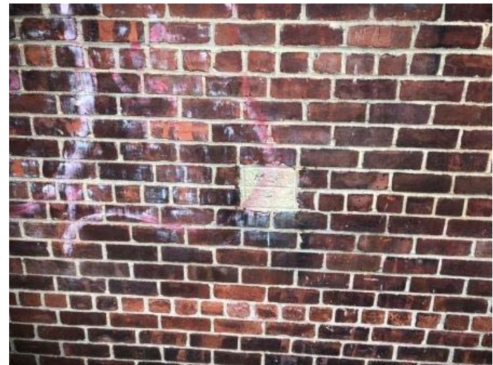
8. Likely former location of fill port associated with former gasoline USTs, located in southeastern quadrant of building bordering Gerard Avenue.
