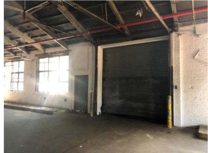
6. Roll up garage door entrance along Gerard Avenue.
