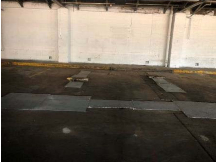
5. Hydraulic lifts located in the southeastern quadrant of the building
