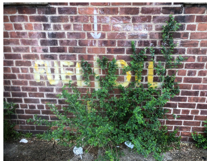
4. Former remote fill along Gerard Avenue for the abandoned 2,500-gallon UST located in the basement.
