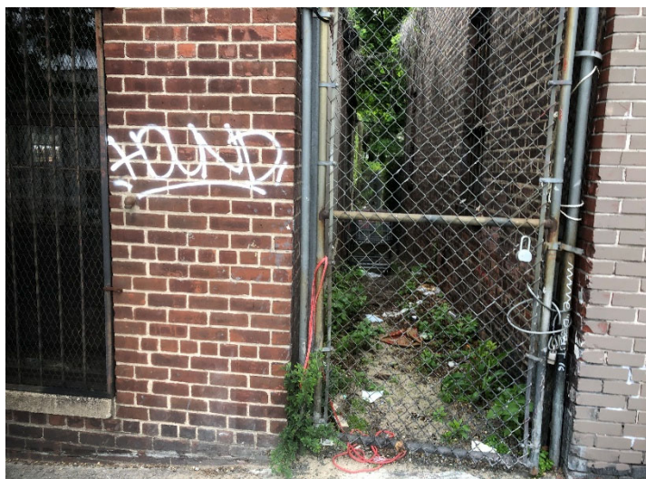
3. View of the entrance to the rear path along 150 th Street.
