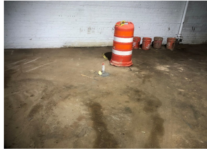
10. Looking at the monitoring well located in the northwest corner of the project site.
