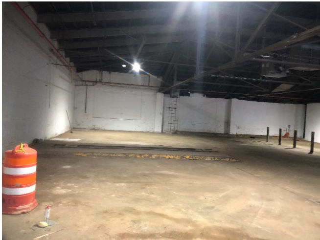
5. View of the former truck lifts located in the northern portion of the building.
