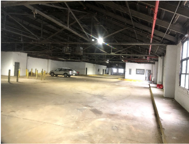
9. View of the building's interior, looking south from the northwestern corner.
