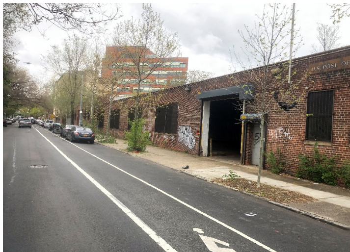
1. Looking at the project site building along Gerard Avenue.
