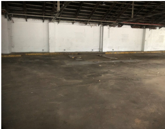
11. View of the former hydraulic lifts located in the southeastern portion of the building.
