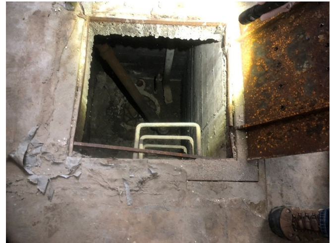
6. View of the sewer connection located near the center of the building.
