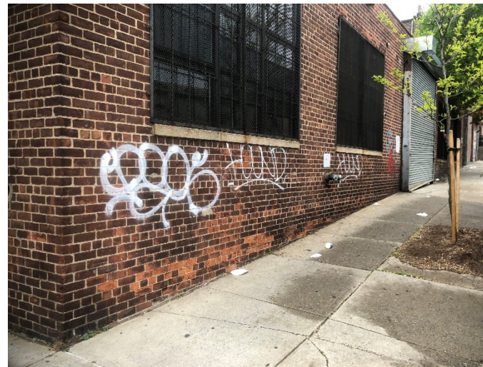
2. Looking along the south side of the building along 150 th Street.
