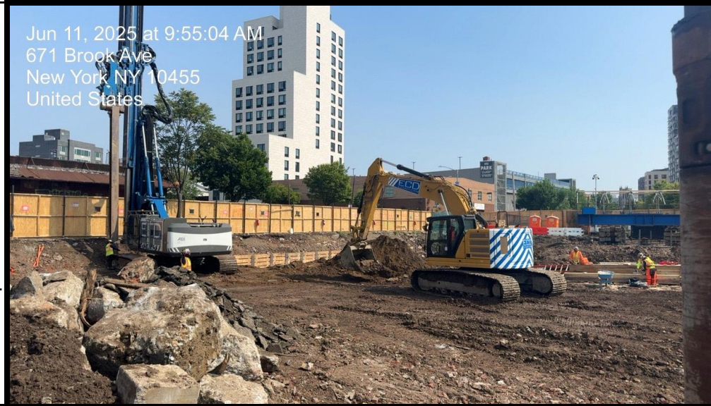
Photograph 1 - ECD installs SOE piles in Grid A12 while excavating soil from Grids A14/16 for export to Bayshore. View facing northwest.
