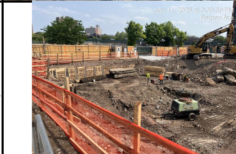
Photograph 3 - Overview of excavation on Lot 26. View facing southeast.
