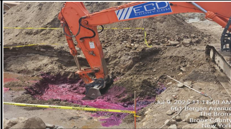
Photograph 3 - ISOTEC and ECD conducting soil mixing using sodium permanganate in Grid A15. View facing south.
