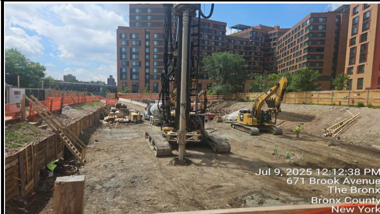
Photograph 1 - RYC NY installing and grouting production piles in Grid A4. View facing south.
