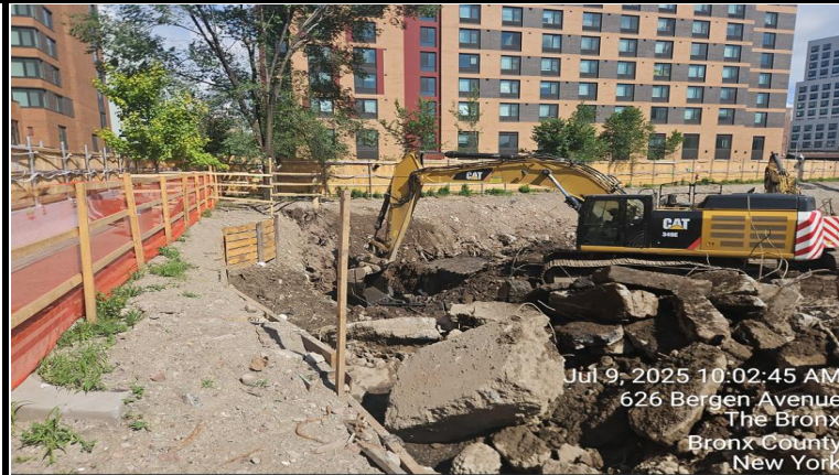
Photograph 2 - Site work in Grids A1- A5. Hazardous lead stockpile staged on two layers of poly (and covered with two layers of poly) in Grid A5 for future off-site disposal. View facing south.
