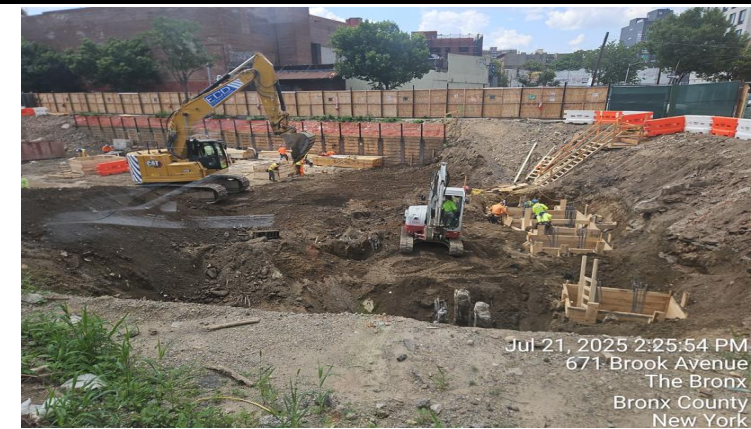
Photograph 3 - A view of ECD site work in Grids A13/A14/A15/A16. View facing west.
