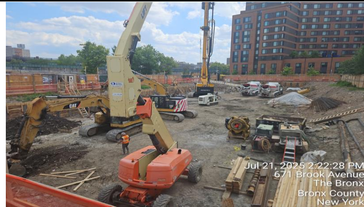
Photograph 2 - A view of RYC NY site work. Hazardous lead stockpile staged on two layers of poly (and covered with two layers of poly) in Grid A5 for future off-site disposal. View facing south.
