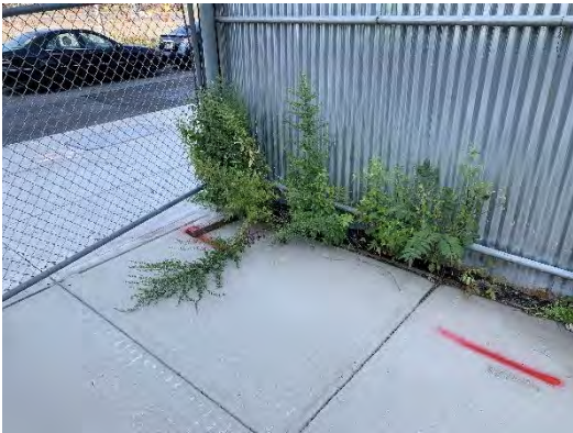
Photo of found conduit (red) located with EM locator.
