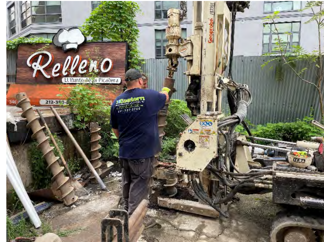
Photo 2: View of MW3 installation.
