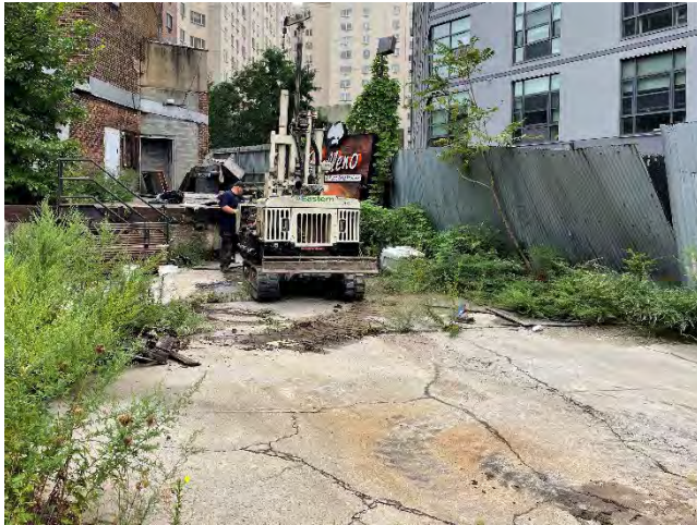
Photo 1: View of drilling at location MW3/SB3/SV3.
