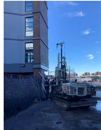
Photo 4: View of MW7 installation.
