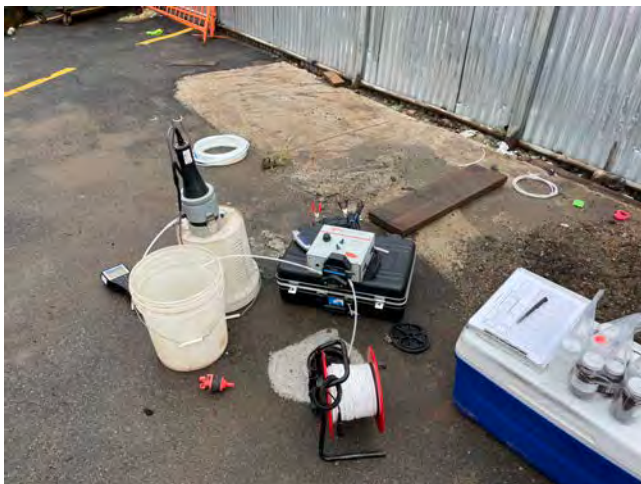
Photo 1: View of groundwater purging.
