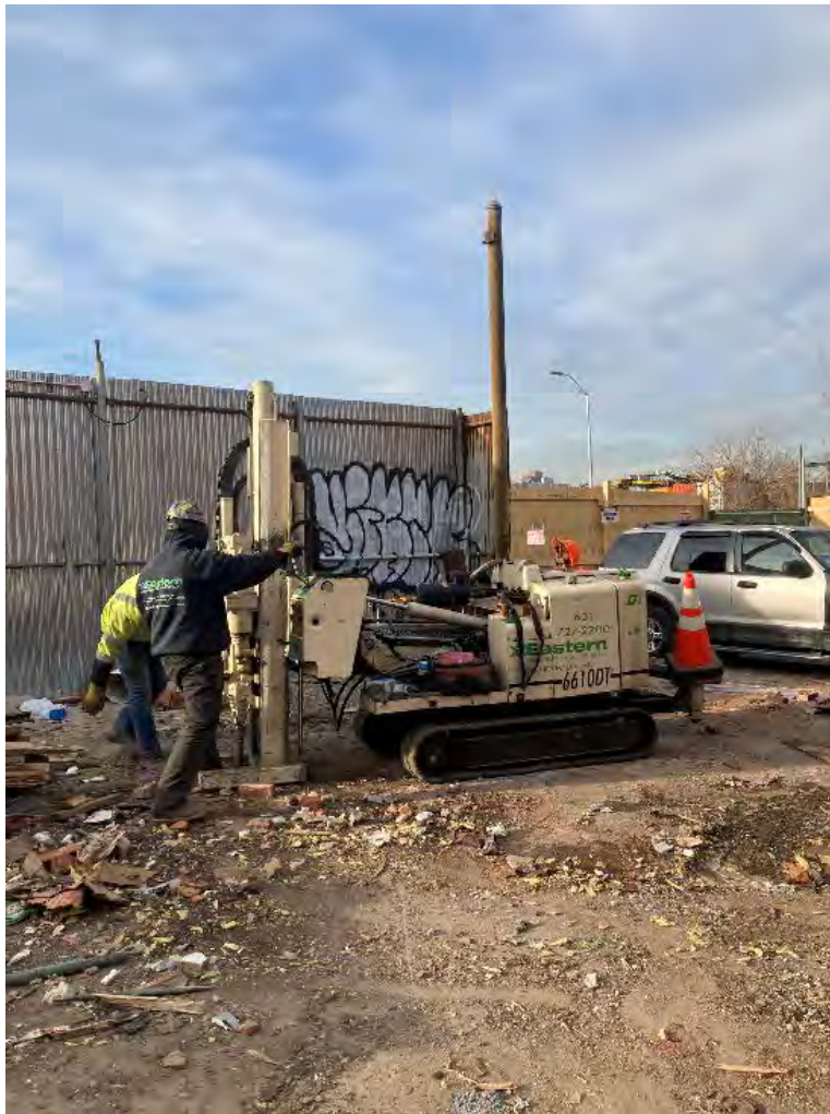
Photo 1: View of soil boring installation at location PDI-14.
