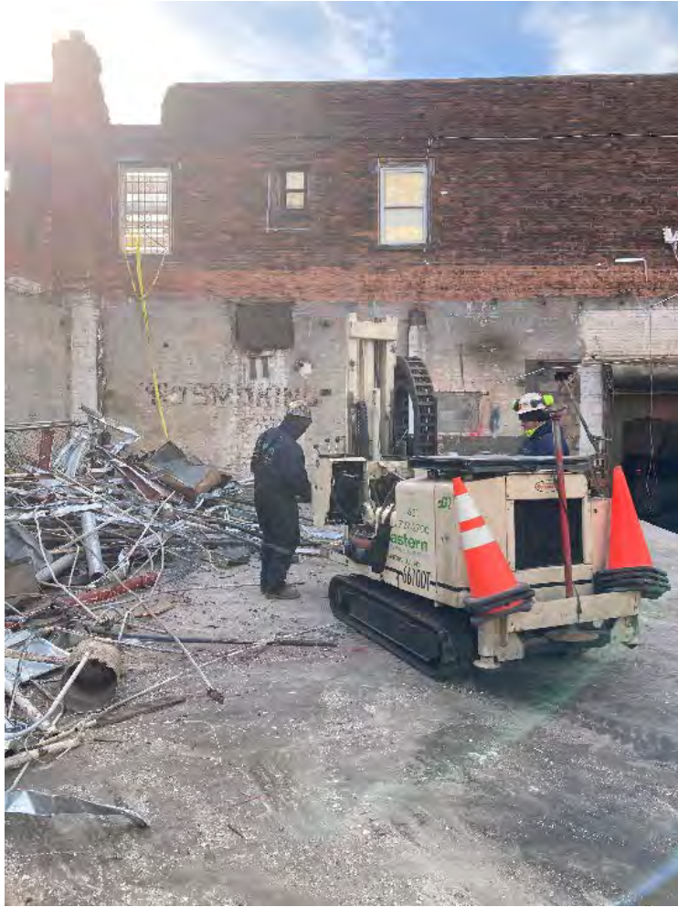
Photo 1: View of soil boring installation at location PDI-5.
