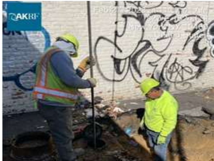
Photograph 2 - IPT checking the depth of the waste oil tank and for any residual oil.
