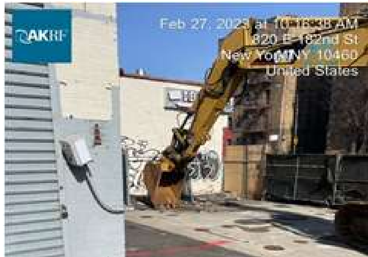
Photograph 1 - IPT removing concrete over the tank vault to gain access to the tanks.
