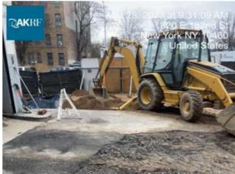
Photograph 1 - IPT backfilling open excavation with virgin fill material.
