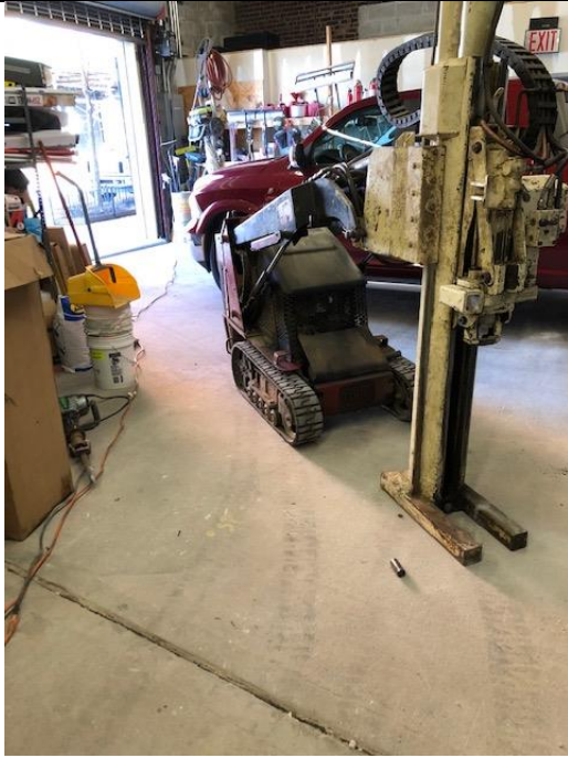
Installation of soil boring W11
