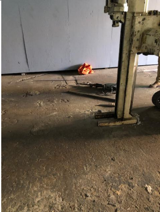
Installation of soil boring W1
