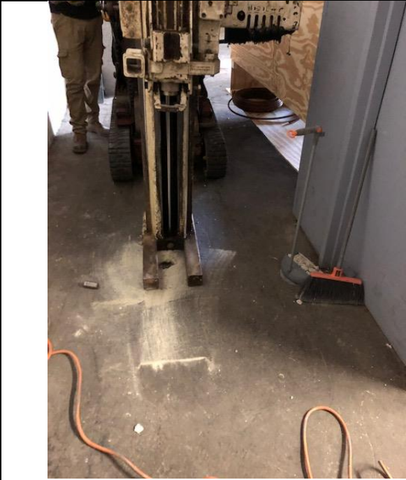
Installation of soil boring W8
