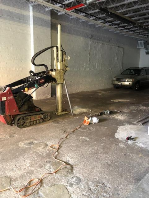
Installation of soil boring W2
