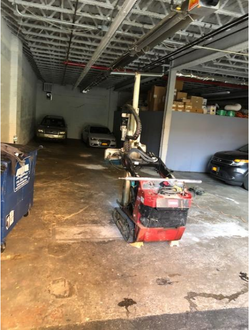
Installation of soil boring W3
