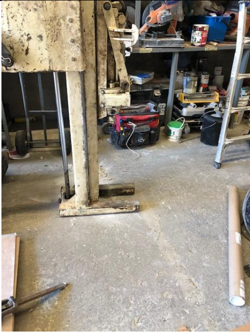
Installation of soil boring W14
