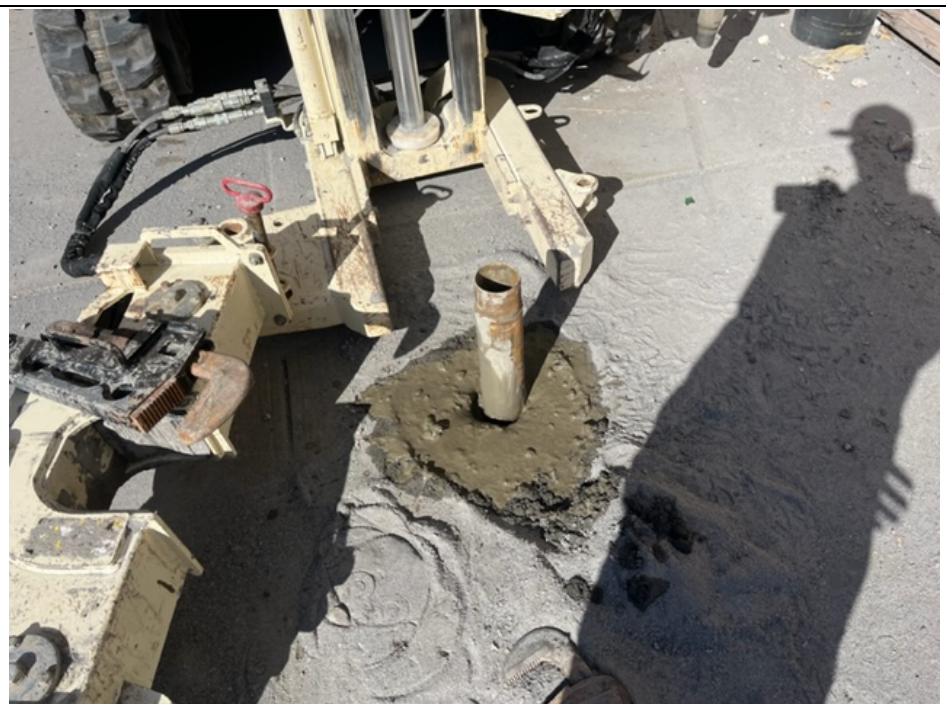
Photo 5: View of steel casing at MW-5
