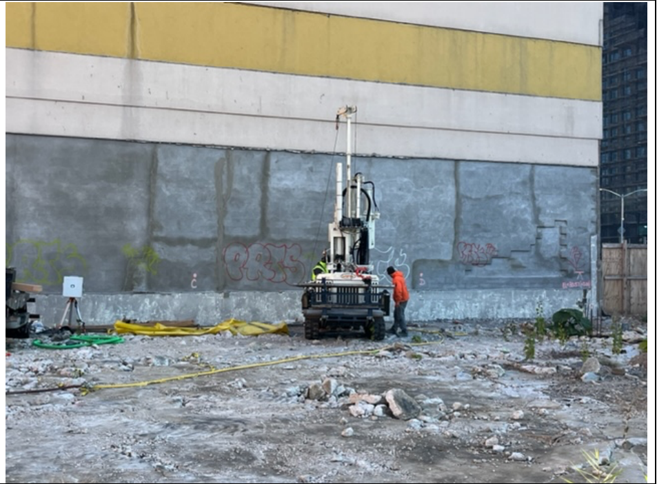
Photo 1: Coastal Environmental installing steel casing at MW-4 and view of downwind CAMP station
