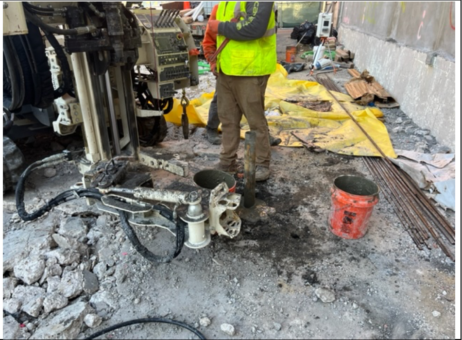
Photo 3: View of setting steel casing at MW-4
