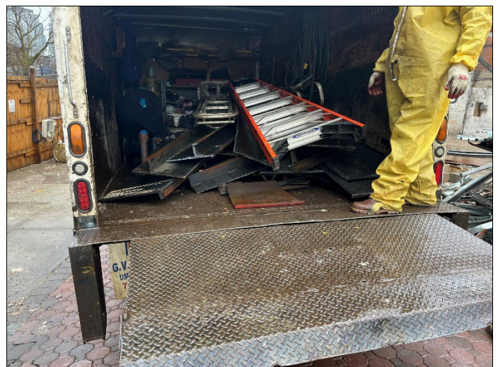
30. View of disassembled ASTs in truck for proper disposal
