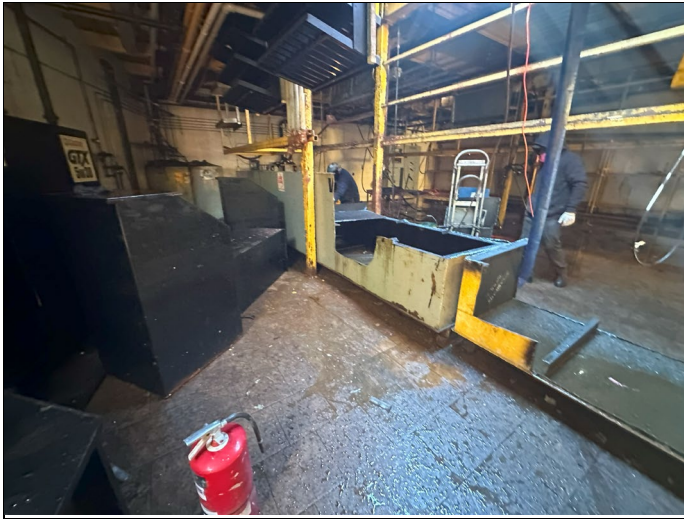
25. View of AST removal activities
