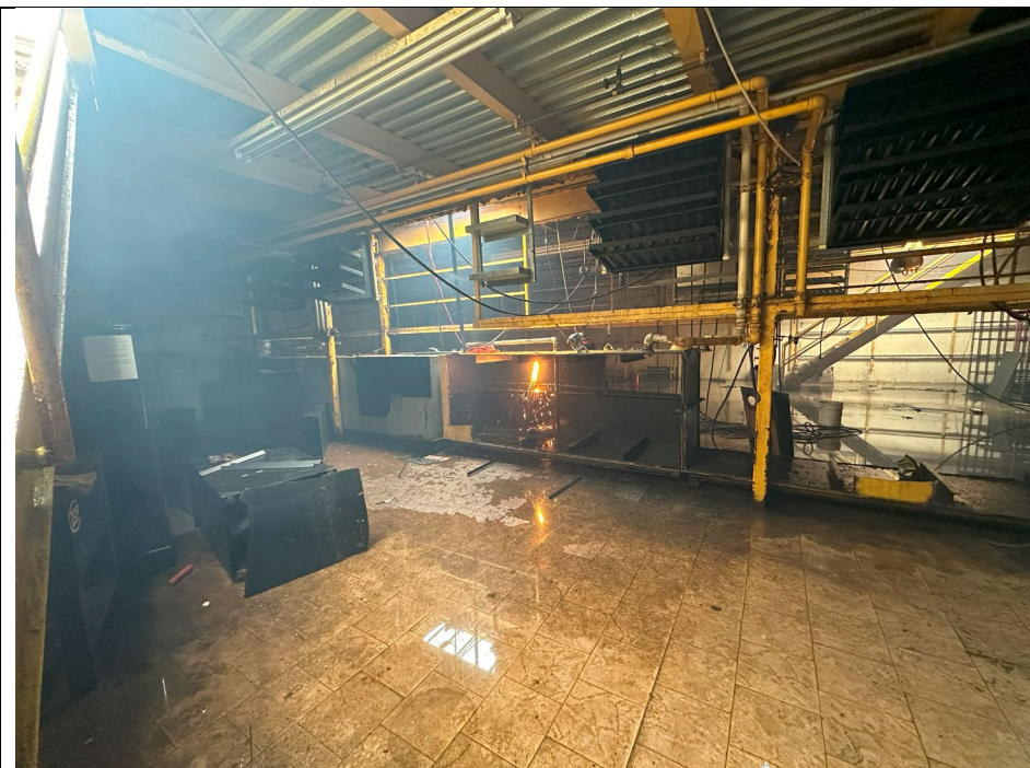
Photo 3: View of disassembly of AST carcass by ABC tanks.
