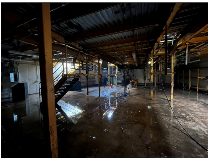
29. View of cellar after removal of ASTs
