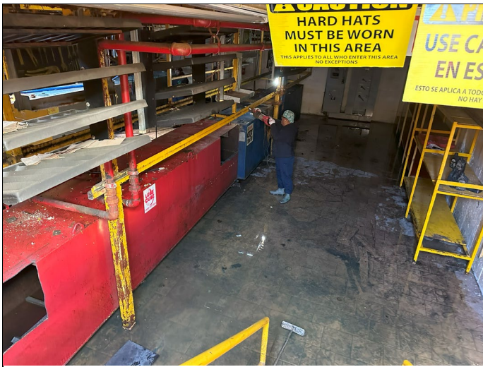
9. View of AST removal activities
