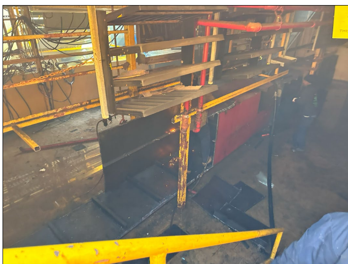
15. View of AST removal activities
