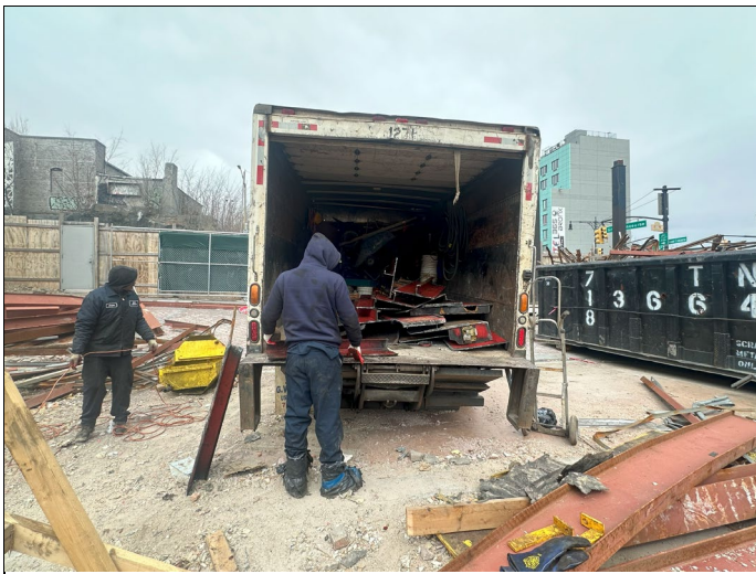
21. View of dissembled ASTs in truck for proper disposal
