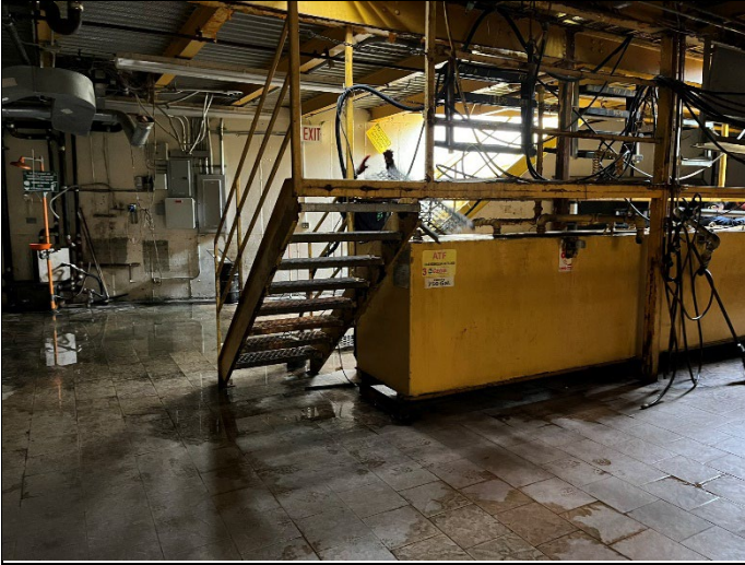
1. View of cellar prior to start of AST removal activities
