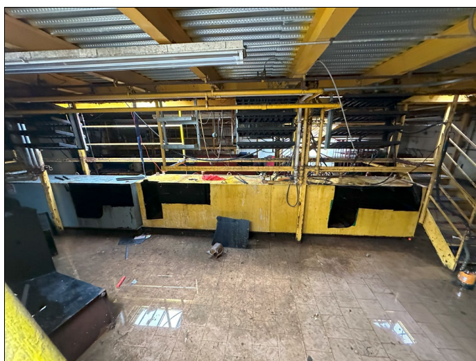
18. View of exposed ASTs
