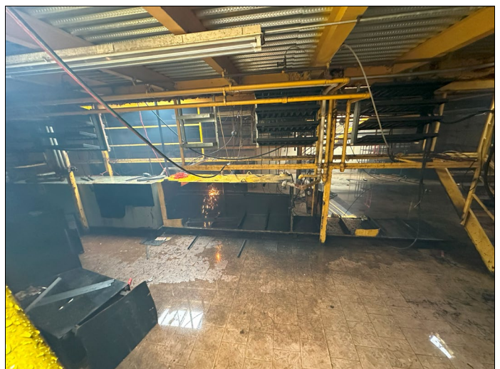
24. View of AST removal activities
