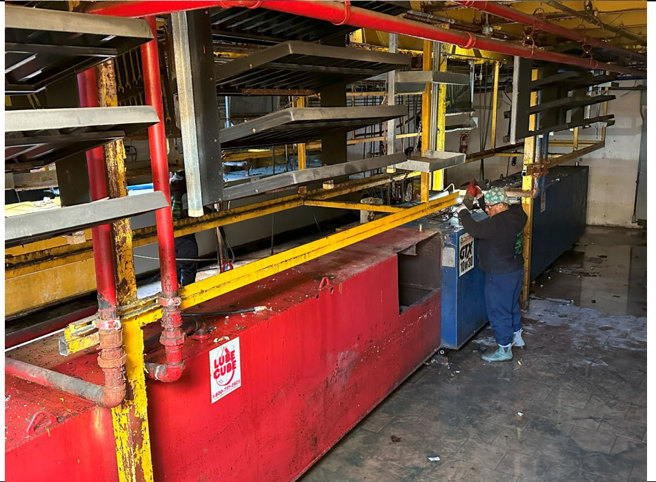
Photo 2: View of ABC tank cleaning cutting open ASTs.
