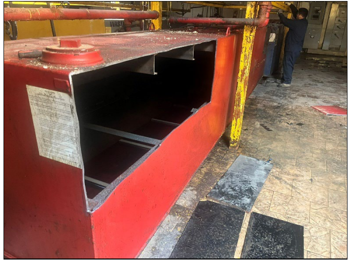
8. View of cut open AST
