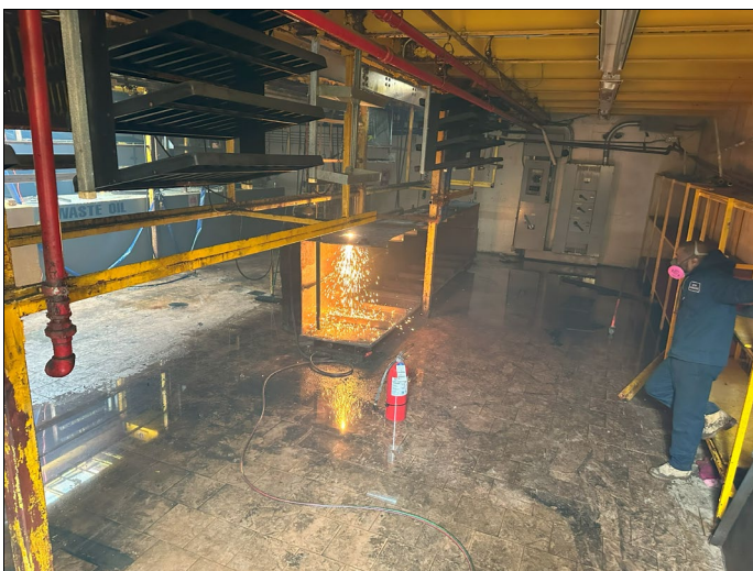
23. View of AST removal activities
