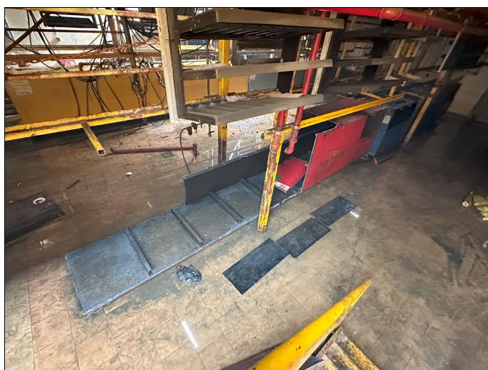
16. View of AST removal activities
