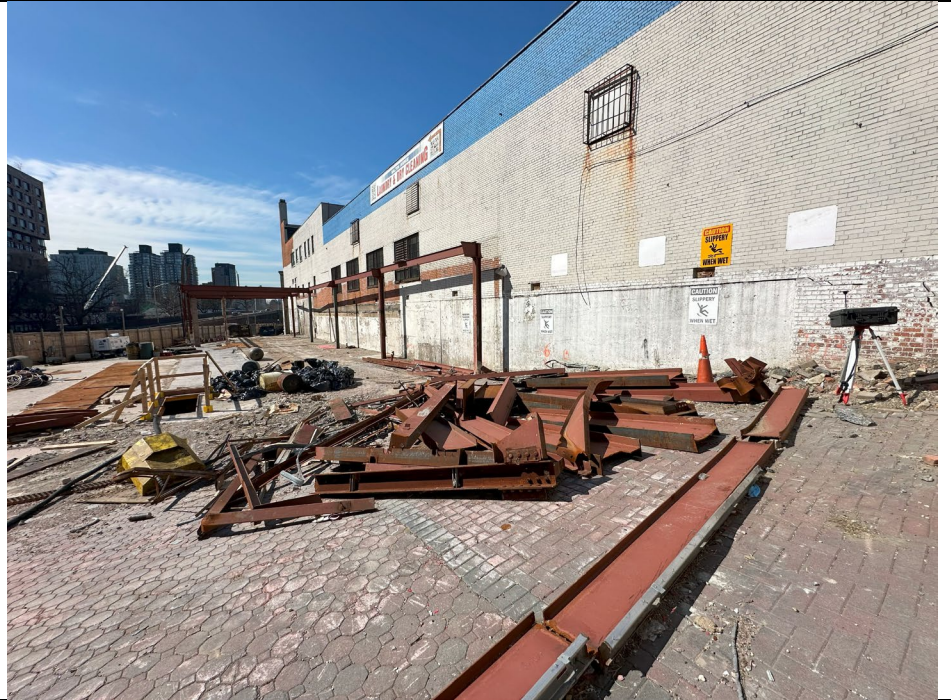
Photo 1: View of upwind CAMP station and cellar facing south.
