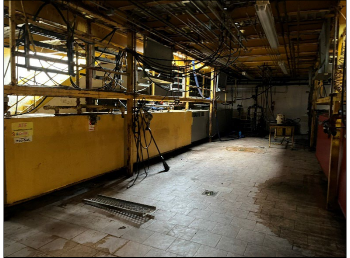
2. View of cellar prior to start of AST removal activities
