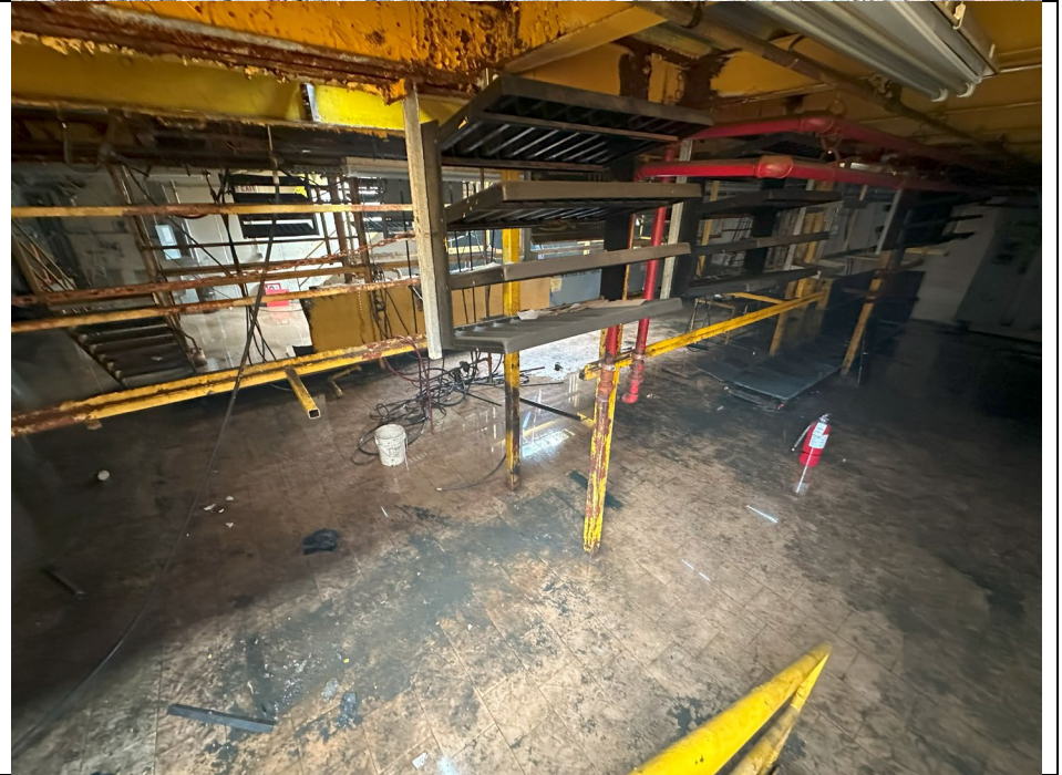
Photo 4: View of cellar after AST carcass was removed.
