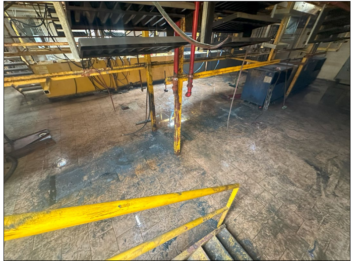
20. View of removed ASTs
