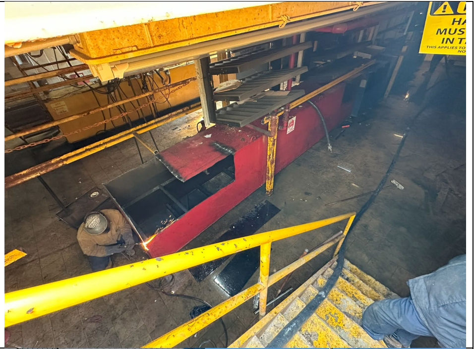
Photo 3: View of welder disassembling AST carcass.
