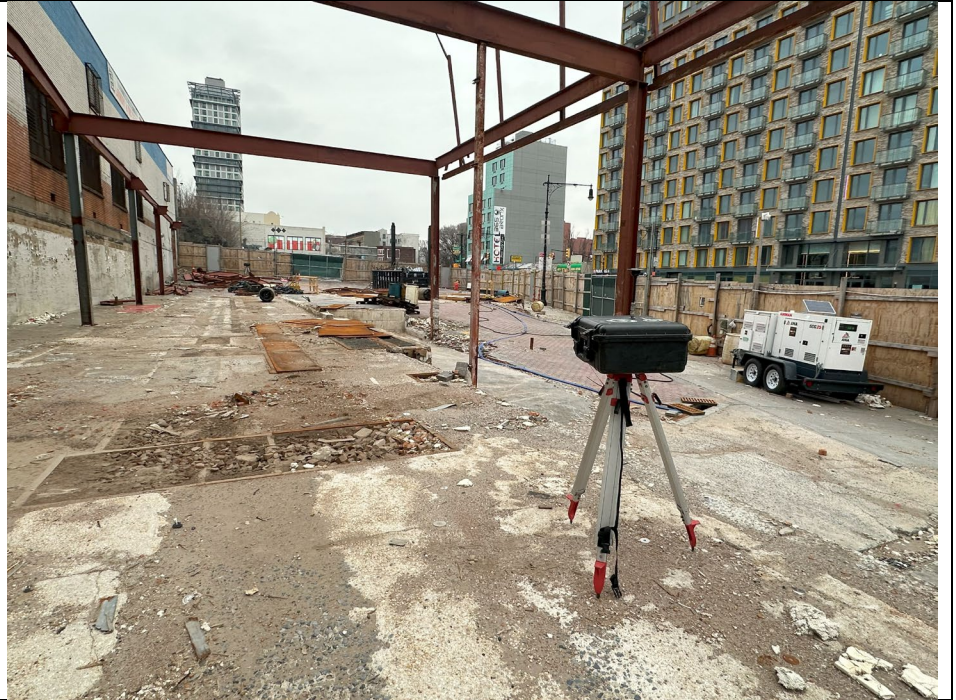
Photo 1: View of downwind CAMP station and cellar facing north.
