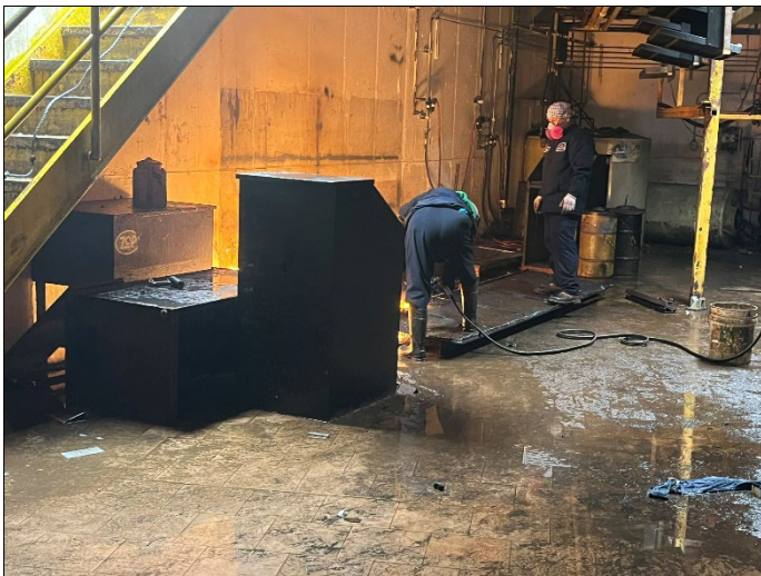
27. View of AST removal activities
