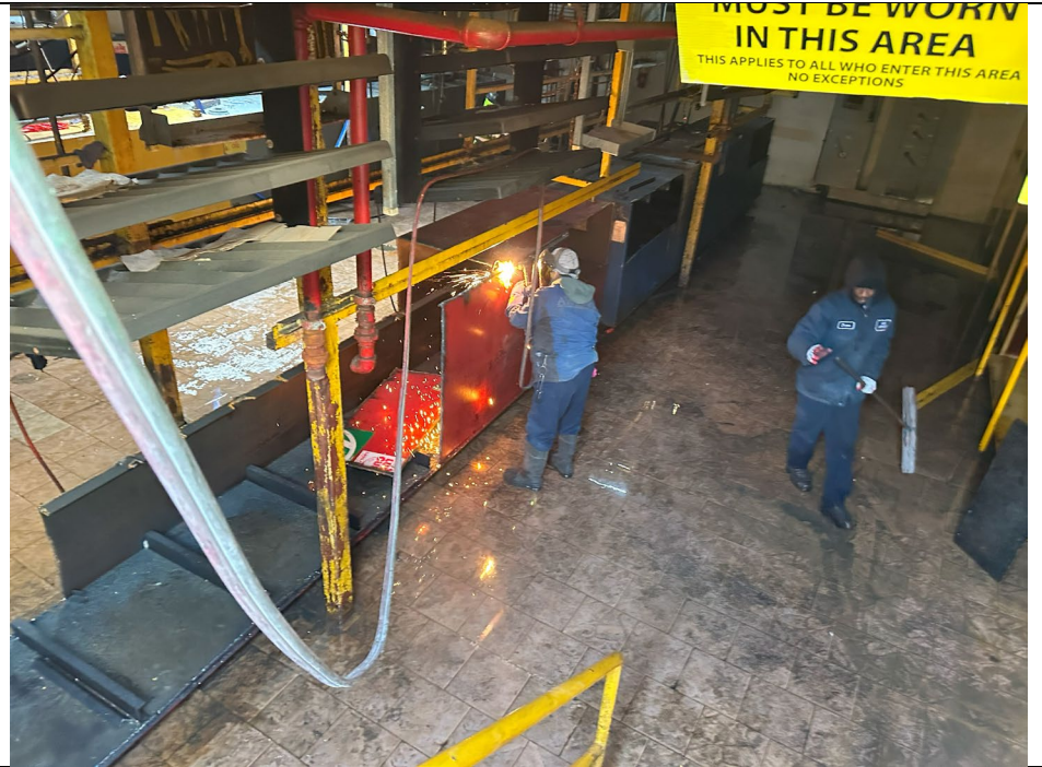
Photo 3: View of welder disassembling AST carcass.
