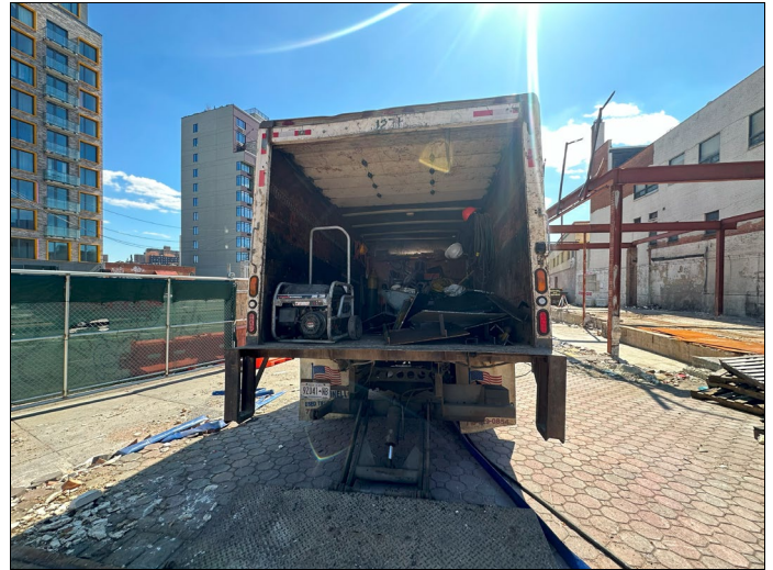
26. View of disassembled ASTs in truck for proper disposal
