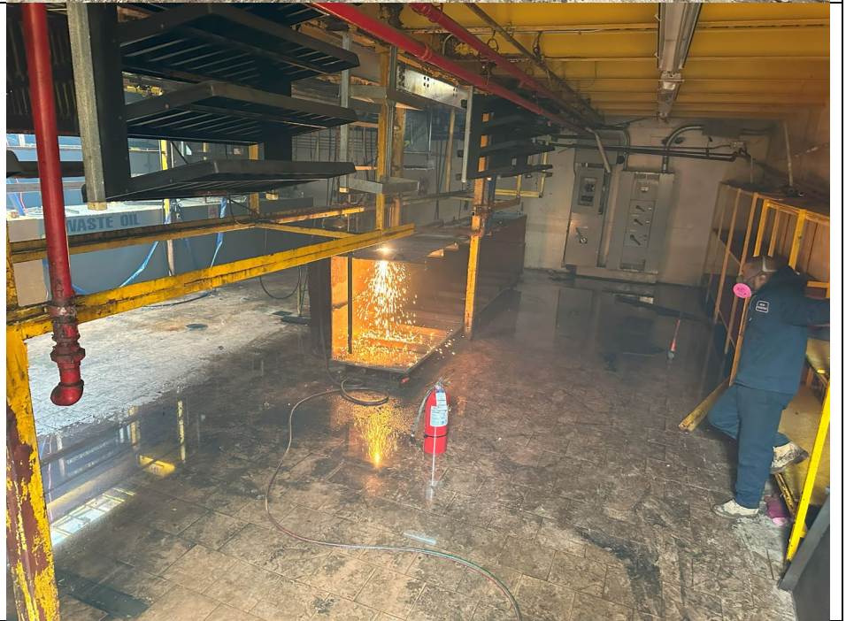
Photo 2: View of AST cut by welding, disassembled, and removed by ABC.
