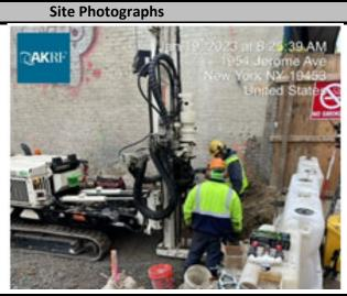
Photograph 2 - Isotec added Modified Fentons Reagent to the groundwater while JEL mixes the soil, view facing east.
