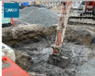
Photograph 3 - JEL backfilling the excavation with 3/4"stone following Isotec activities, view facing east.
