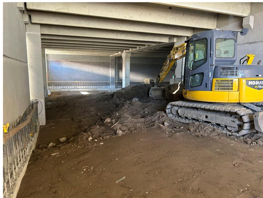
**Photo 4:** Soil was graded next to retaining walls in grids B1/B2.
