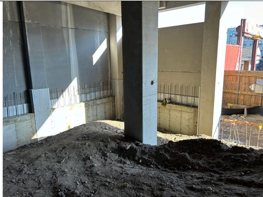
**Photo 2:** Removing forms from concrete retaining walls in B1.
