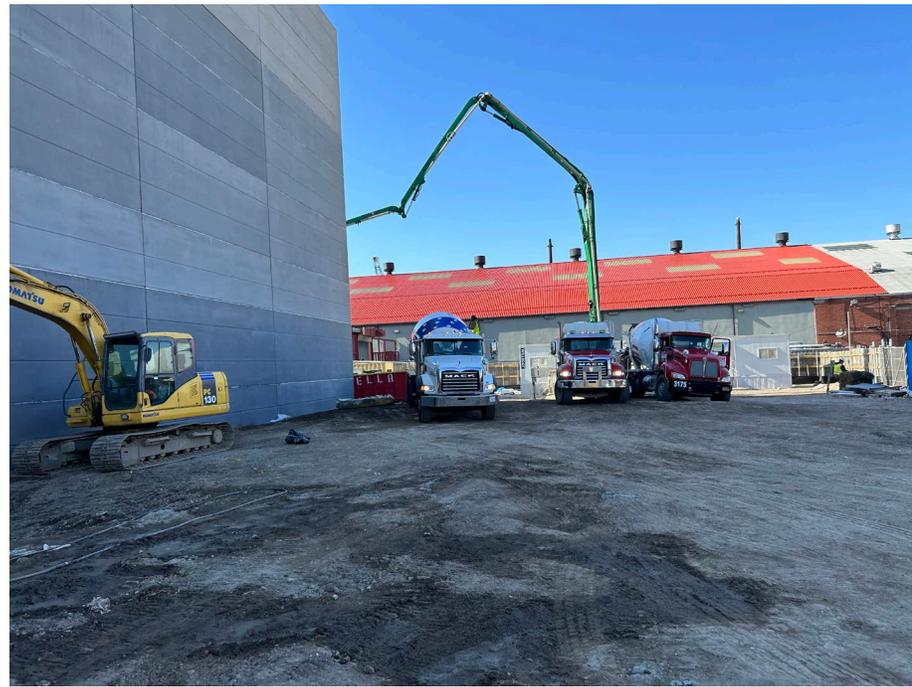
**Photo 1:** View of laydown area to the west of the building being use for 2<sup>nd</sup> floor concrete pour.
