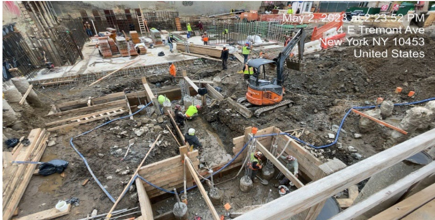
Photograph 2 - Trench excavated in grid WC-04. View facing Northeast.
