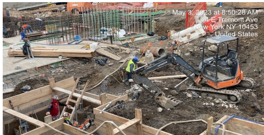
Photograph 3 - Unearthing of foundation piles with shovels in WC-04. View facing Southwest.
