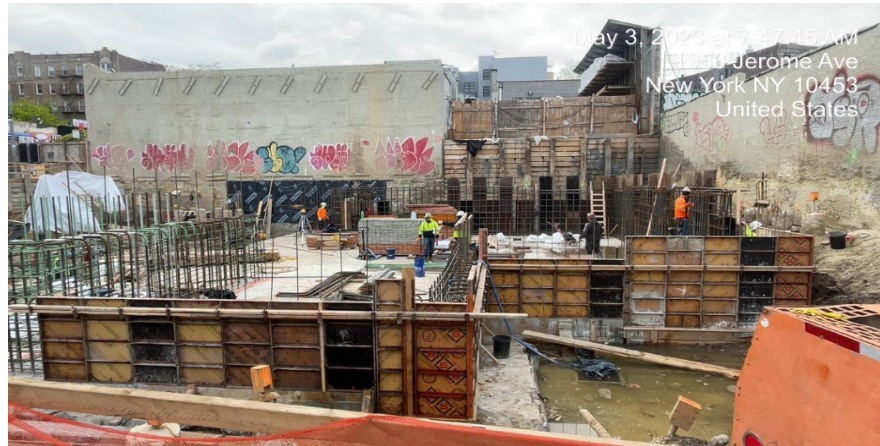
Photograph 1 - Rebar installation and foundation work in WC-03. View facing Southeast.
