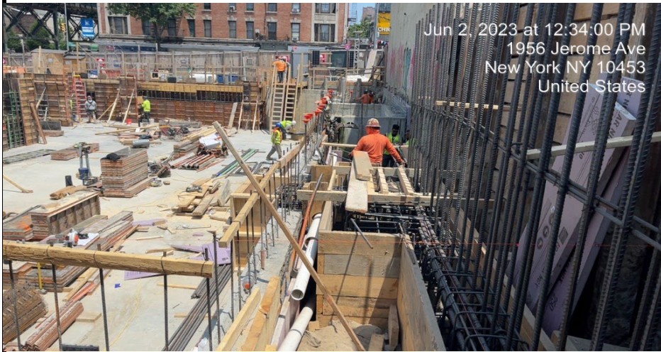
Photograph 2 - SSDS installation progress in WC-03 facing North.
