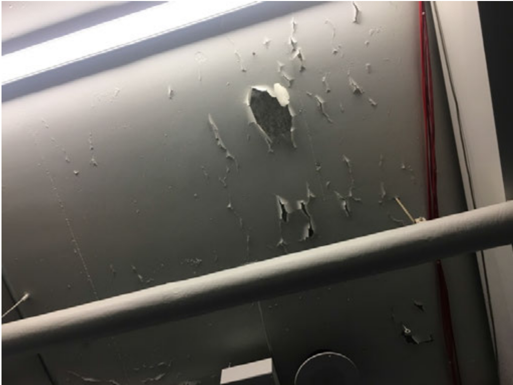
11. Chipped ceiling paint was observed in the basement self storage areas
