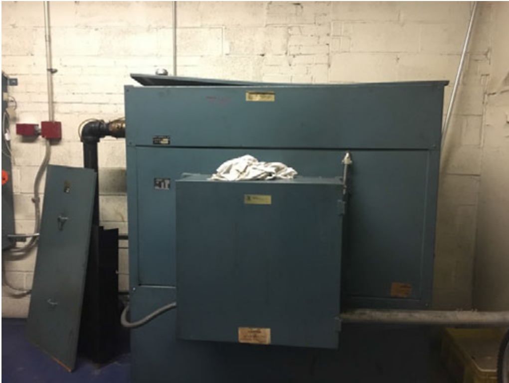
9. Representative elevator mechanical equipment (hydraulic)
