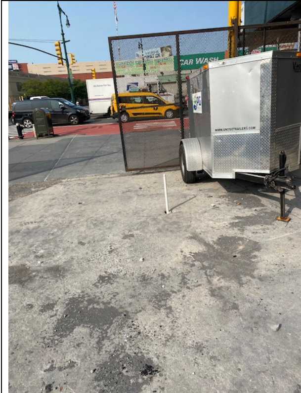
Monitoring Well Installation at Subject Property
