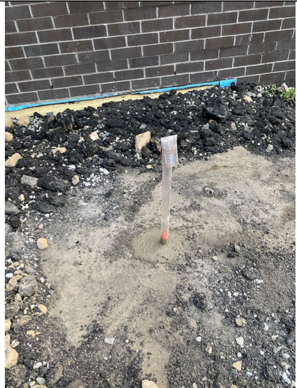
Monitoring Well Installation at Subject Property
