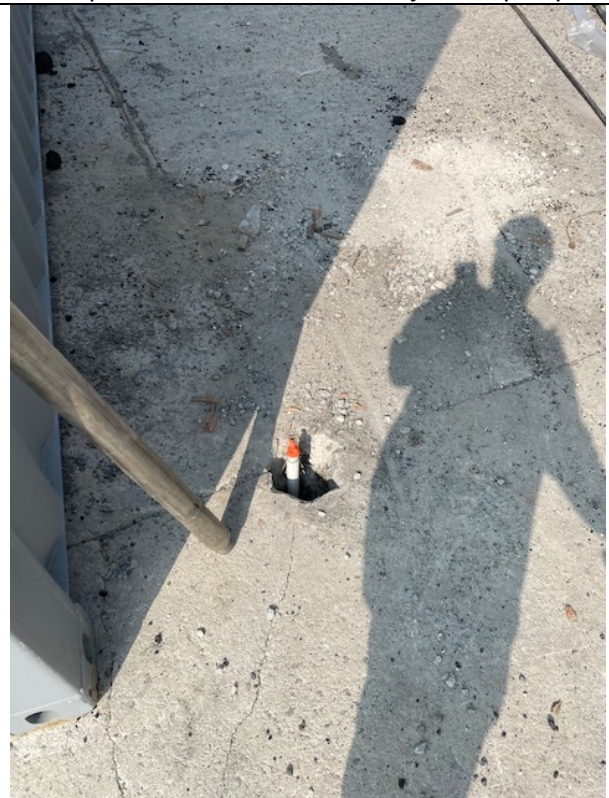
Monitoring Well Installation at Subject Property
