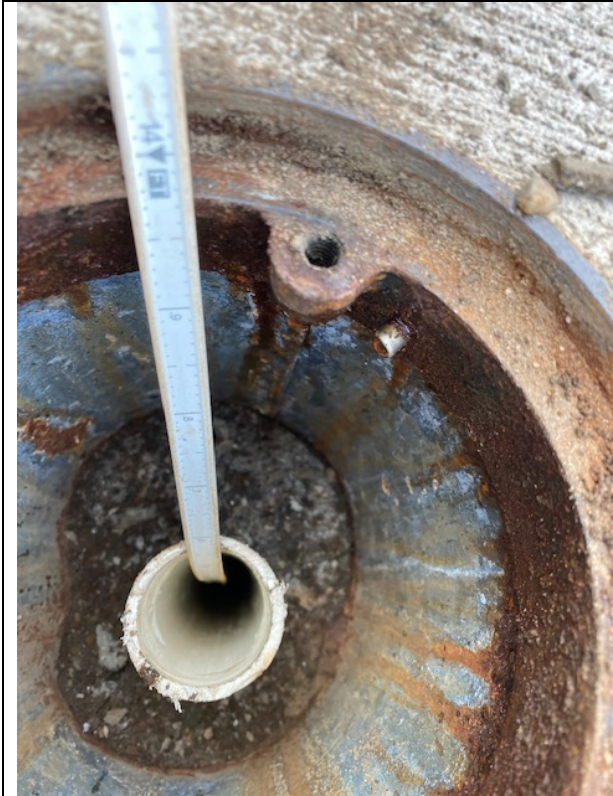
Depth to Water Measurement in Sidewalk Well
