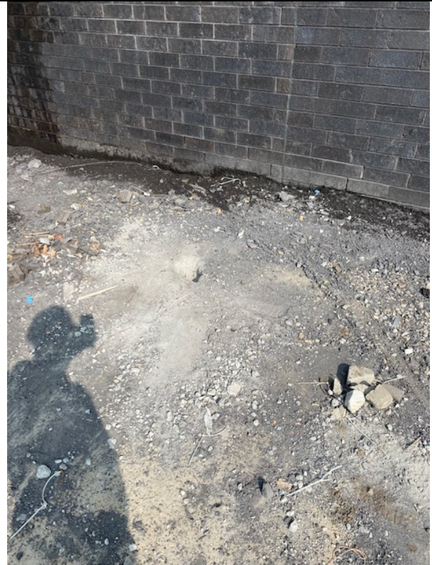
Monitoring Well Installation at Subject Property
