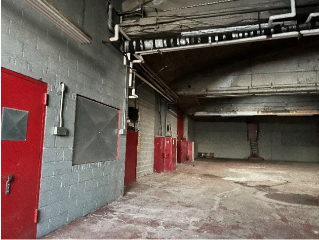
Photo 1: Site view indoor facing north
