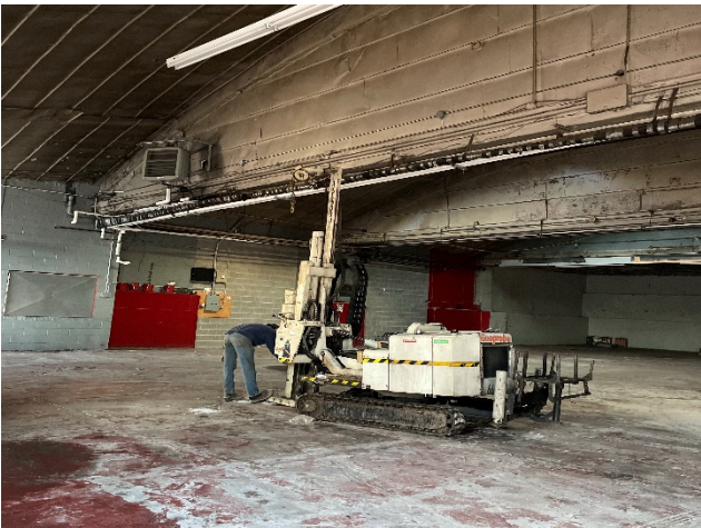
Photo 3: HA-01 soil boring drilling setup
