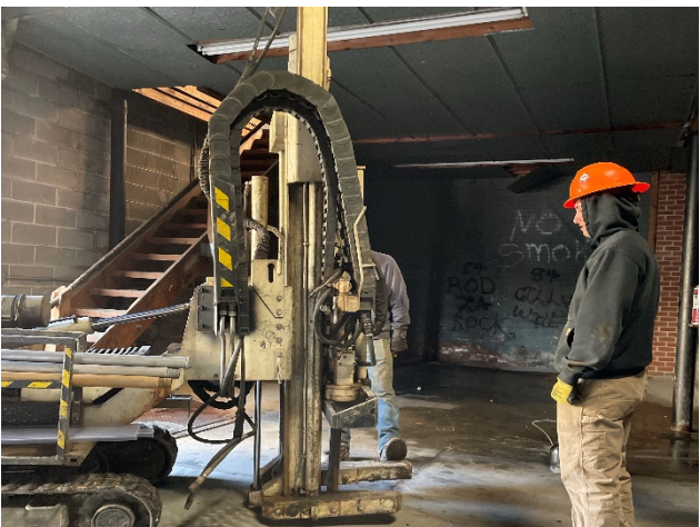
Photo 5: HA-05 soil boring drilling setup
