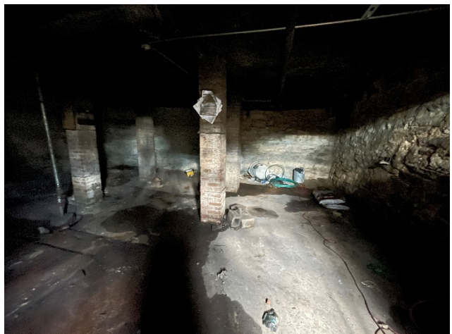
Photo 6: Partial cellar facing west
