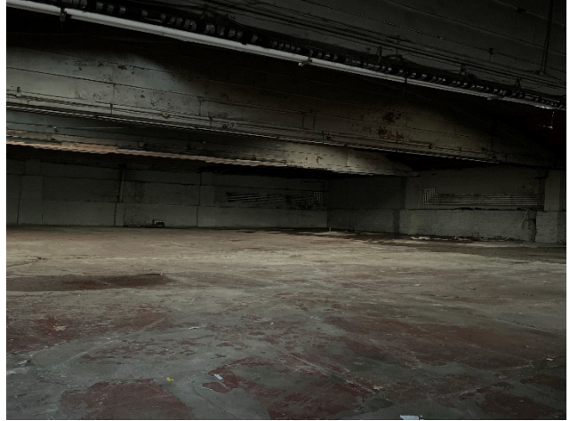
Photo 2: Site view indoor facing northeast
